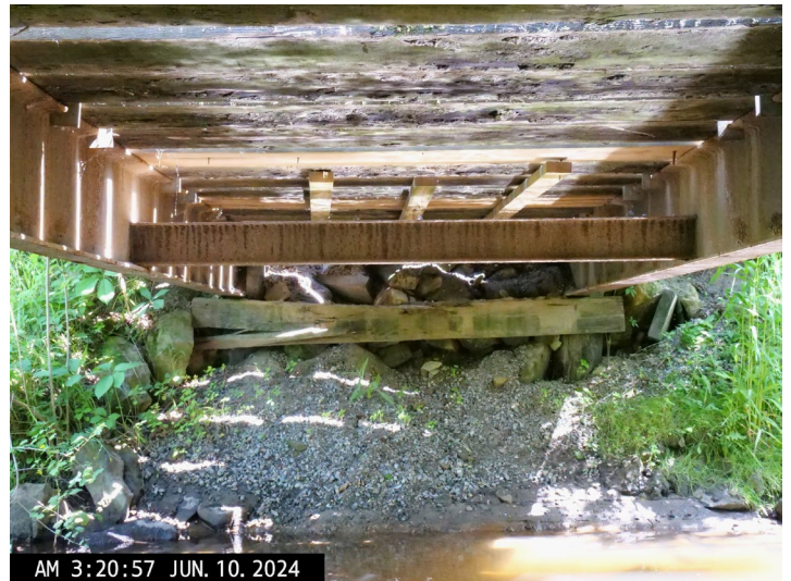
South Abutment Retaining Wall
