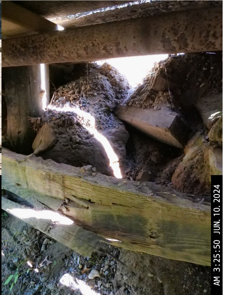
South Abutment & Retaining Wall
