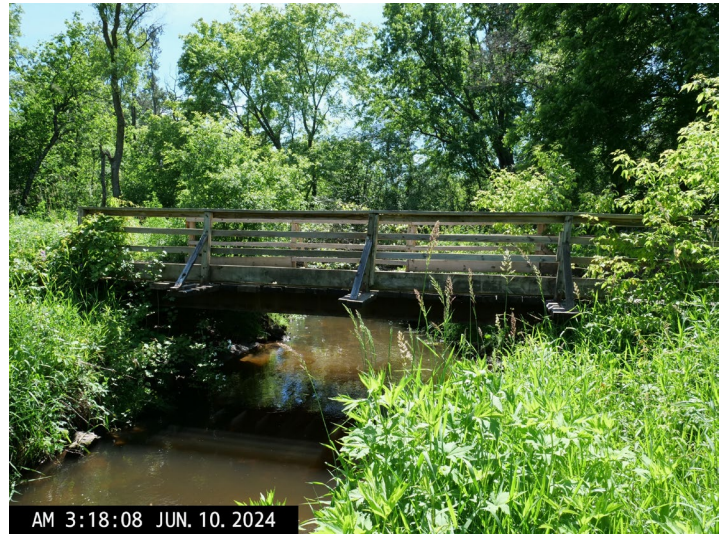
Bridge Profile Looking Downstream to West
