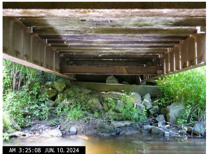
North Abutment & Retaining Wall
