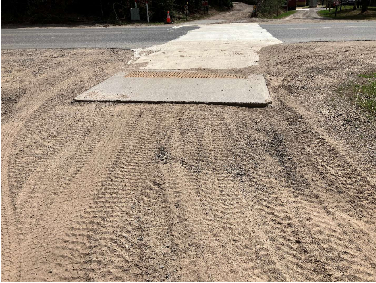
Vilas Co Trail 8 Rehab – Hwy 45 to Burnt Bridge
