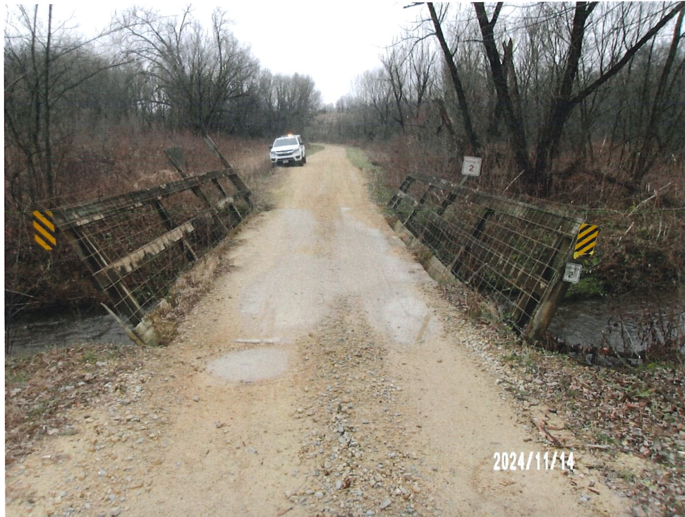
Figure 1 South Approach Looking North
