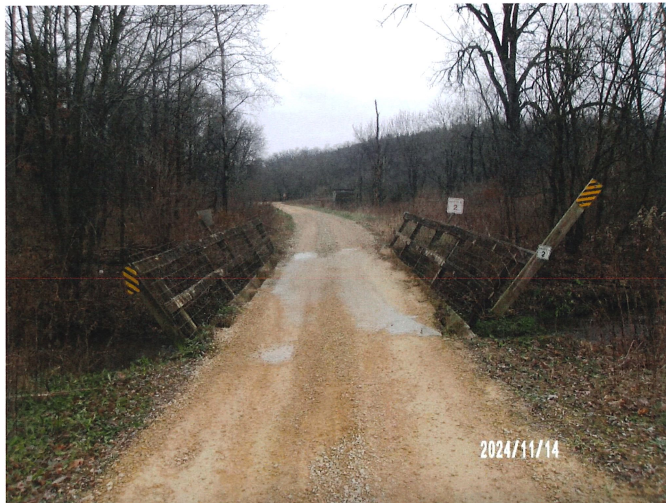
Figure 2: North Approach looking South
