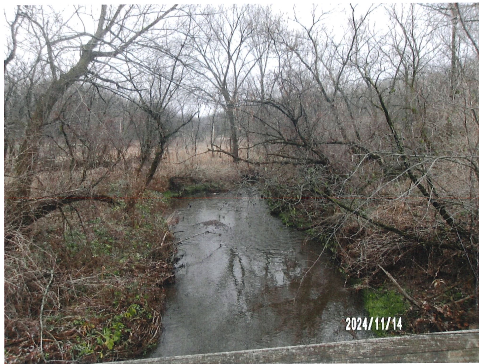
Figure 4: Looking Downstream from Top of Deck
