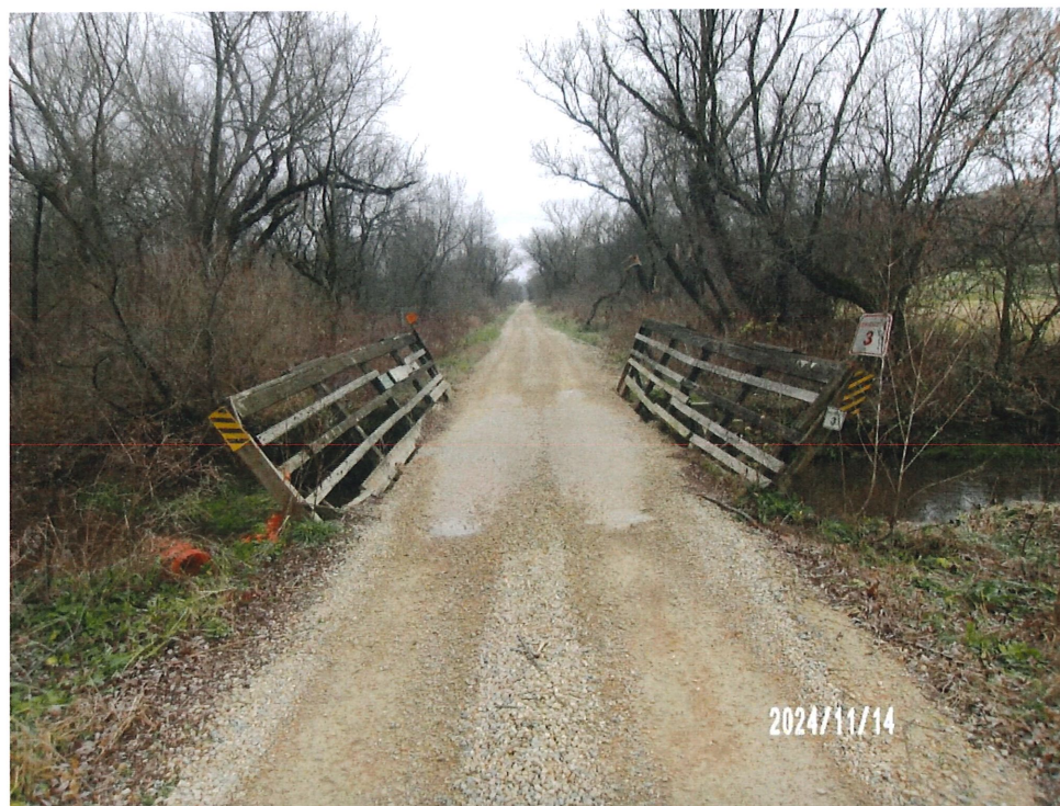
Figure 2: North Approach looking South
