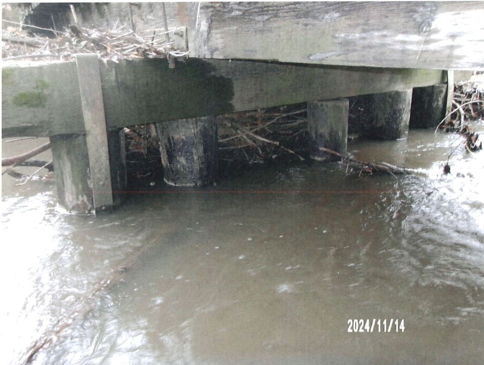
Figure 10: North Face of Pier
