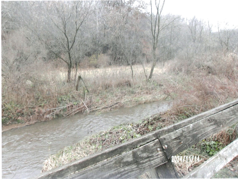
Figure 3: Looking Upstream from Top of Deck
