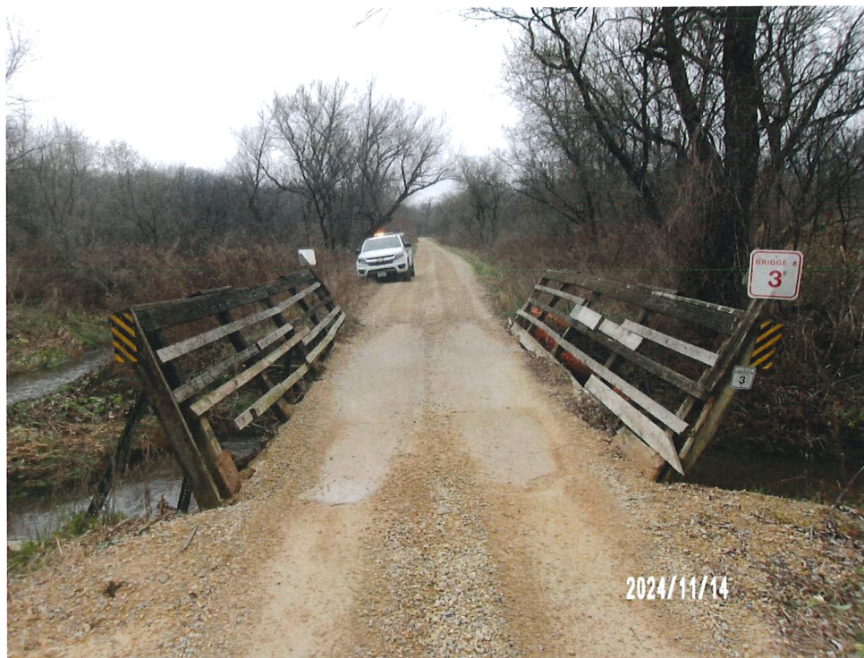
Figure 1 South Approach Looking North
