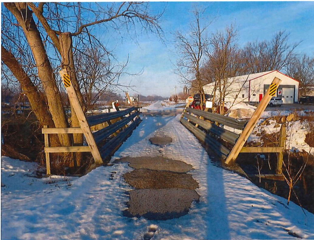
View of east approach, looking west.
