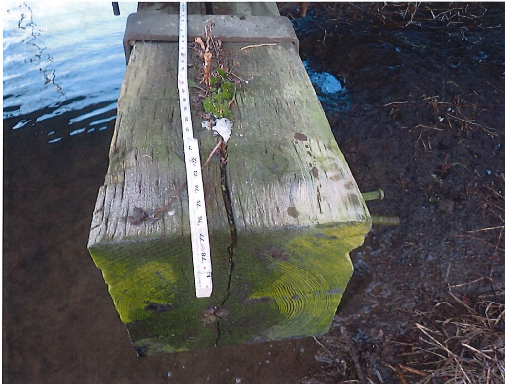
View of pier cap end decay, looking south.
