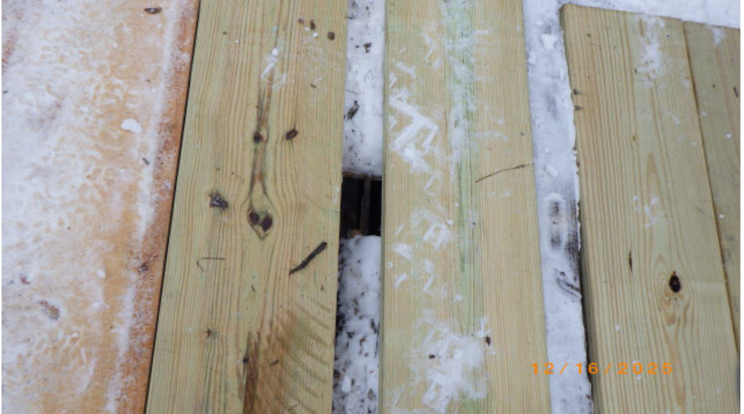
Deck holes patched on top with 2x running planks.
