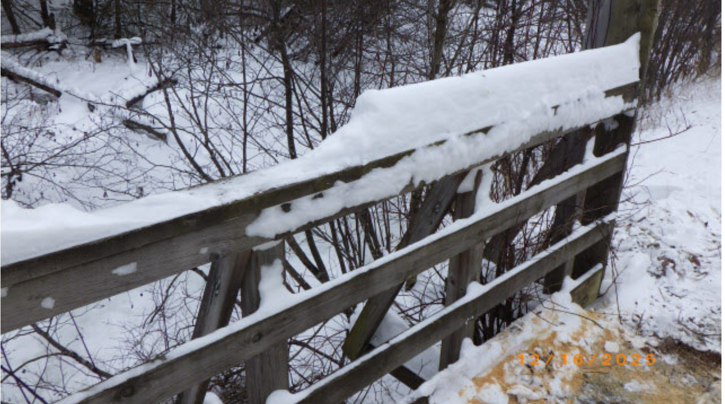
Brush around bridge ends
