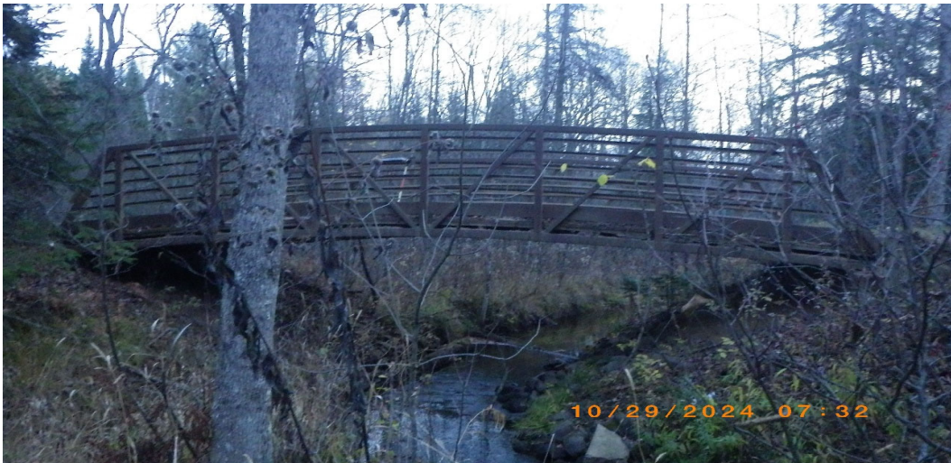
Looking Downstream - Elevation Profile
