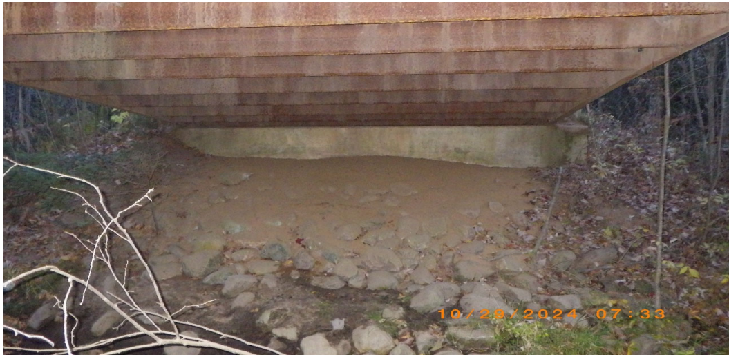
River Right Abutment
