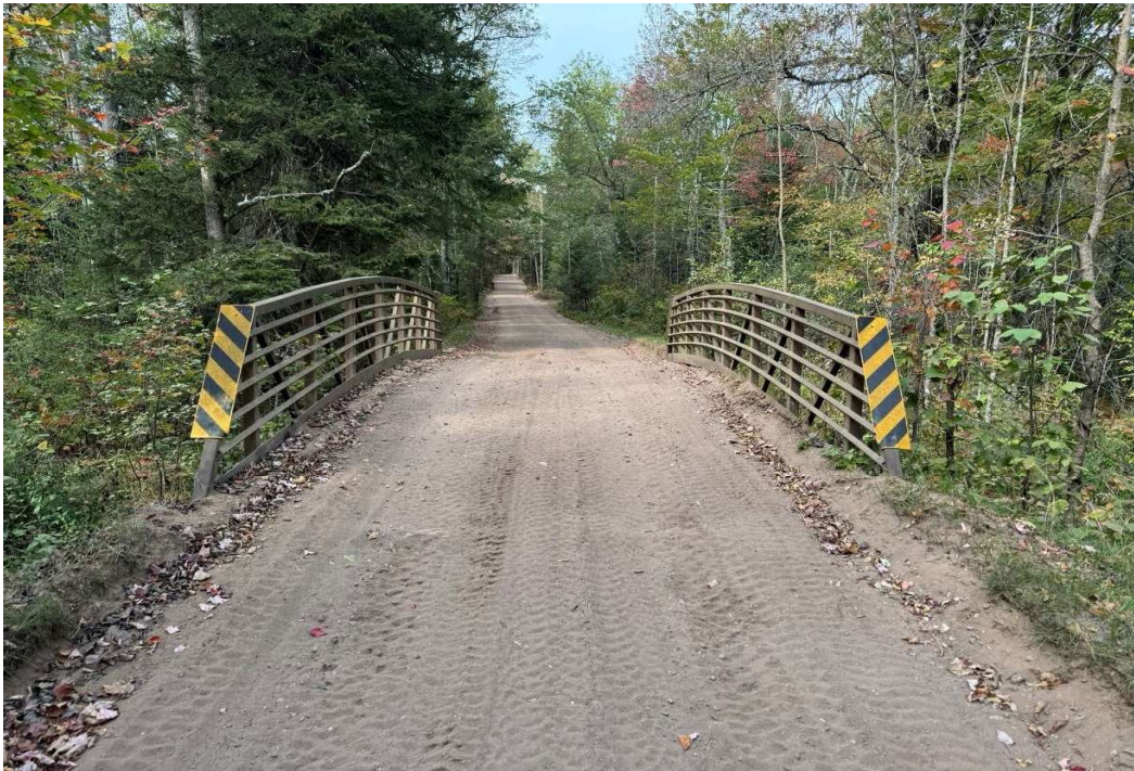
Closer view looking north
