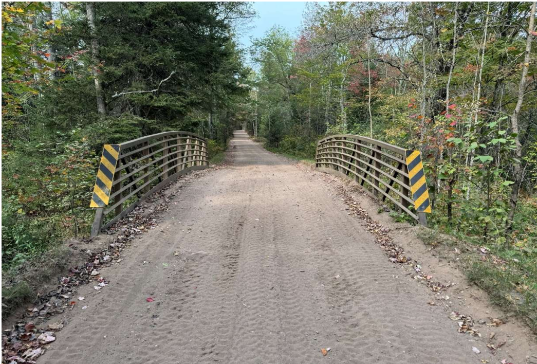
Closer view looking north
