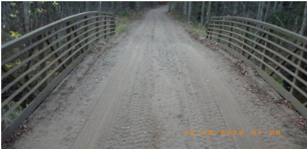
View of Deck and Rails
