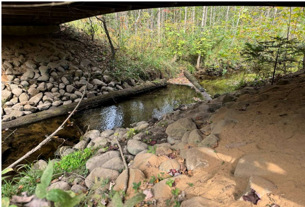
Channel under bridge
