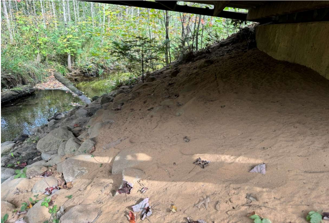
South riprap slope looking DS
