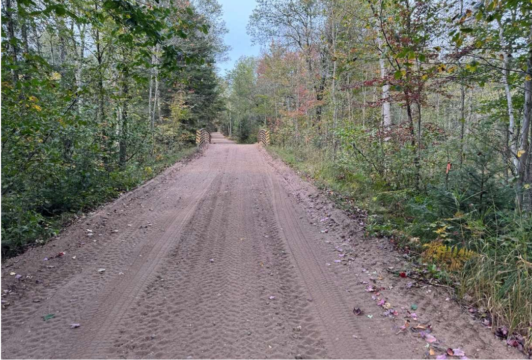
Hay Creek Bridge - looking north
