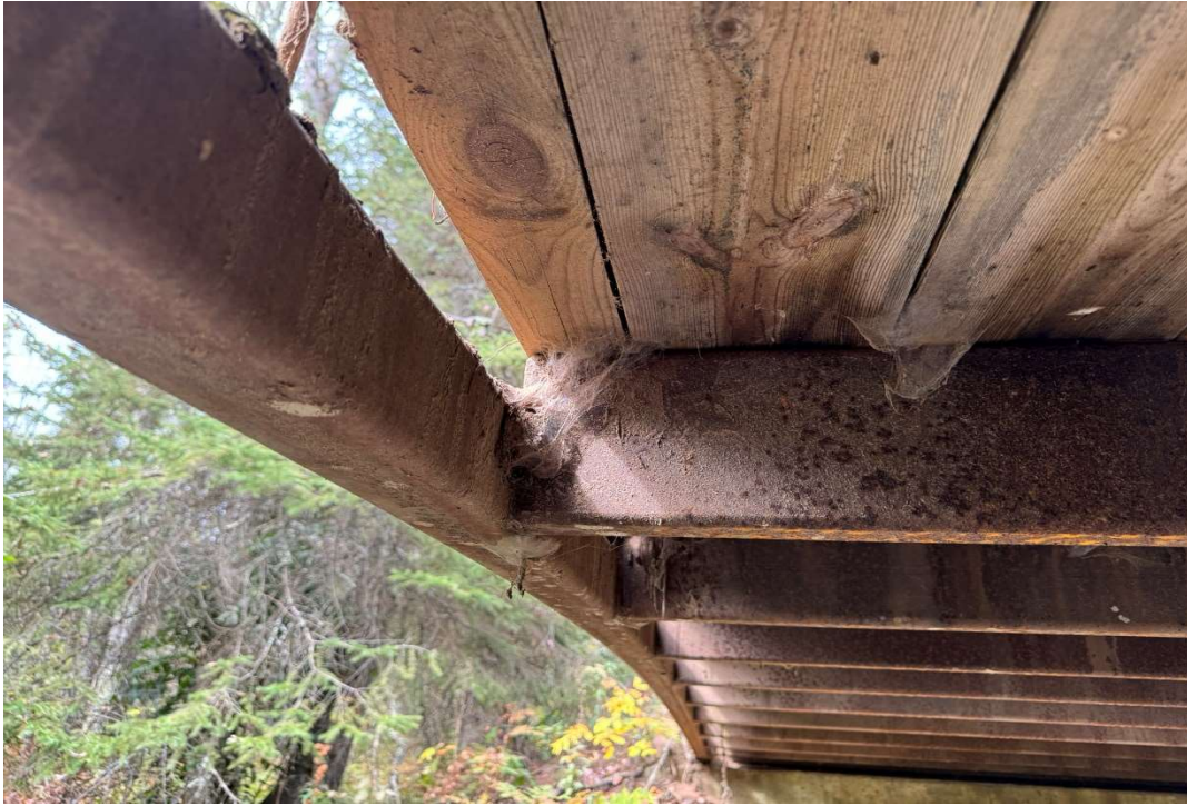
Typical floorbeam connection
