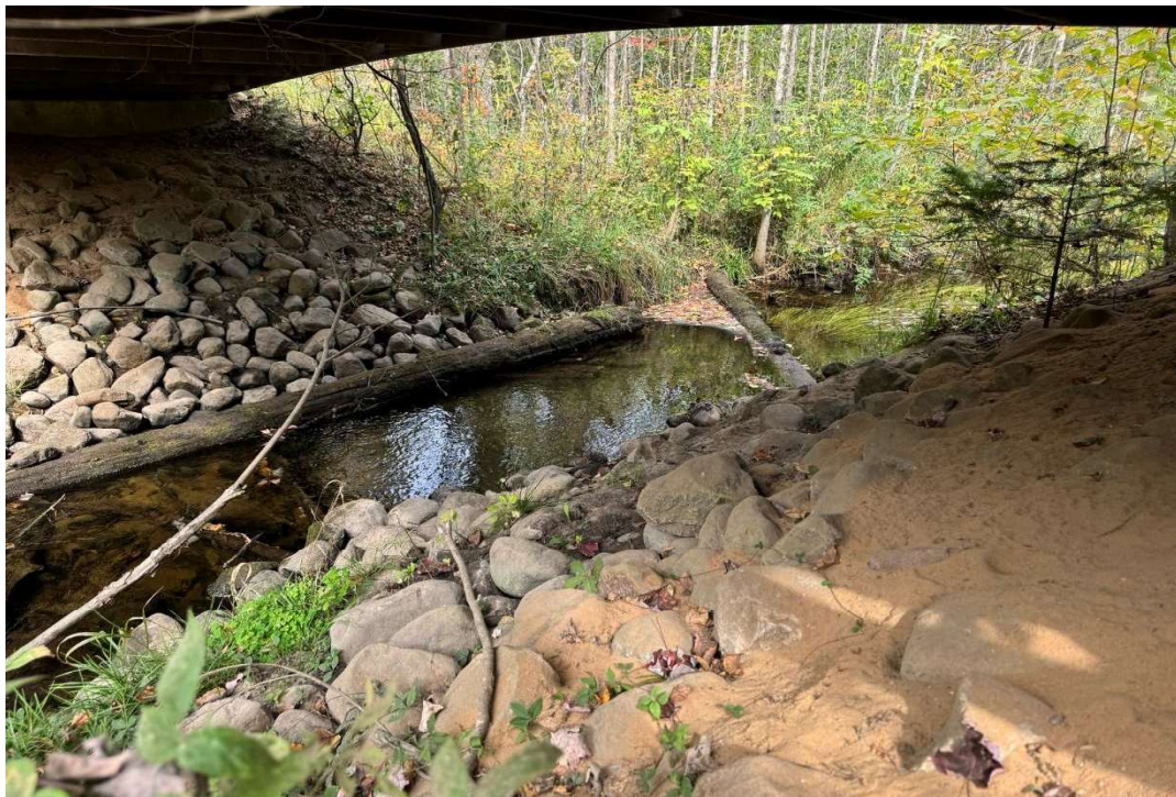
Channel under bridge
