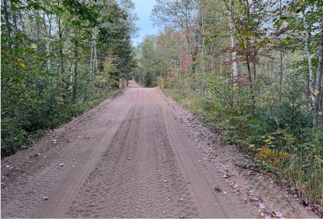
Hay Creek Bridge - looking north
