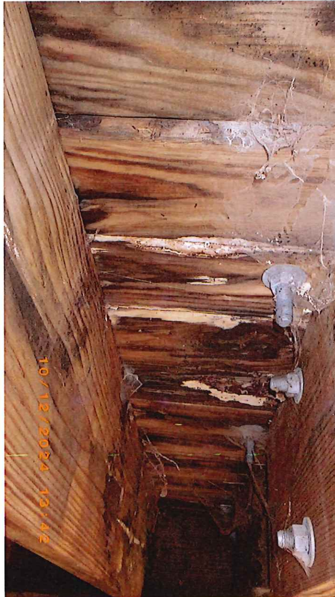
Rotten deck planks
