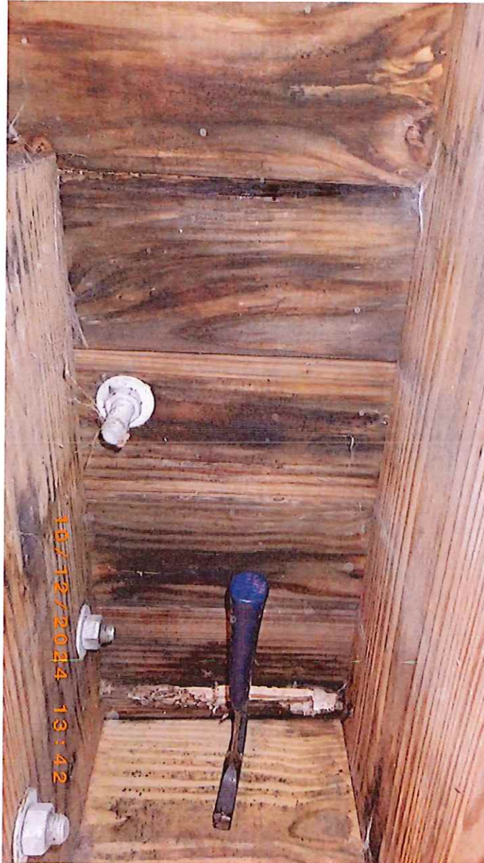
Rotten deck planks
