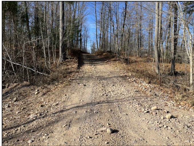
ATV Trail – Kozak Ln. to Cty Rd. 0 Pic. 1
