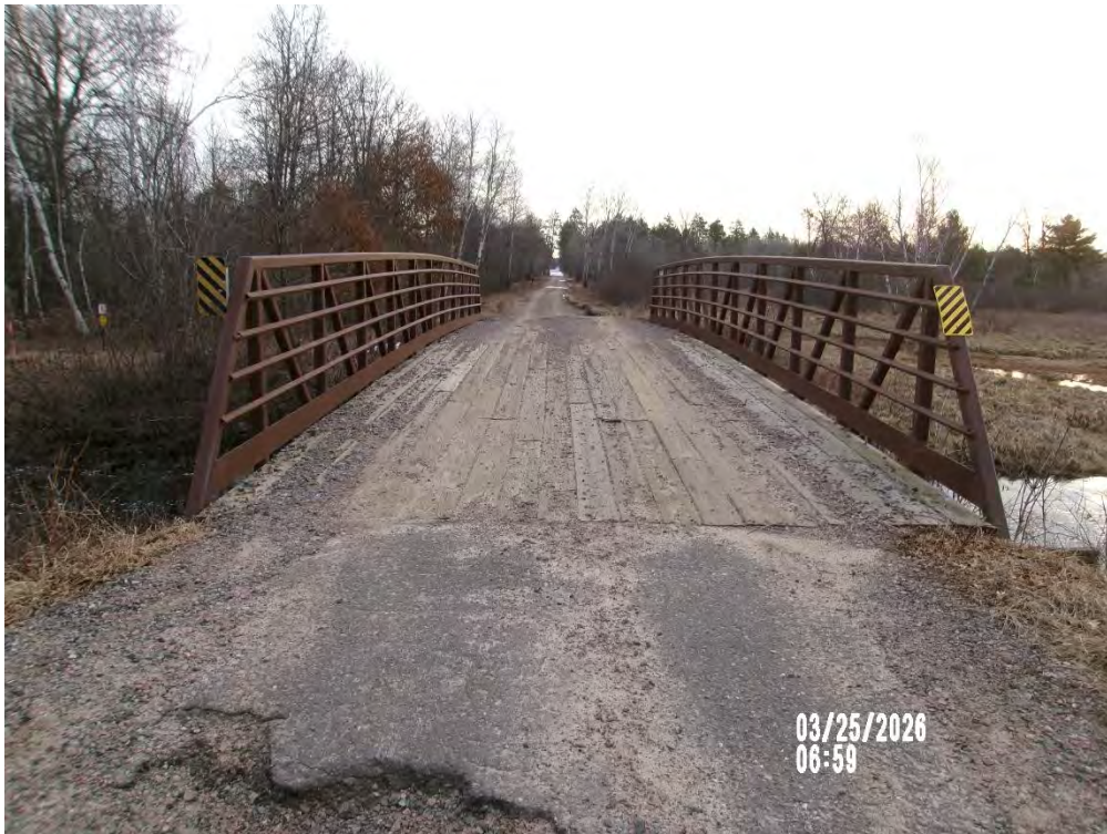
Figure 2: West Approach looking East
