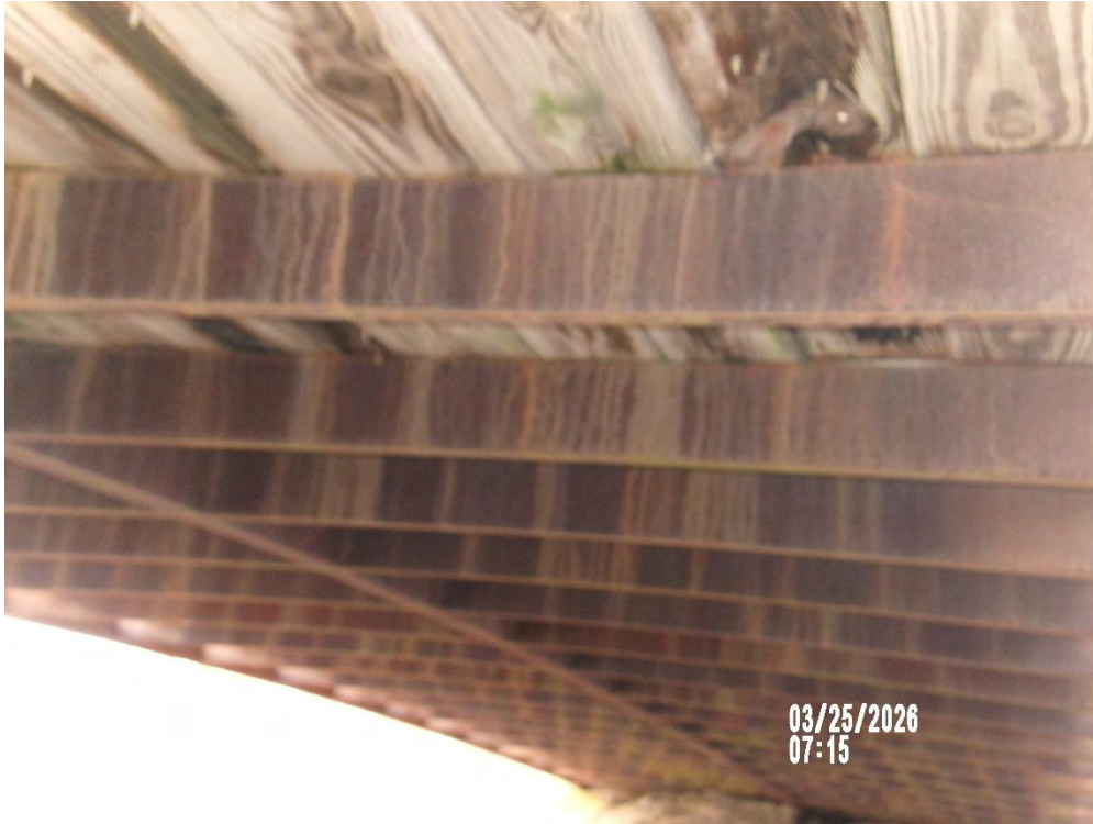
Figure 11: Typical floor beam condition
