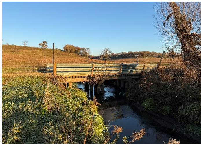
Photo 5 – Side View Looking West.
