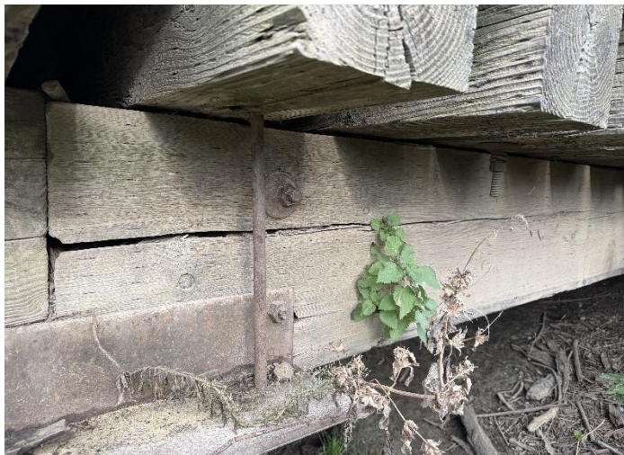
Photo 15 – East Beam-North Span Over North Pier.
