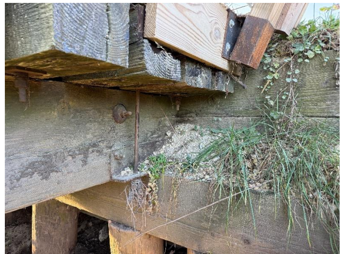
Photo 10 – West beam Over South Abutment.
