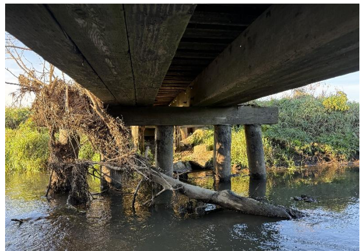
Photo 12 – South Pier Looking South.
