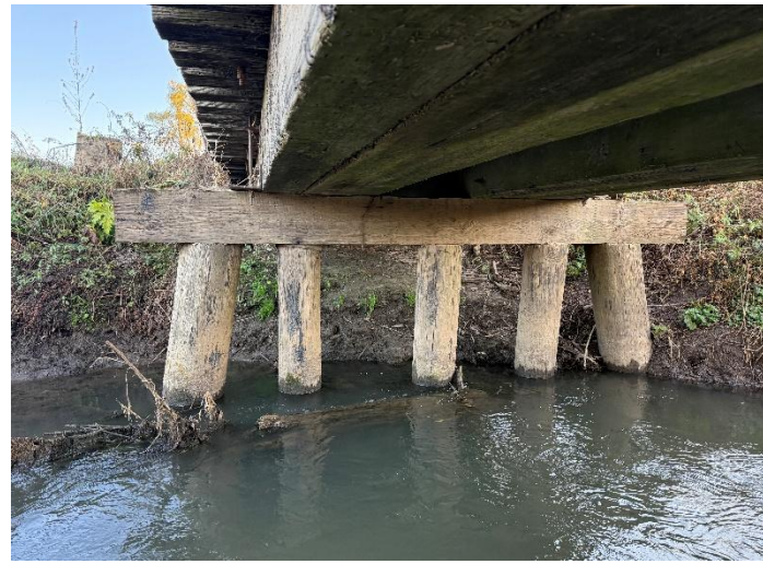
Photo 7 – North Pier Looking North.
