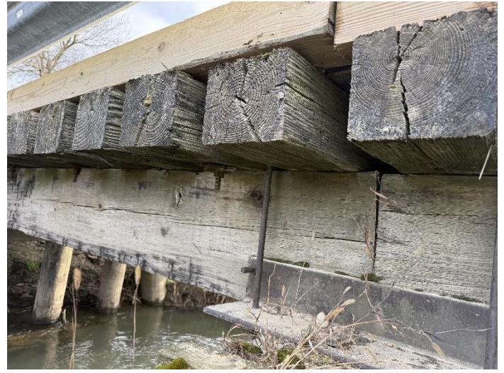
Photo 14 – West Beam/Edge of Deck-Center Span.
