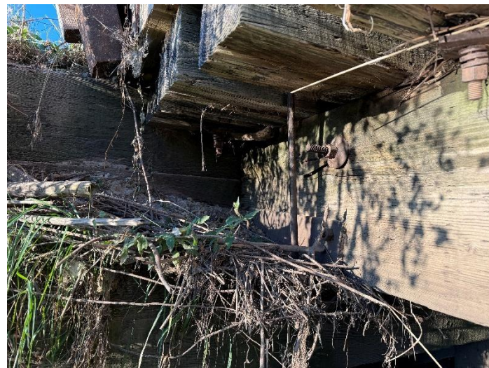
Photo 9 – East Beam Over South Abutment.
