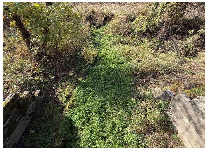
Photo 4 – Downstream Looking West.
