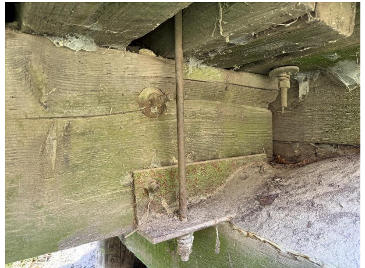
Photo 10 – East Beam Over North Abutment.
