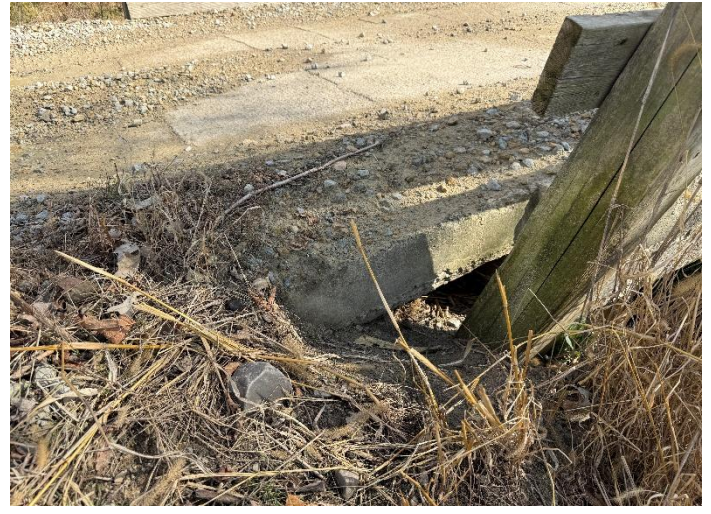
Photo 8 – West Corner of North Approach. Typical.
