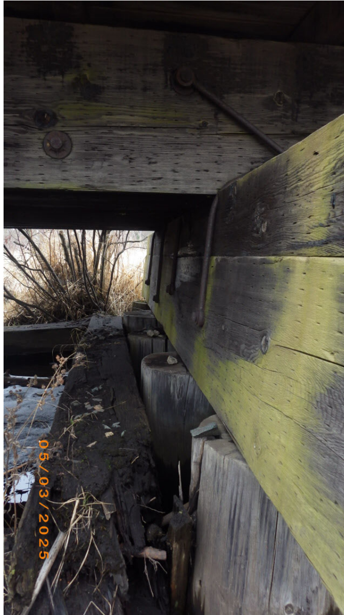
Pier 1 moderate rotation, loss of nearly half of the bearing on piling
