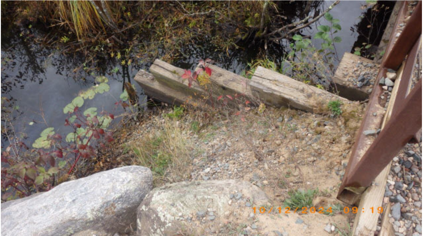
All wingwalls tipping, rotten, unstable shoulders
