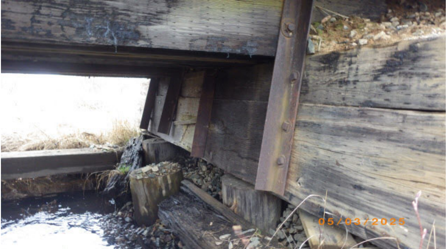
North abutment pile cap tilting back, nearly off piling, fill spilling through
