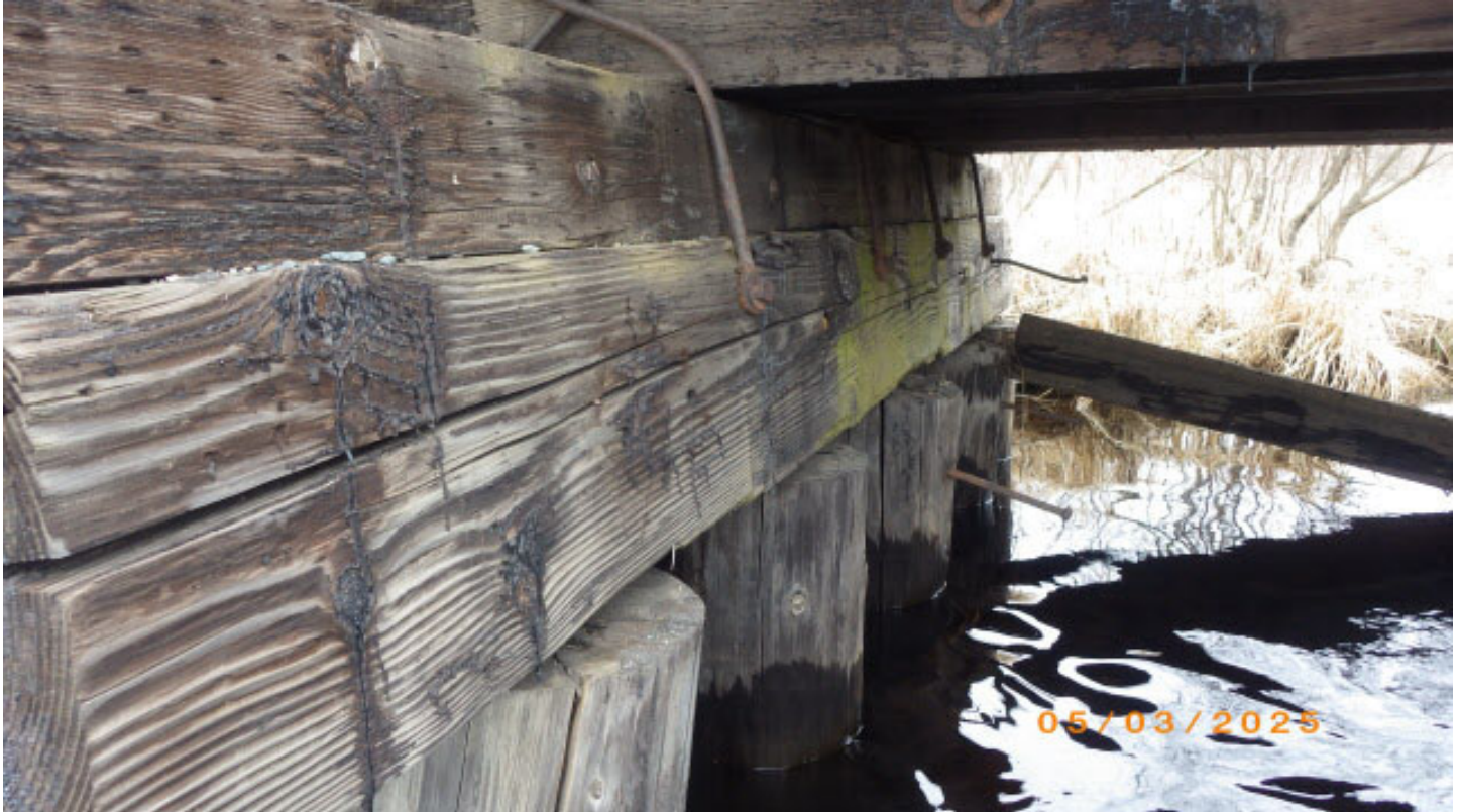
Pier 3 pile cap severe rotation
