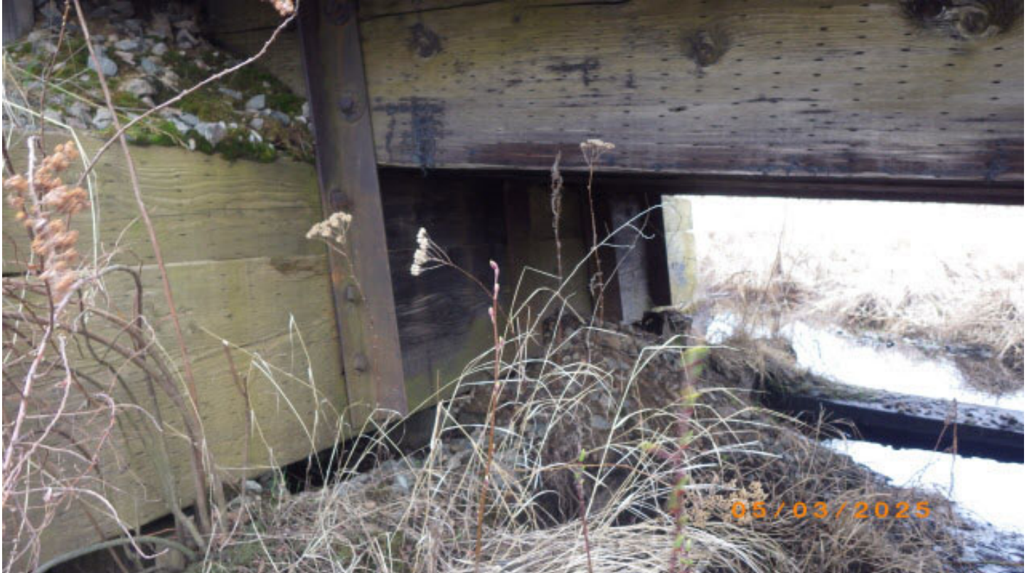
South abutment, pile cap rotated back
