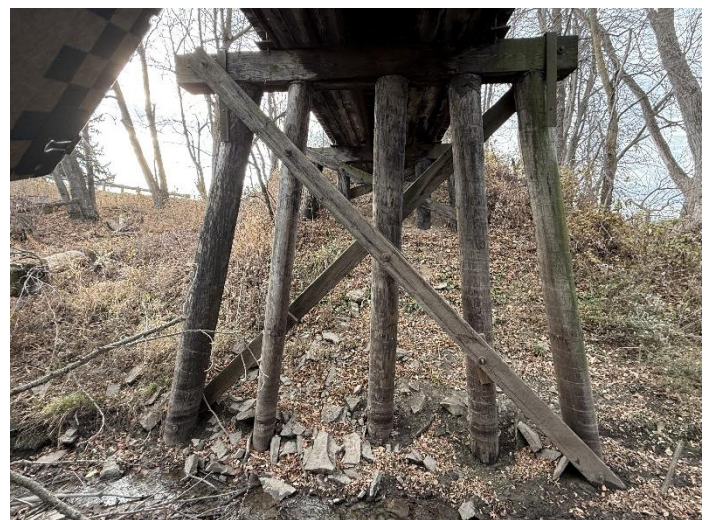
Photo 12 – Pier W2 Looking West.
