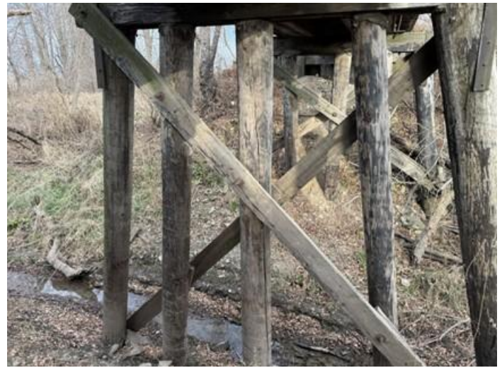
Photo 19 – Pier W2 Looking East.
