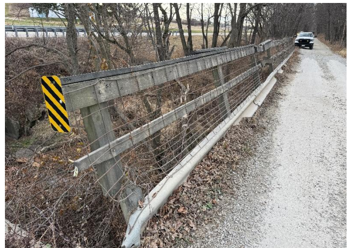
Photo 6 – South Rail Looking West.
