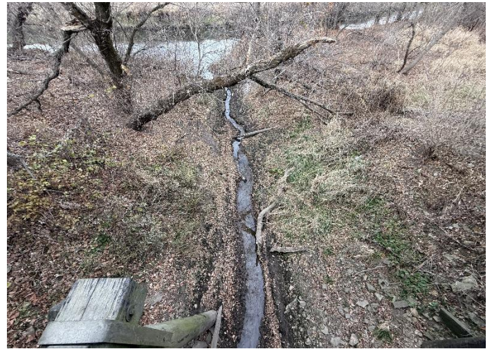
Photo 4 – Downstream Looking North.
