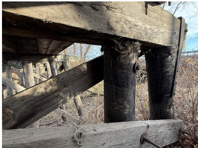
Photo 15 – Pier W1-Pile S2.
