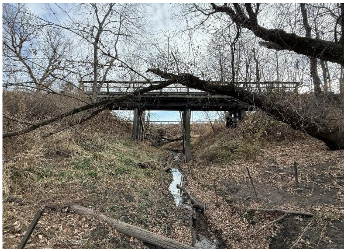
Photo 5 – Side View Looking South.
