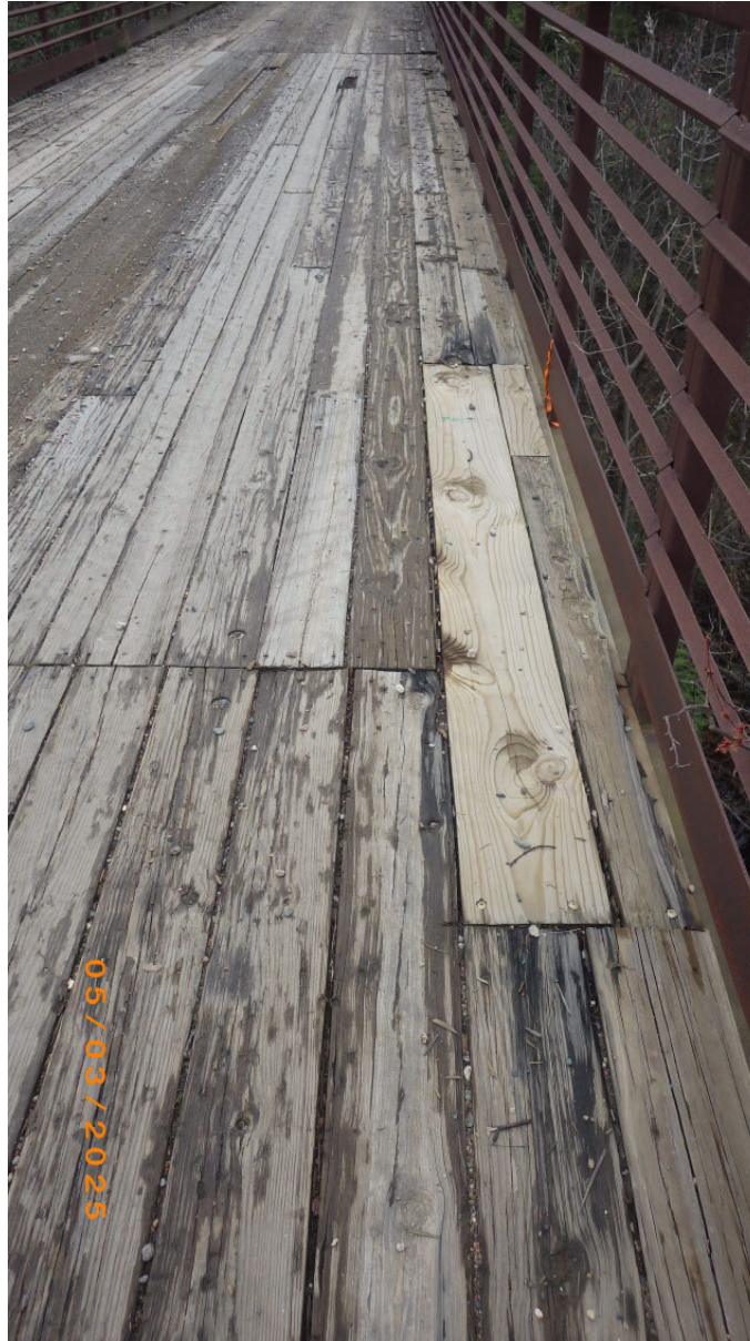
Patched hole at east edge of span 7
