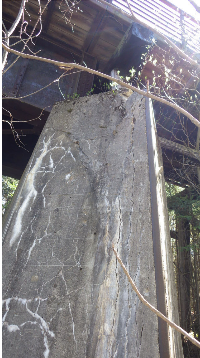
Pier #3 concrete wall with very large spall on upstream nose and top edge with CS3 cracking with rust stained efflorescence throughout
