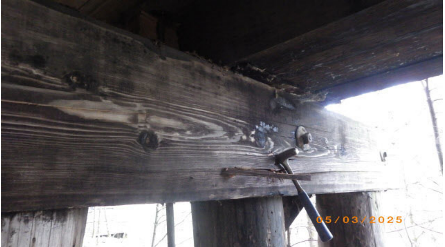
Bent #1, cap rotten / crushing
