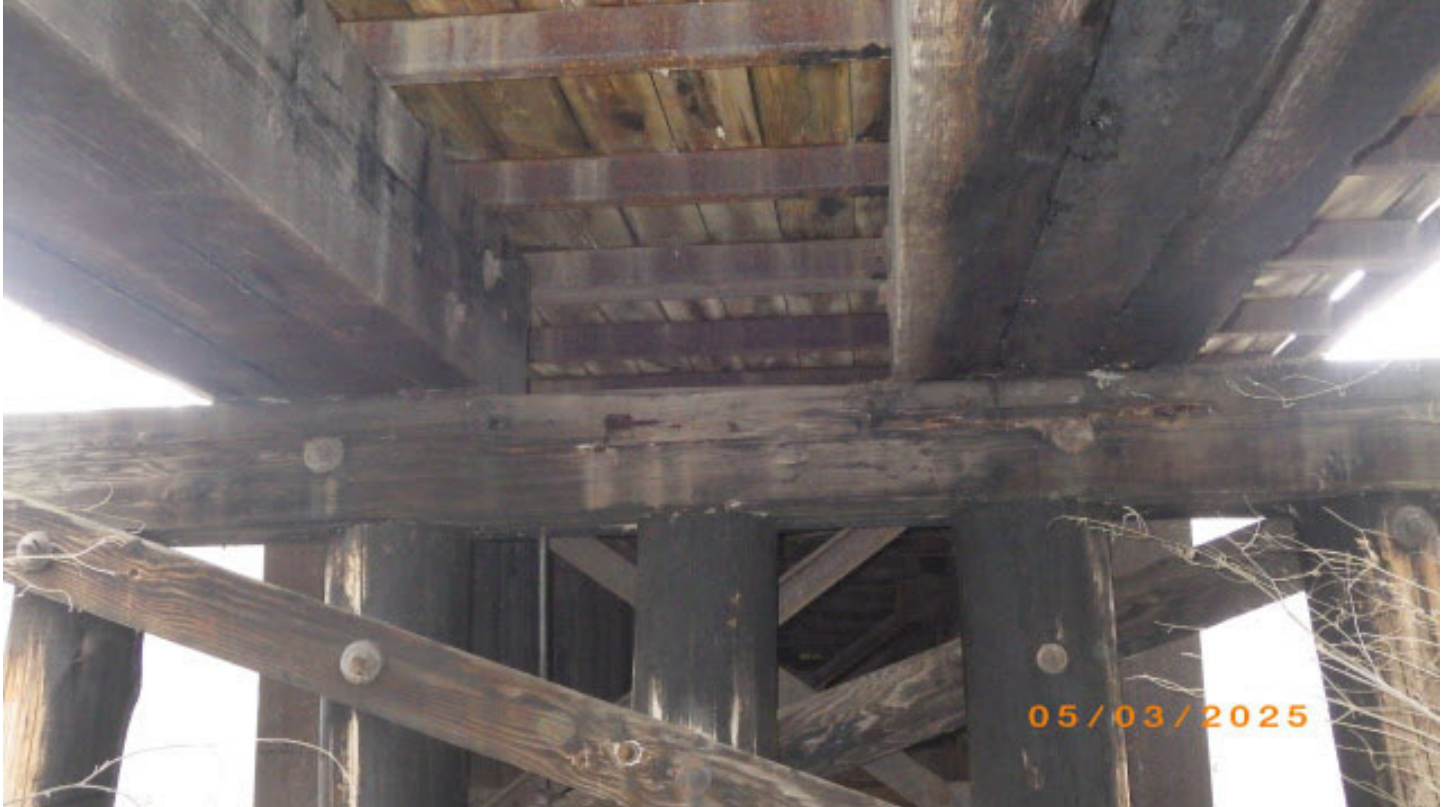
Pier #3, timber cap rotten / crushing (close-up)
