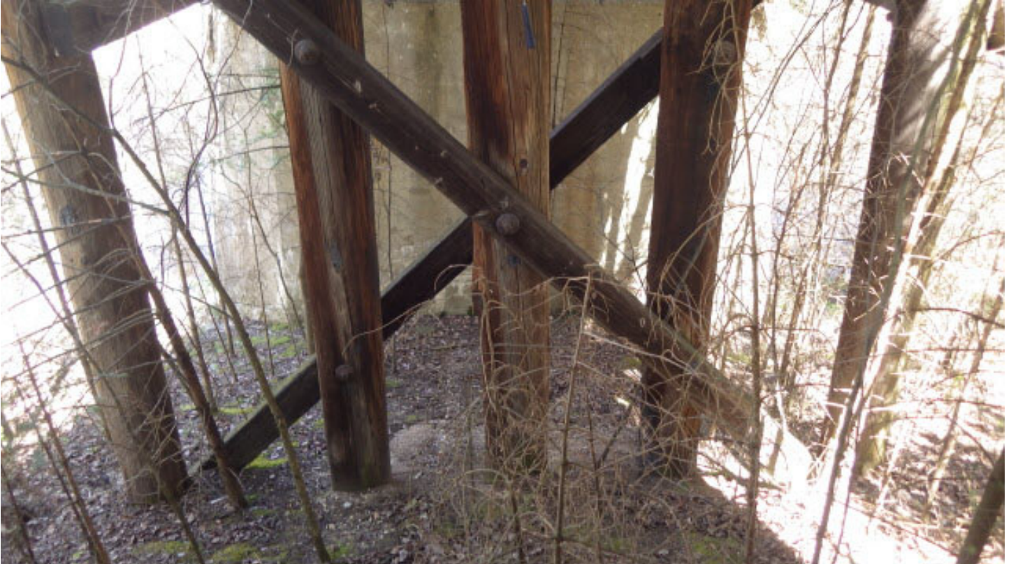
Bent #2 (bottom), center pile hollow
