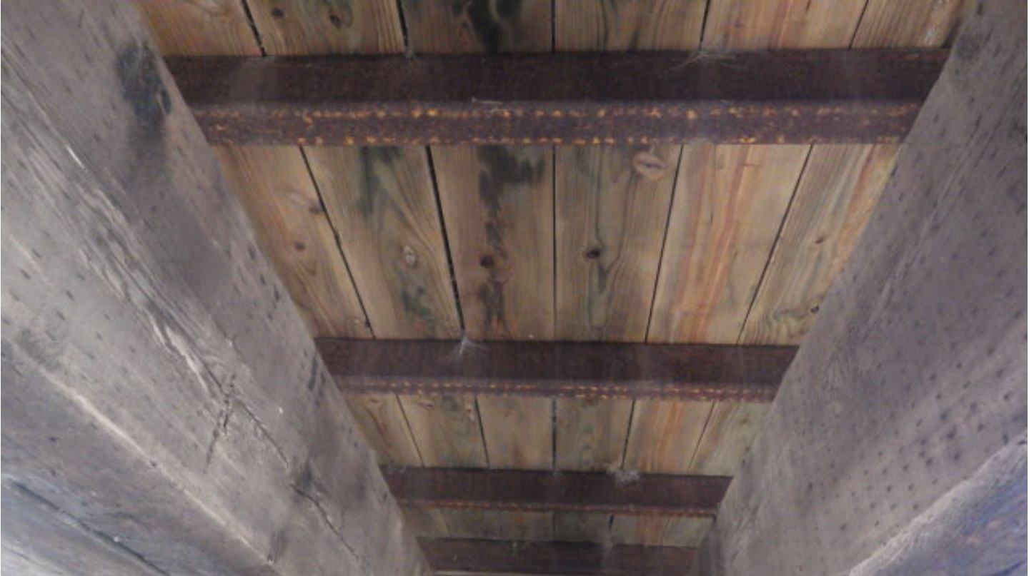
typical underside of deck, scattered black mold.
