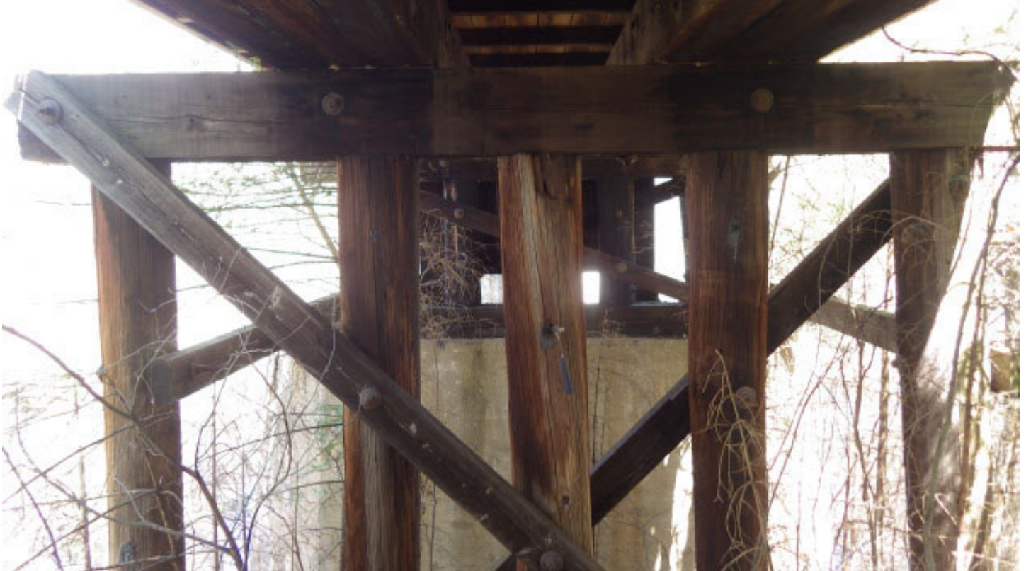
Bent #2 (top), center pile hollow
