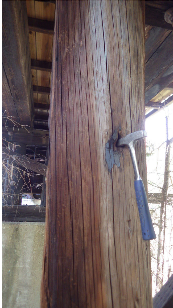
Bent #2, center pile hollow
