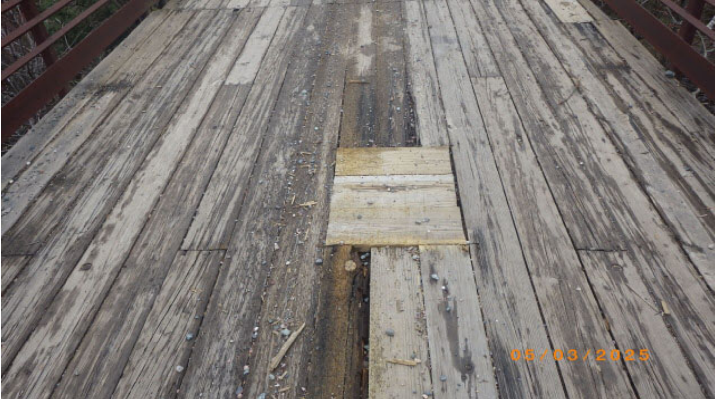
Patched hole near center of bridge
