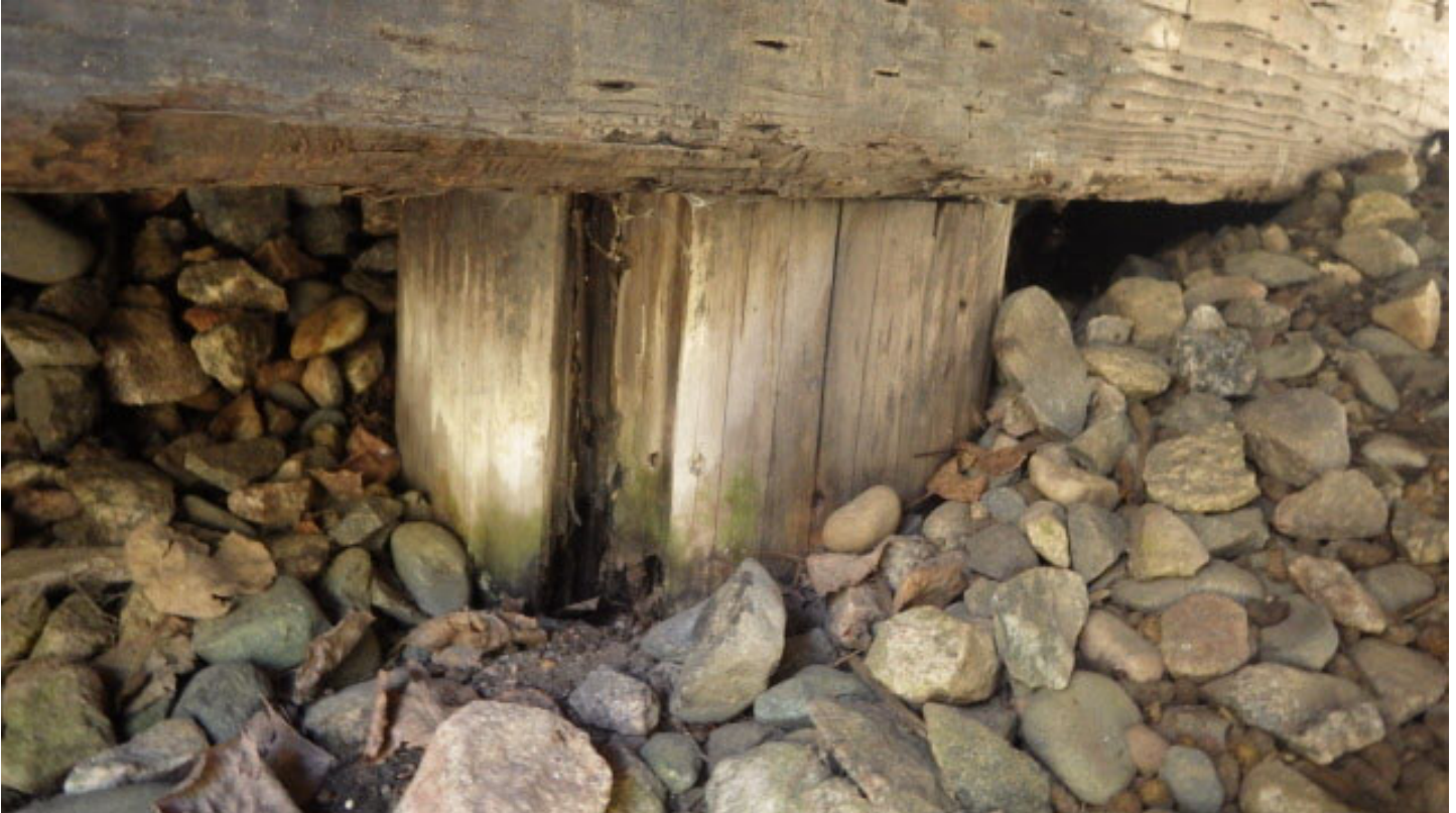
South abutment rotten piling
