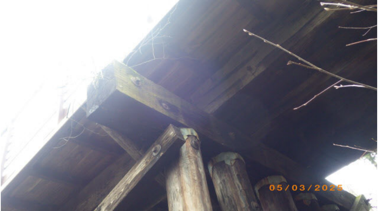
Bent #9 cap is rotten / crushing
