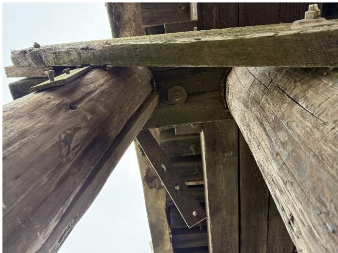
Photo 15 – Pier W2 Cap-Piles S5-S4.
