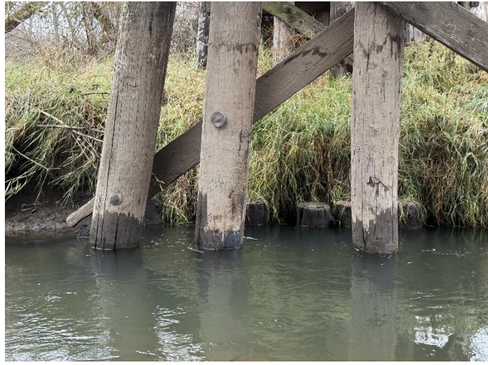
Photo 19 – Pier W3 Looking East-Piles W5-W3.
