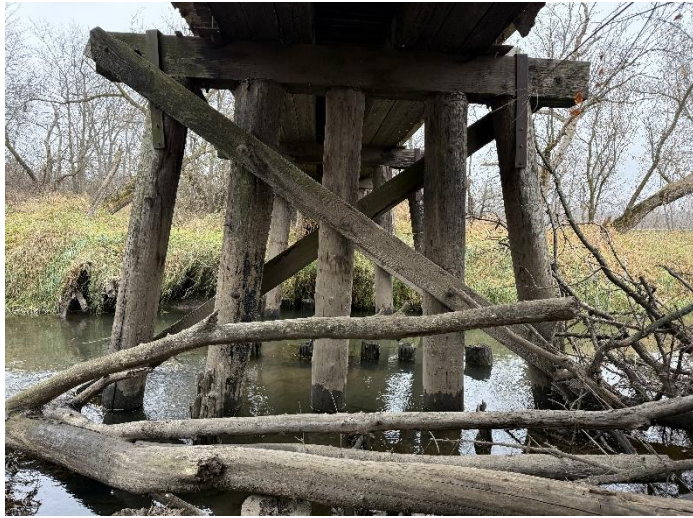
Photo 13 – Pier W2 Looking East.
