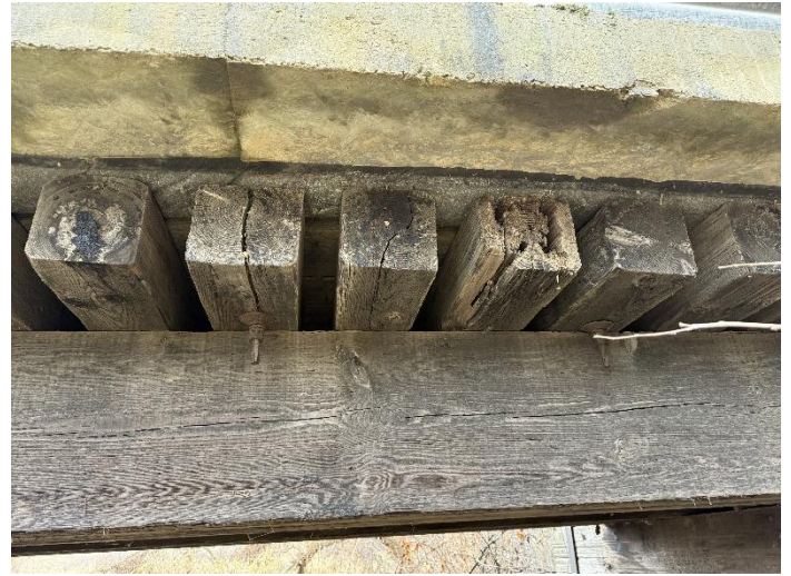
Photo 8 – North Edge of Deck in Span W1.
