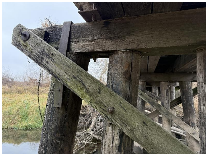
Photo 21 – Pier W3 Looking West-Piles W3-W1.
