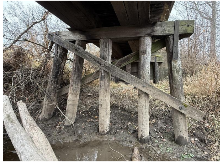
Photo 14 – Pier W1 Looking East.
