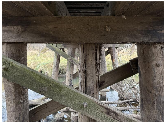
Photo 11 – Pier W1-Pile S3.
