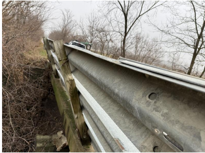
Photo 7 – North Rail Looking East.
