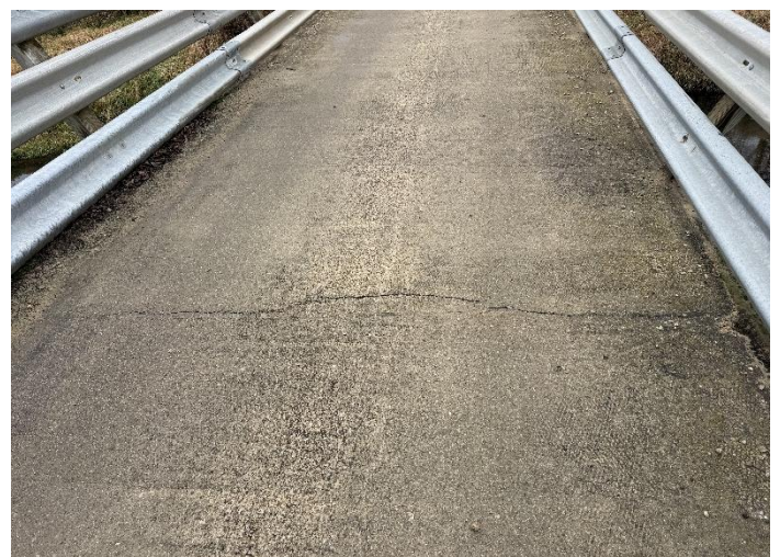
Photo 6 – Deck Looking South.
