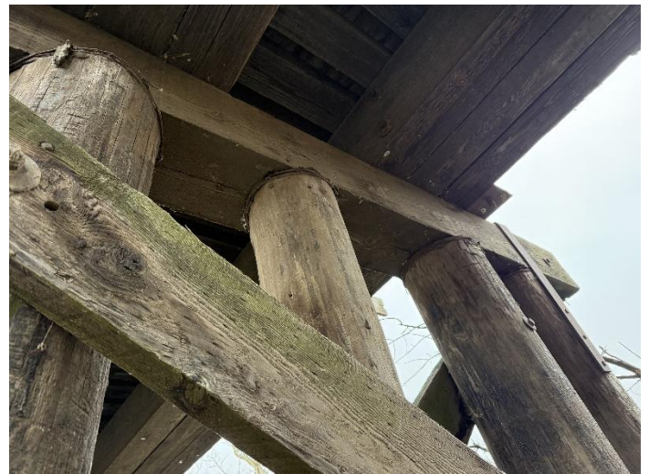
Photo 16 – Pier W2 Cap-Piles S4-S1.
