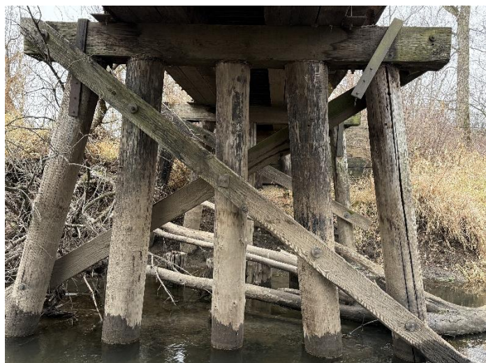
Photo 23 – Pier W3 Looking West.
