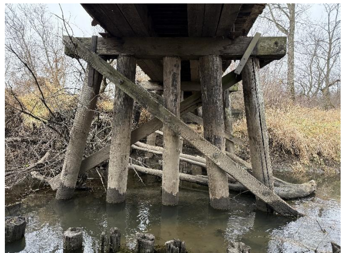
Photo 22 – Pier W3 Looking West.
