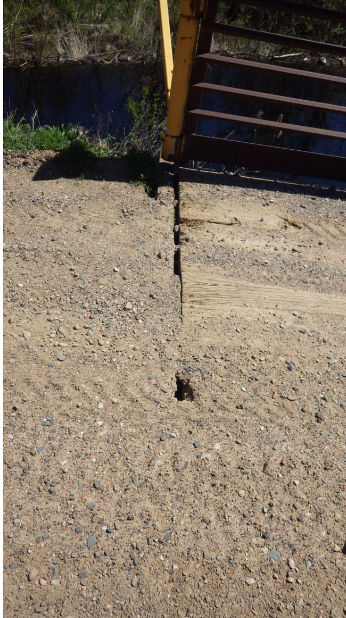
Gap between backwall and deck, north end
