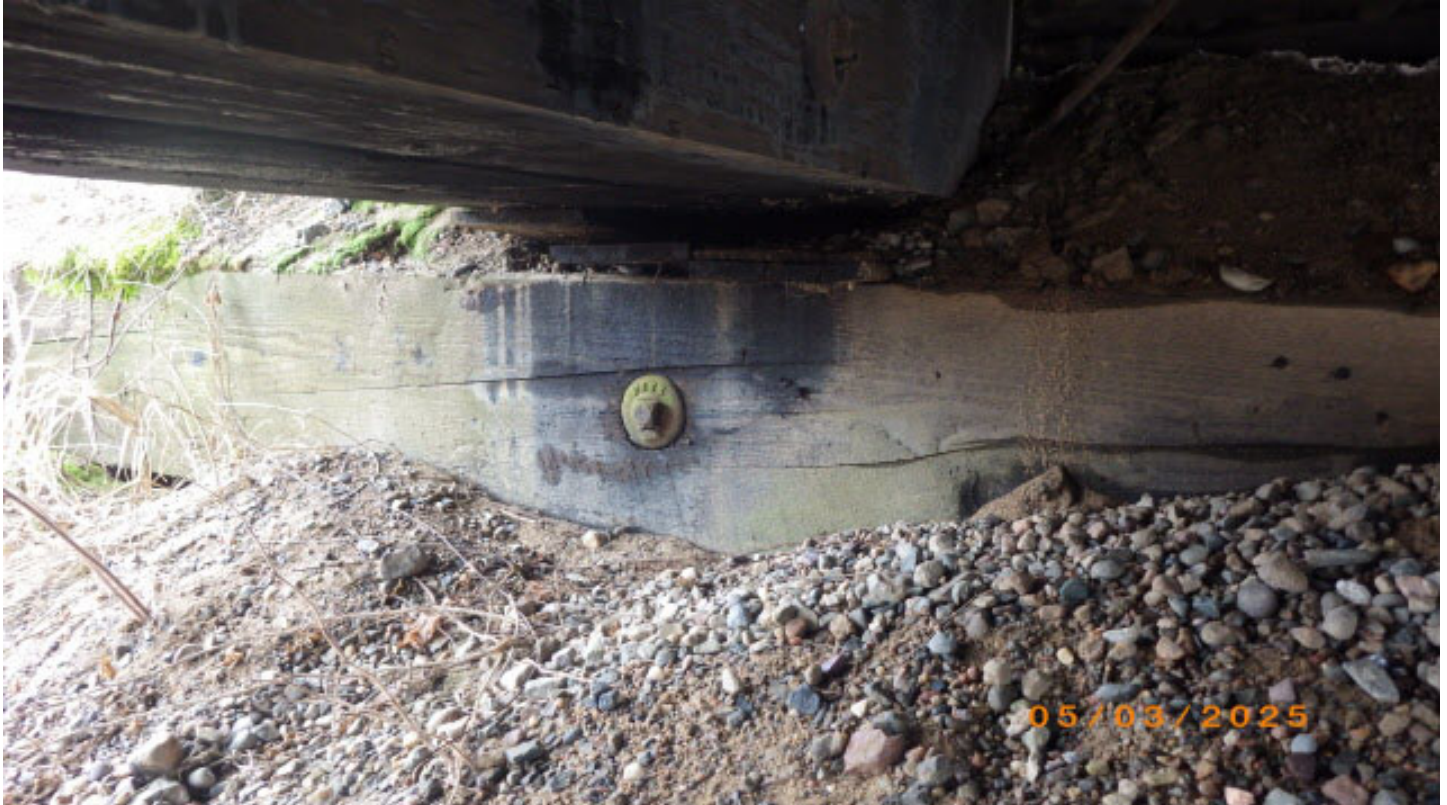
South abutment cap rotten
