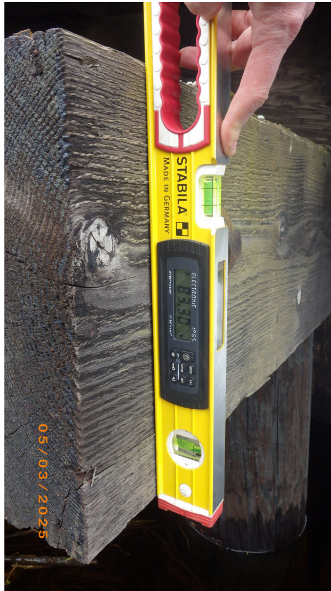
Bent #1 tipping southward. 83.3° measured at east end of pile cap.
