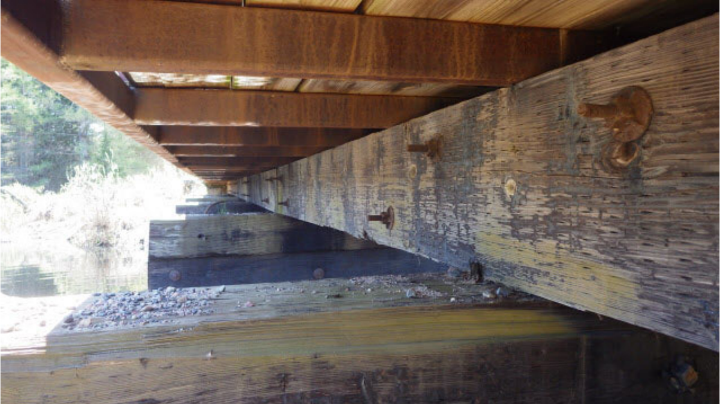
Wide checking on exterior girders
