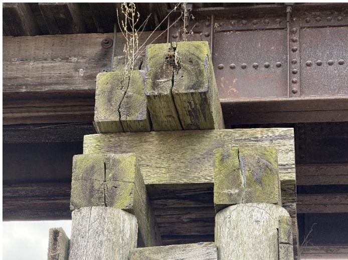
Photo 31 – Pier W4 Looking South.
