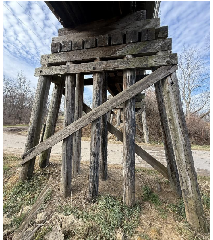
Photo 14 – Pier W4 Looking West.
