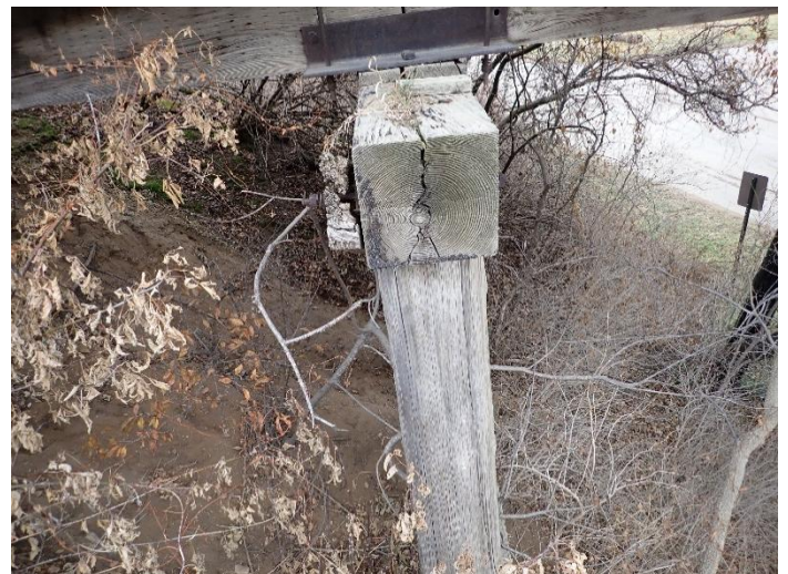
Photo 42 – Pier W1 Looking North.
