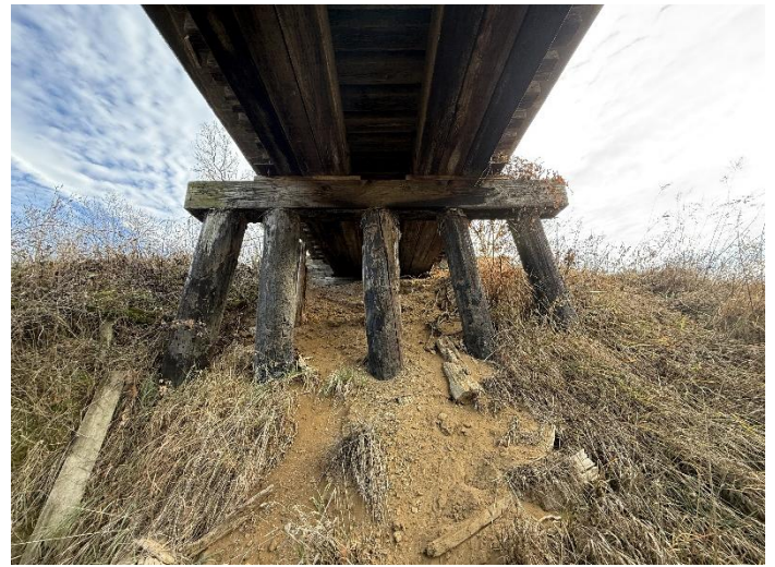
Photo 16 – Pier W6 Looking East.
