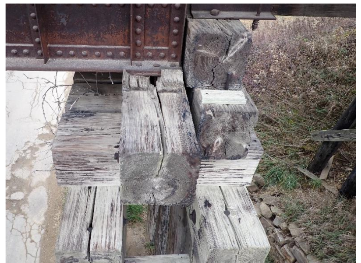
Photo 46 – Pier W4-South End.
