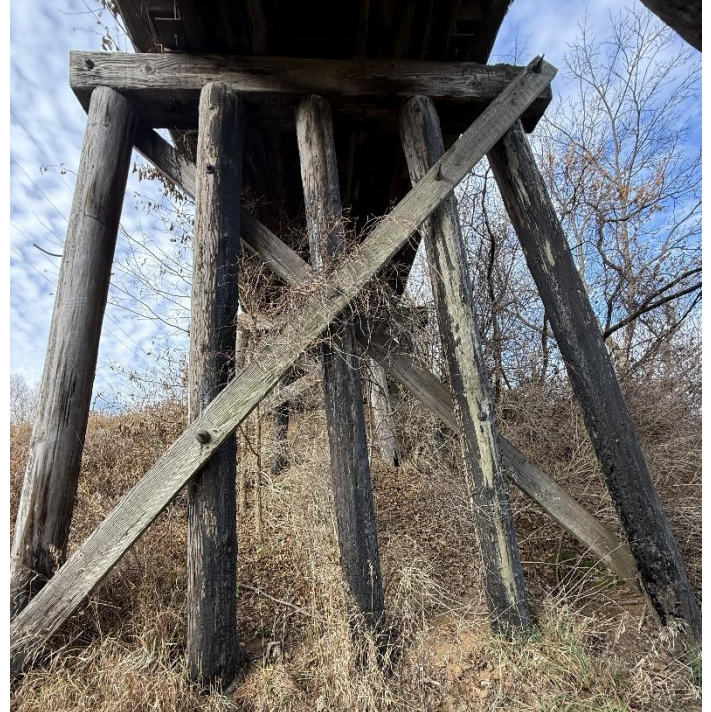
Photo 10 – Pier W2 Looking West.
