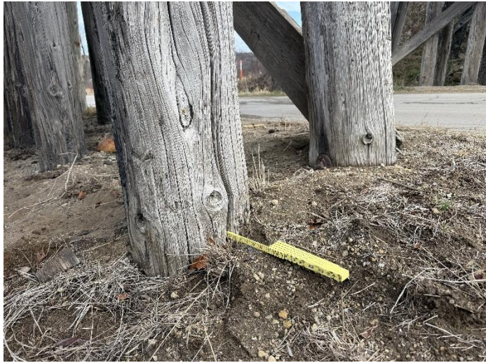
Photo 25 – Pier W3-E. Row-Pile S5.
