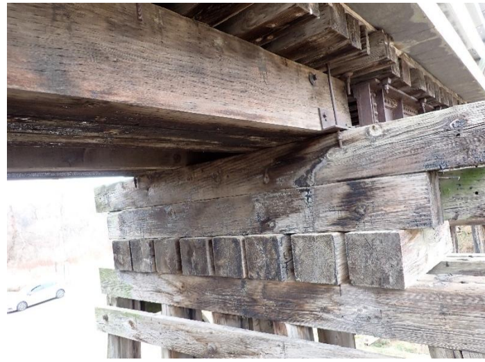
Photo 43 – Pier W3 Looking East.
