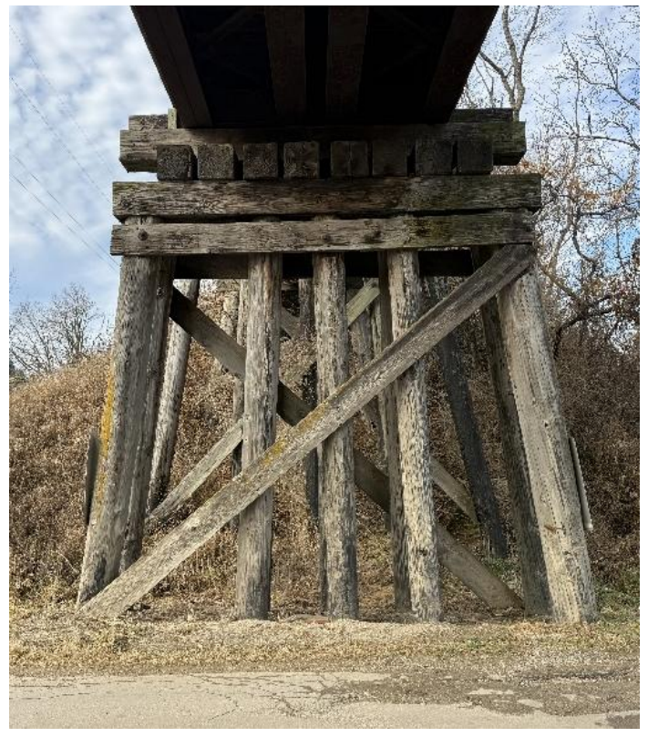
Photo 12 – Pier W3 Looking East.
