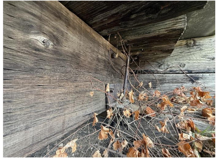
Photo 38 – South Beam Over East Abutment.
