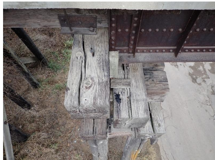
Photo 45 – Pier W3-South End.
