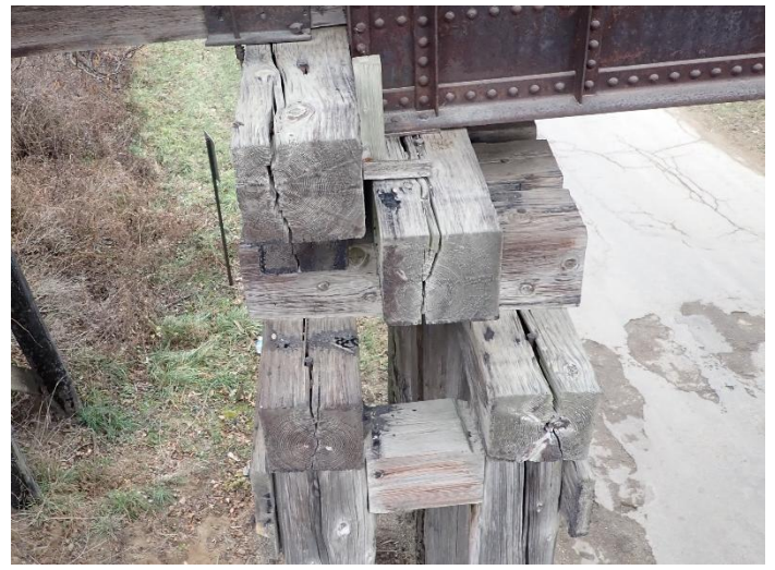
Photo 44 – Pier W3 Looking North.
