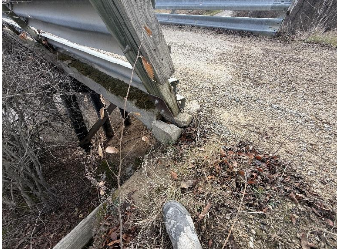
Photo 7 – Northwest Corner of Deck.
