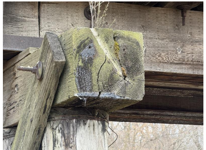
Photo 32 – Pier W5 Looking South.
