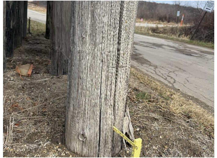
Photo 26 – Pier W3-E. Row-Pile S1.
