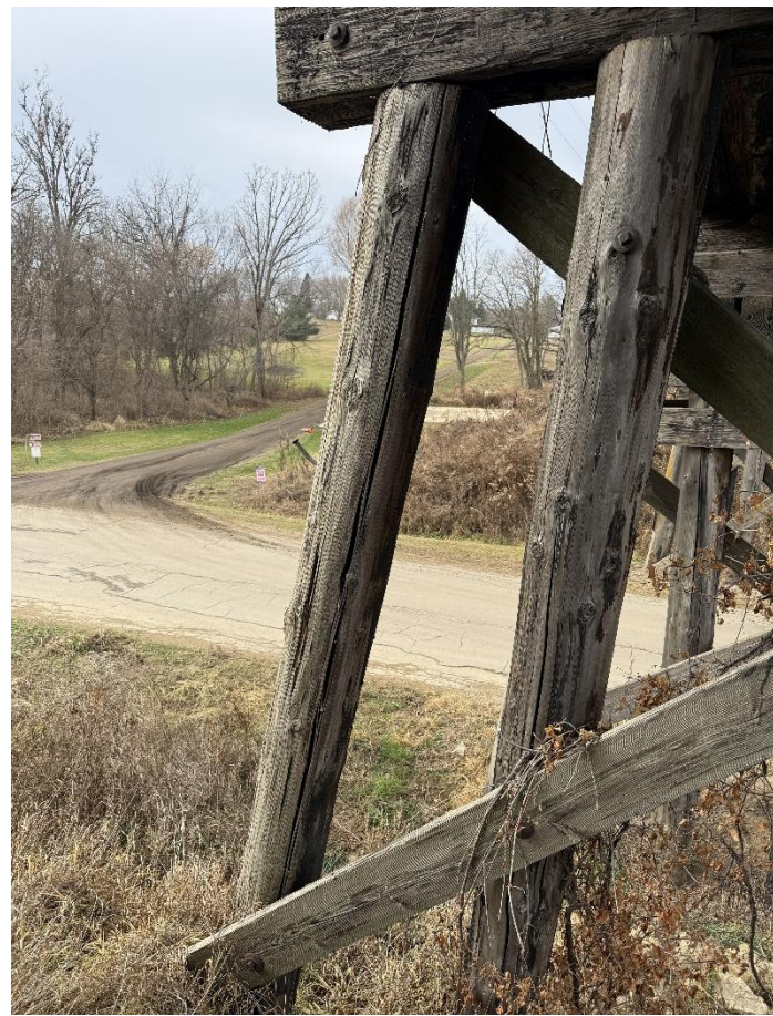
Photo 33 – Pier W5-Pile S1 Looking East.
