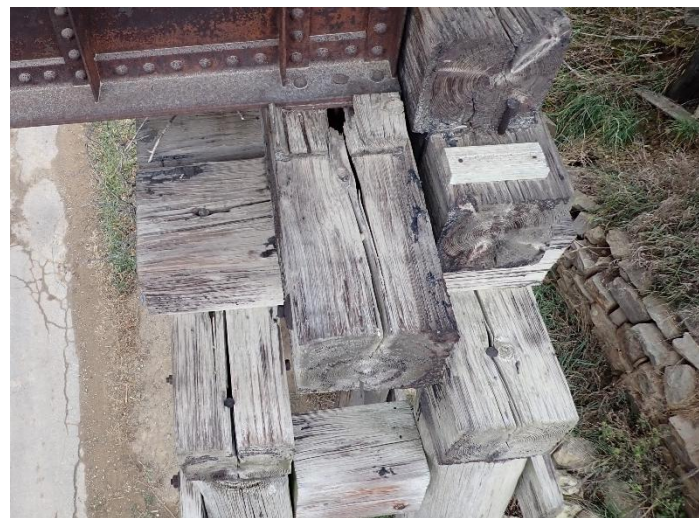
Photo 47 – Pier W4-South End.
