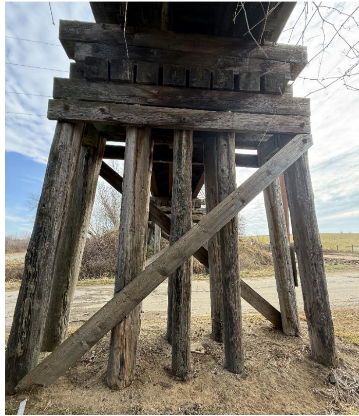
Photo 11 – Pier W3 Looking West.
