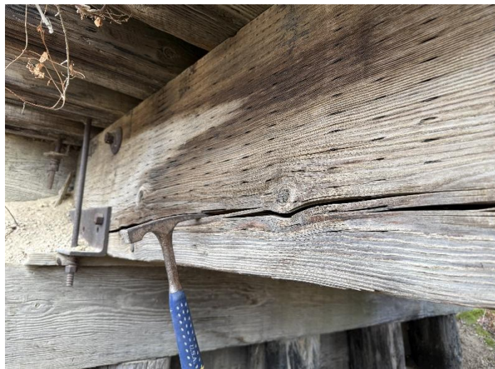
Photo 19 – Span W1-S. Beam-S. Face Over W. Abut.
