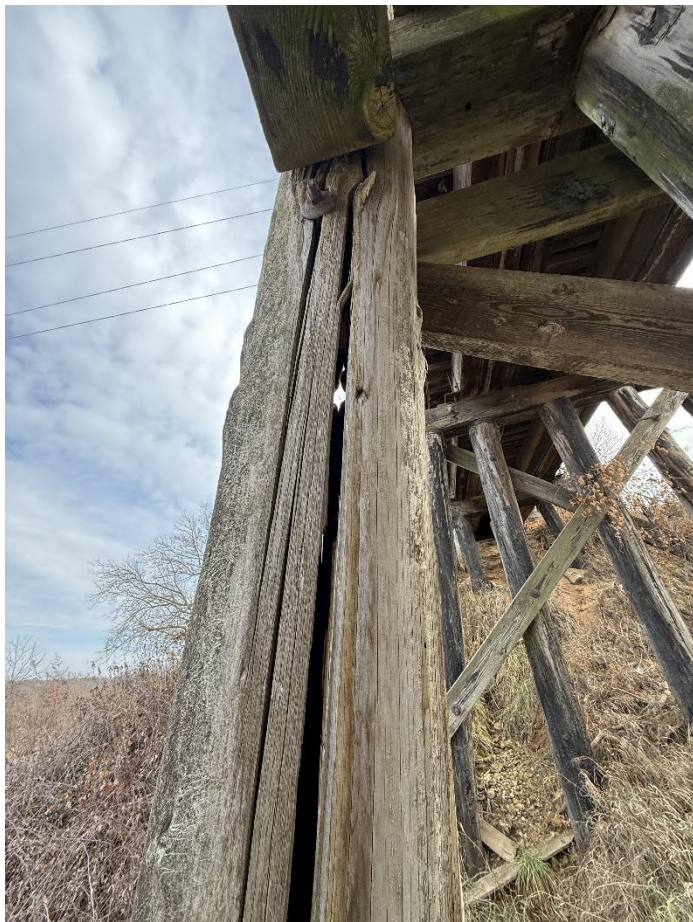
Photo 27 – Pier W4-E. Row-Pile S5.
