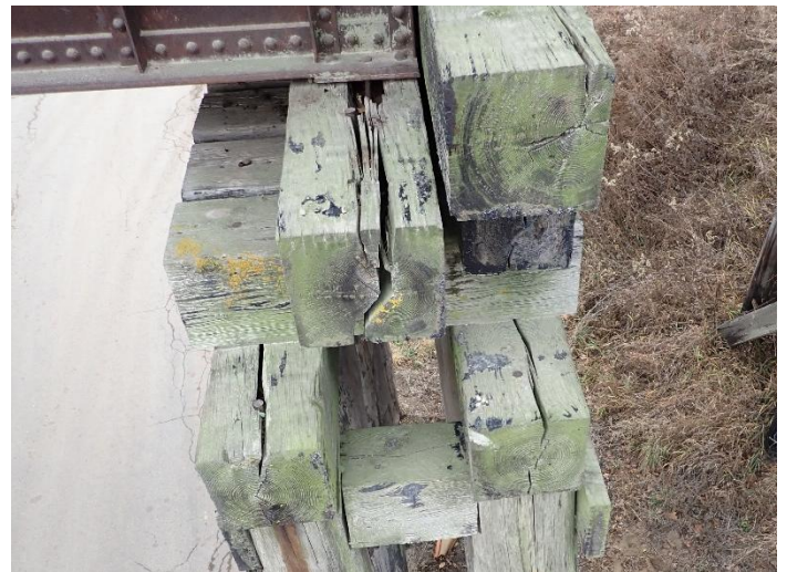
Photo 40 – Pier W3 Looking South.
