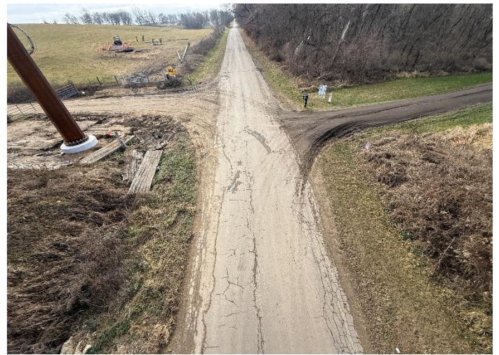
Photo 4 – Allen Road Looking South.
