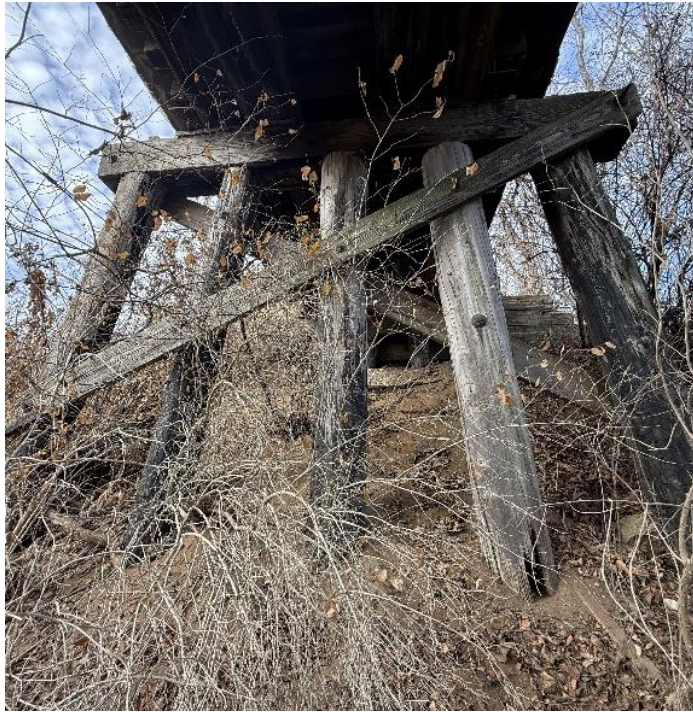
Photo 9 – Pier W1 Looking West.
