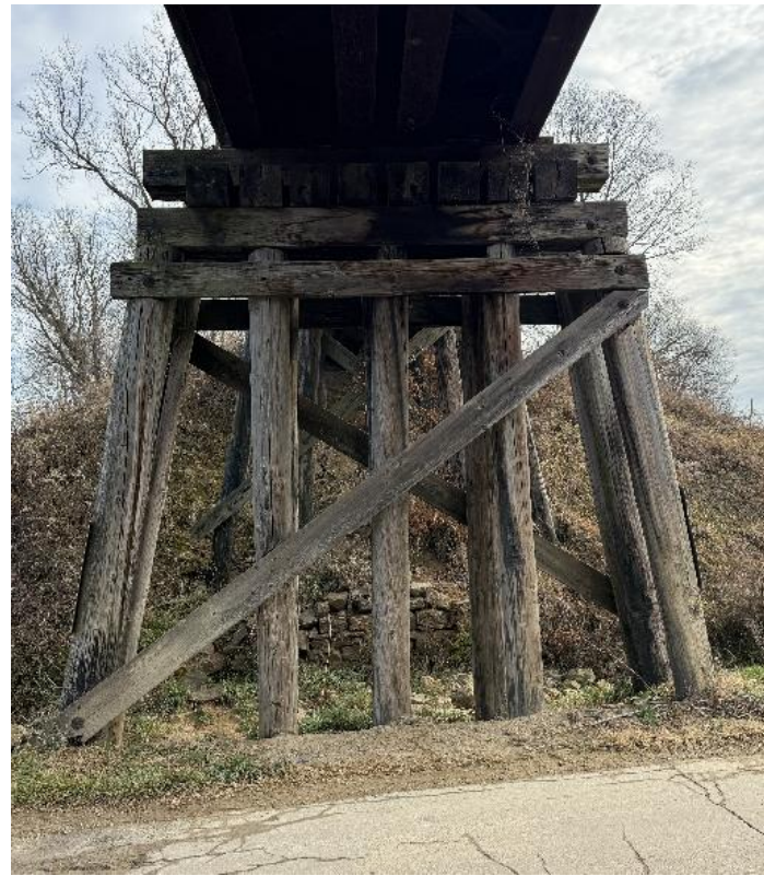
Photo 13 – Pier W4 Looking East.
