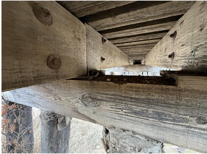
Photo 37 – Beams Over Pier W6 Looking West.
