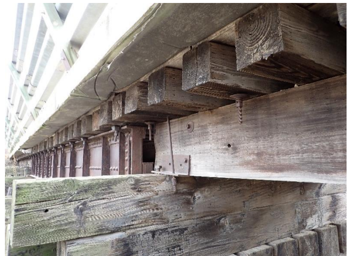
Photo 48 – Span W5-South Beam Looking East.
