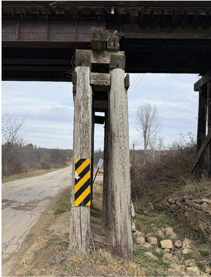
Photo 29 – Pier W4 Looking North.
