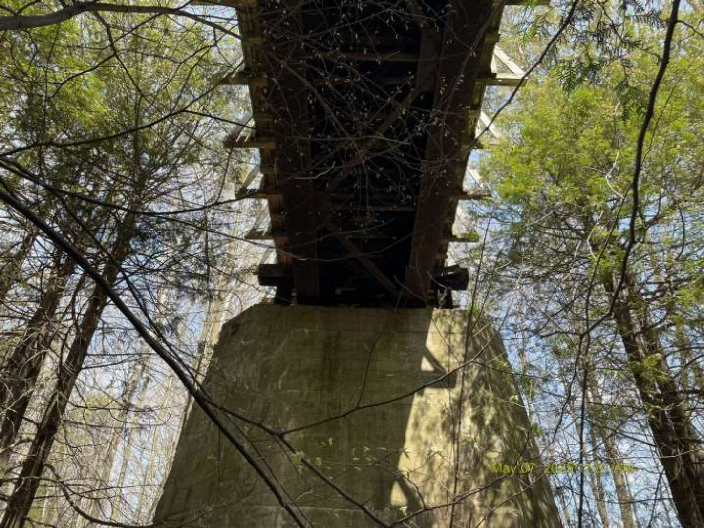
Pier 4 looking north
