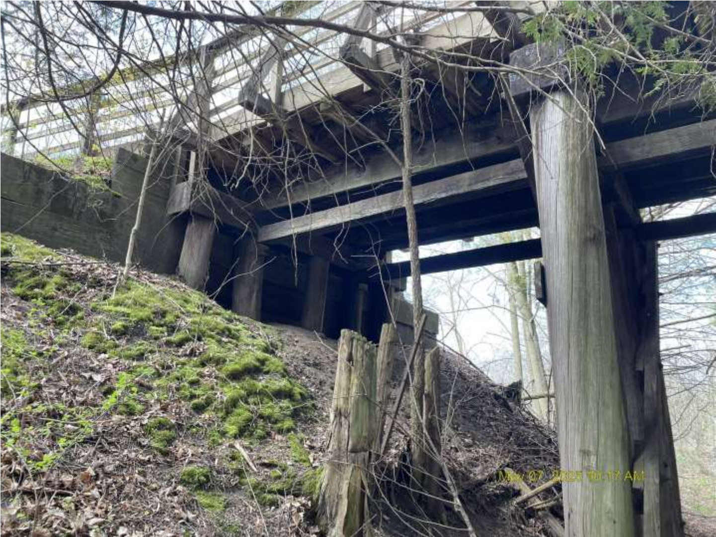
Looking SW between S. Abut. & Pier 1
