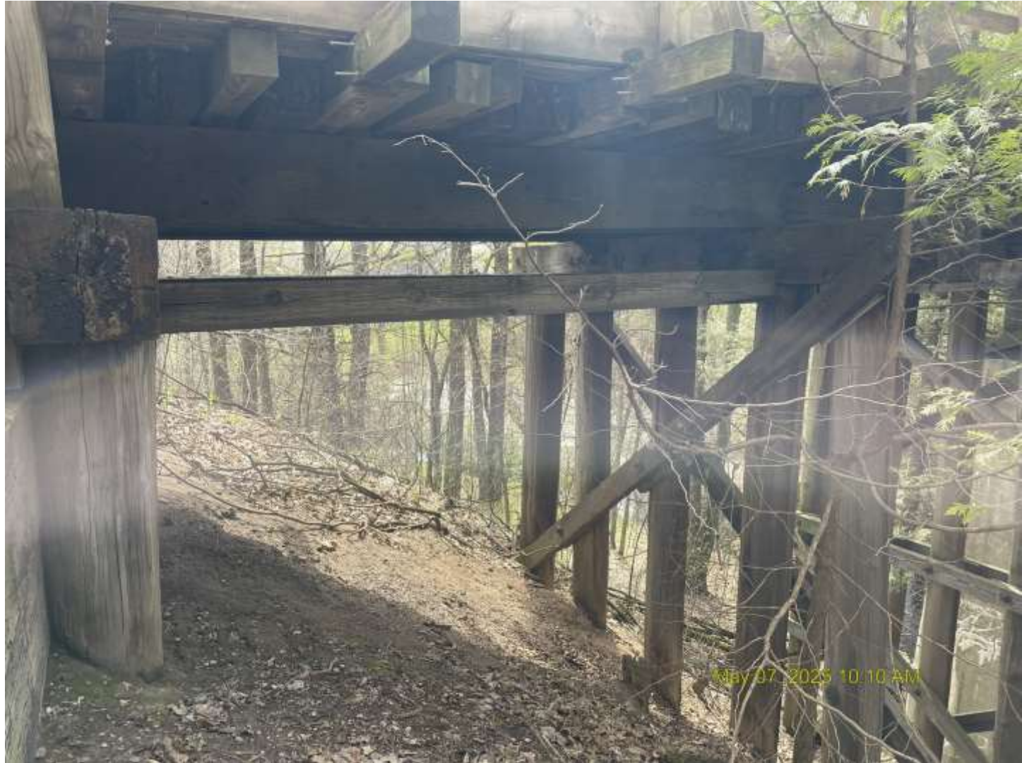
Looking east between N. Abut. & Pier 6
