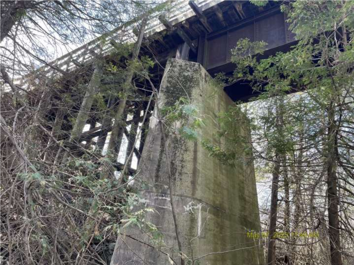
Looking up at Pier 3 (north side)
