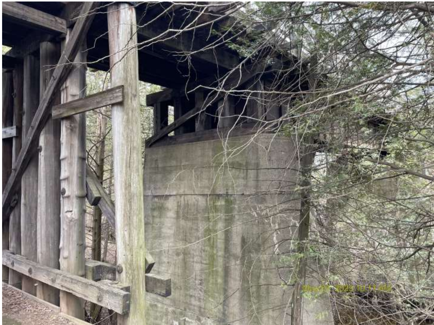
Looking NW between Pier 2 and Pier 3
