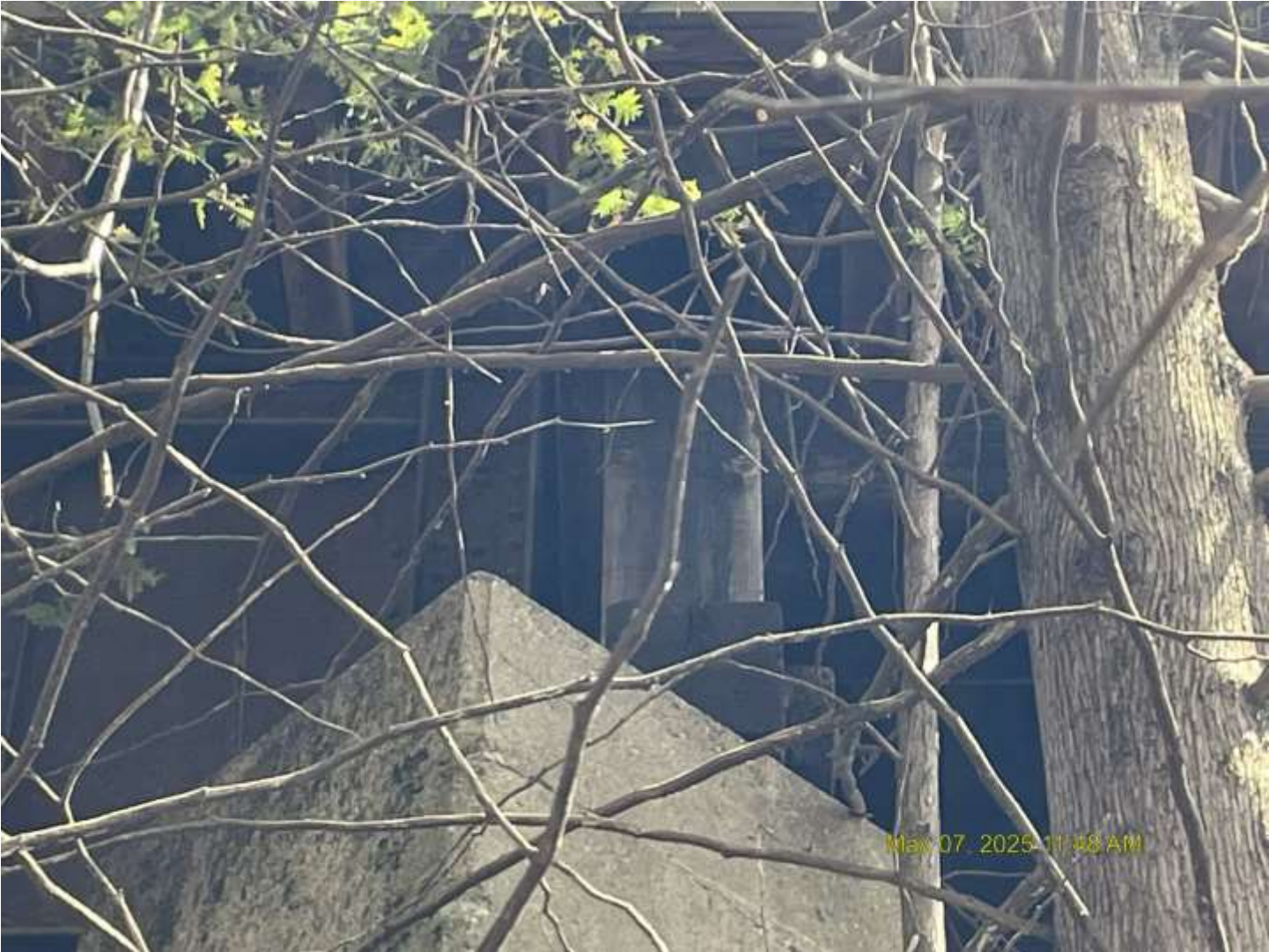
Pier 3 detail west side at girders
