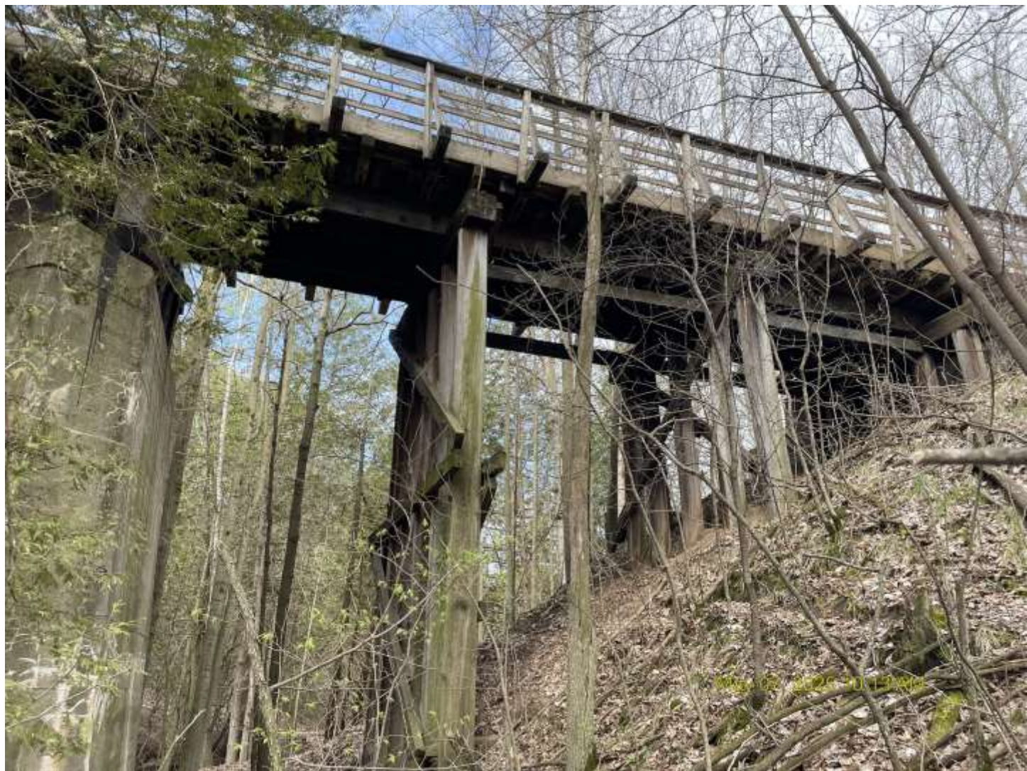
Looking west between Pier 4 and N. Abut.
