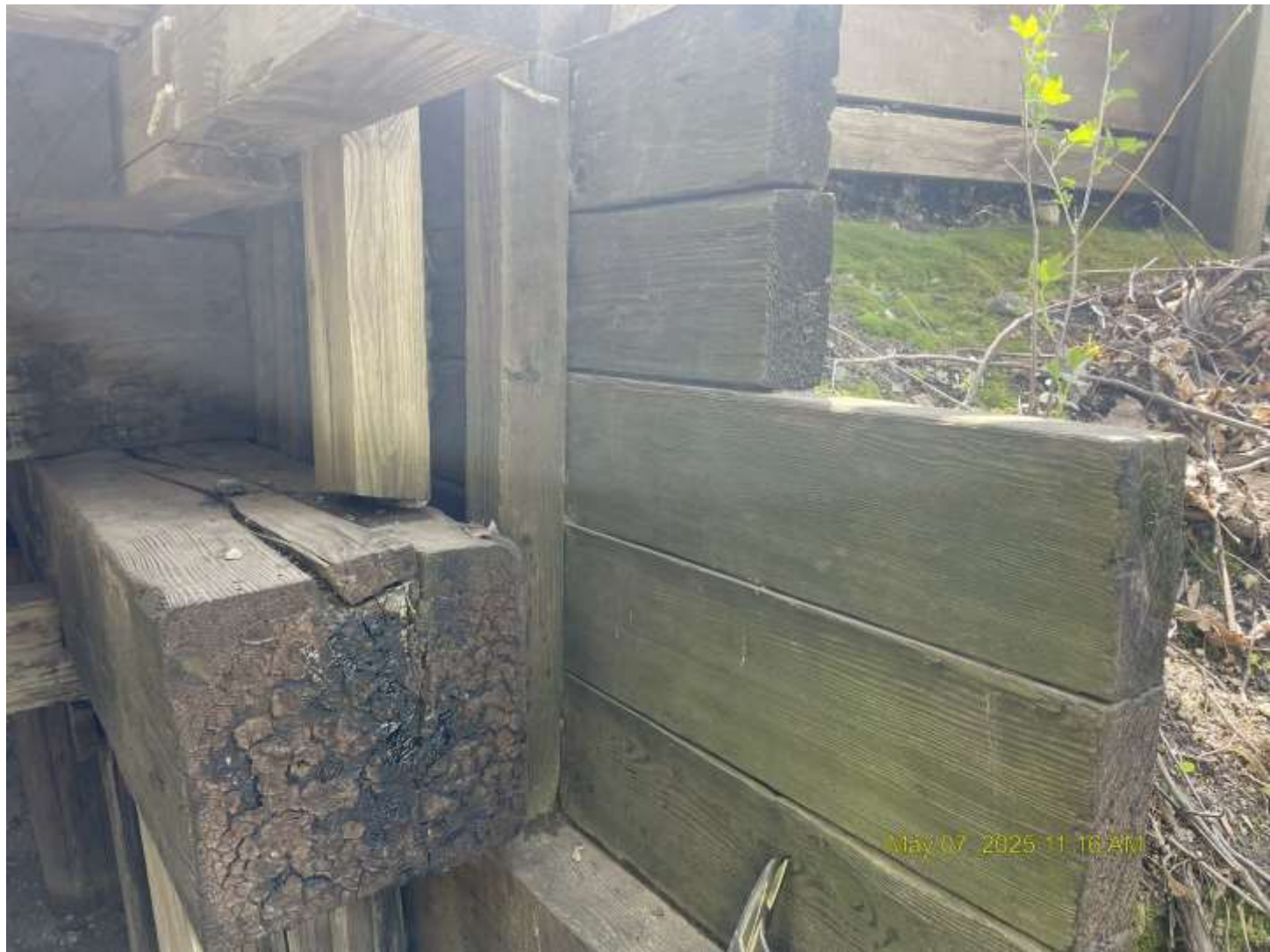
Looking at S. Abut. west side
