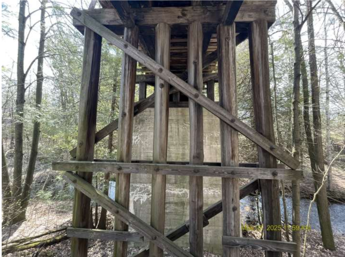
Looking south at Pier 5
