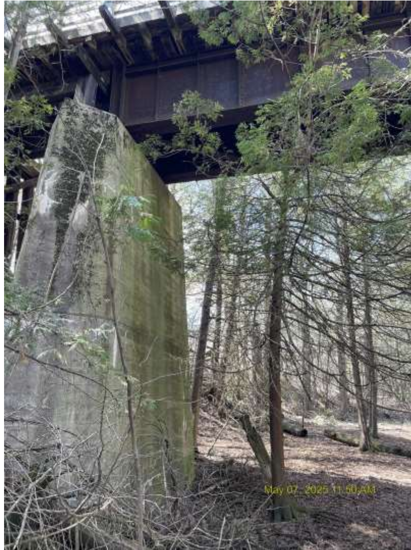
Pier 3 east side – note tree removal
