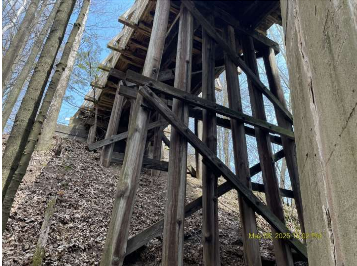
Looking NE at Pier 5
