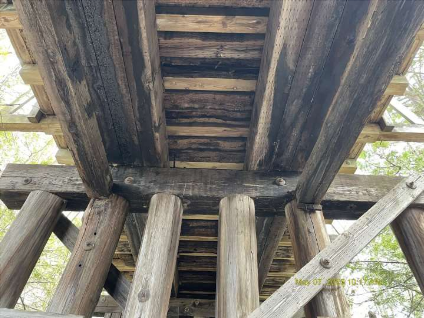
Looking north at underside of bridge at Pier 2
