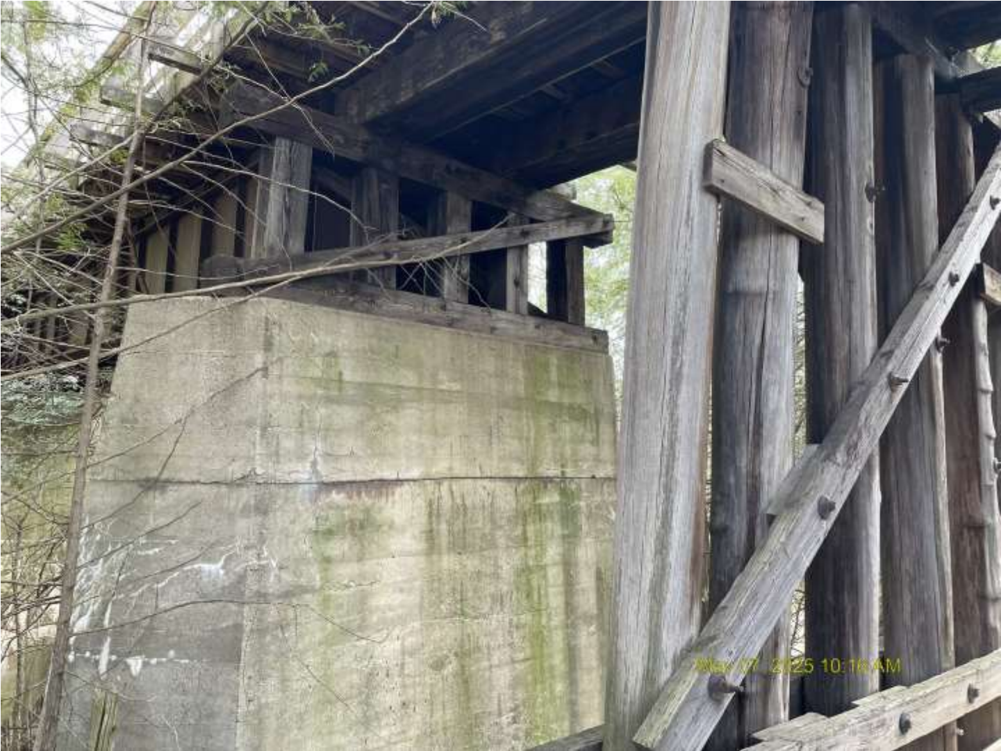
Looking NE between Pier 2 and Pier 3
