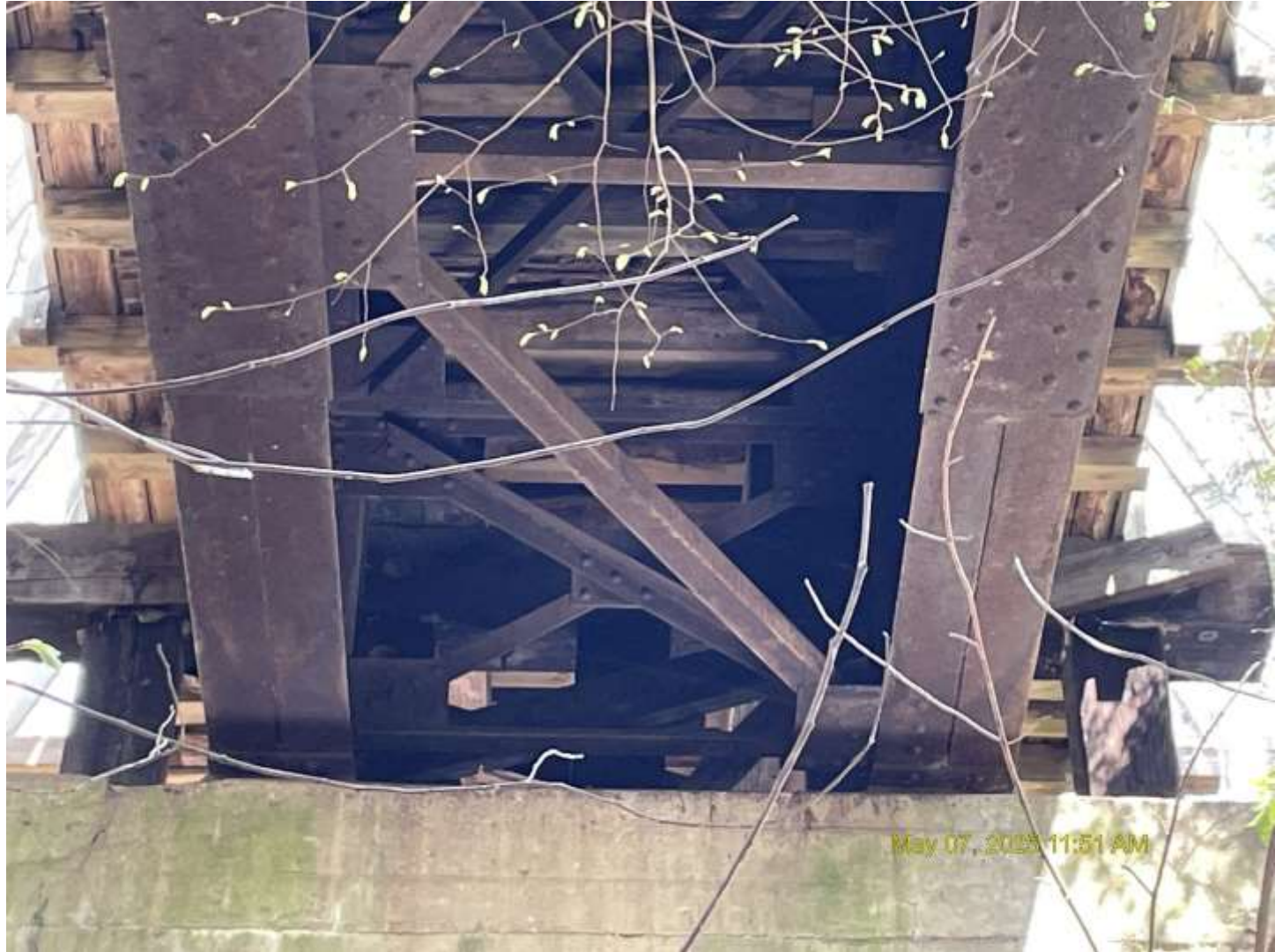
Pier 4 looking north
