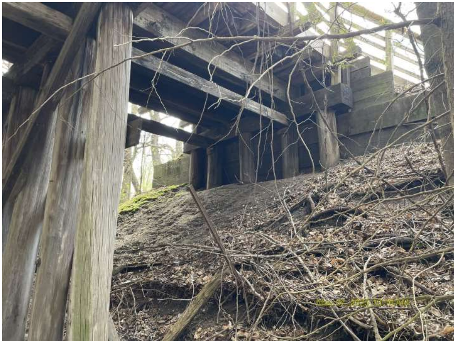
Looking SE between S. Abut. & Pier 1
