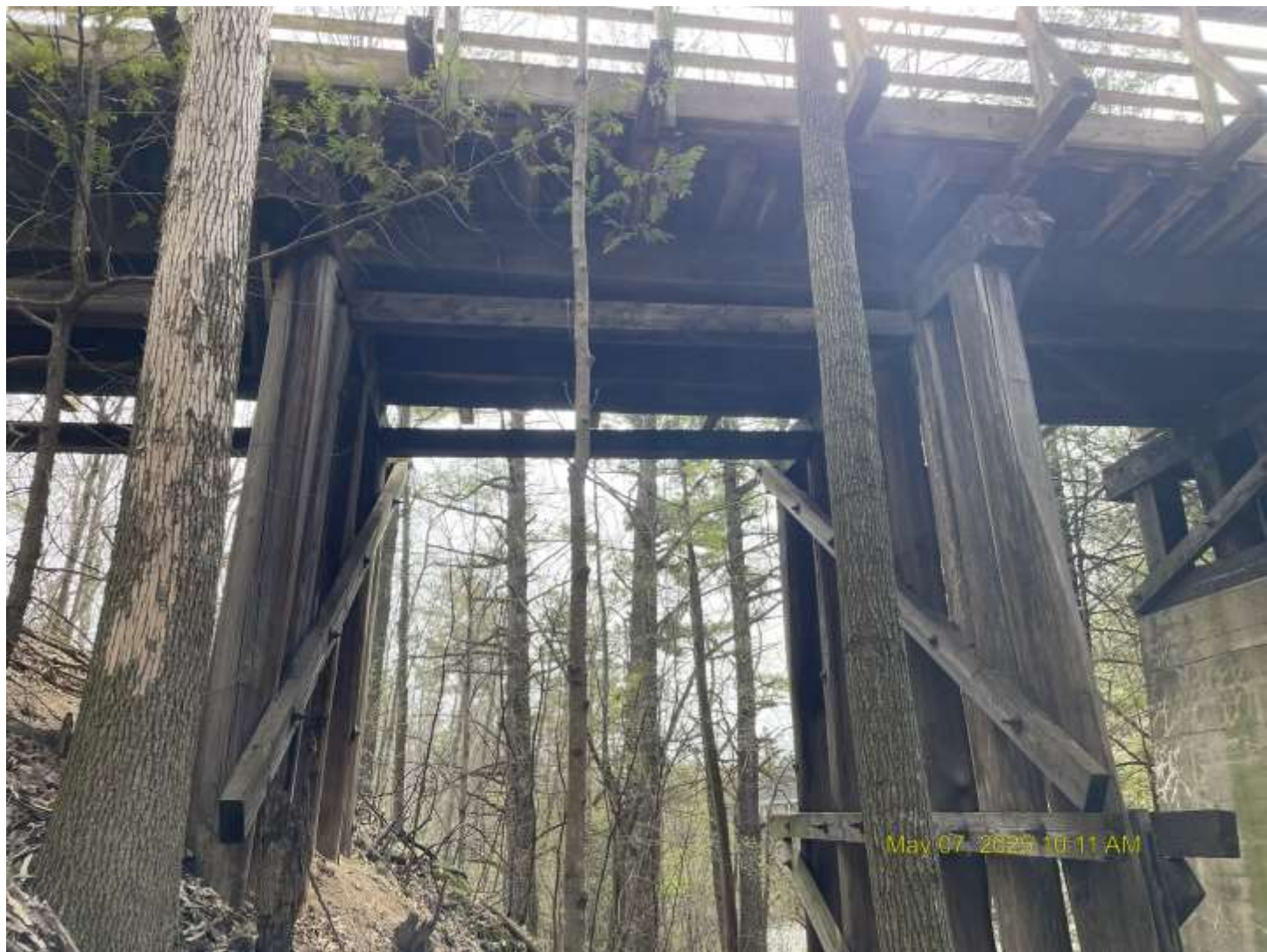
Looking east between Pier 6 and Pier 5
