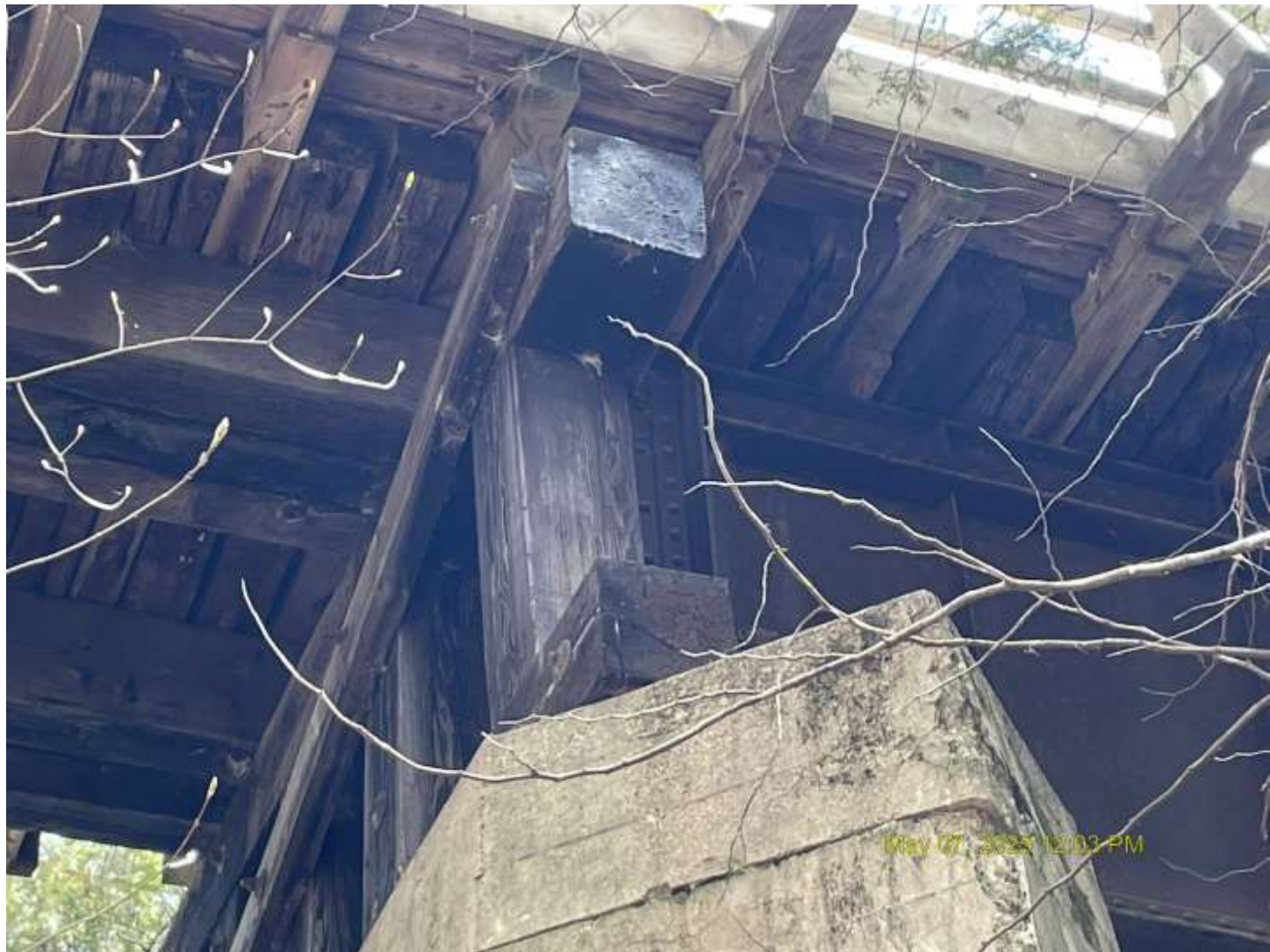
Looking up (east) at Pier 4
