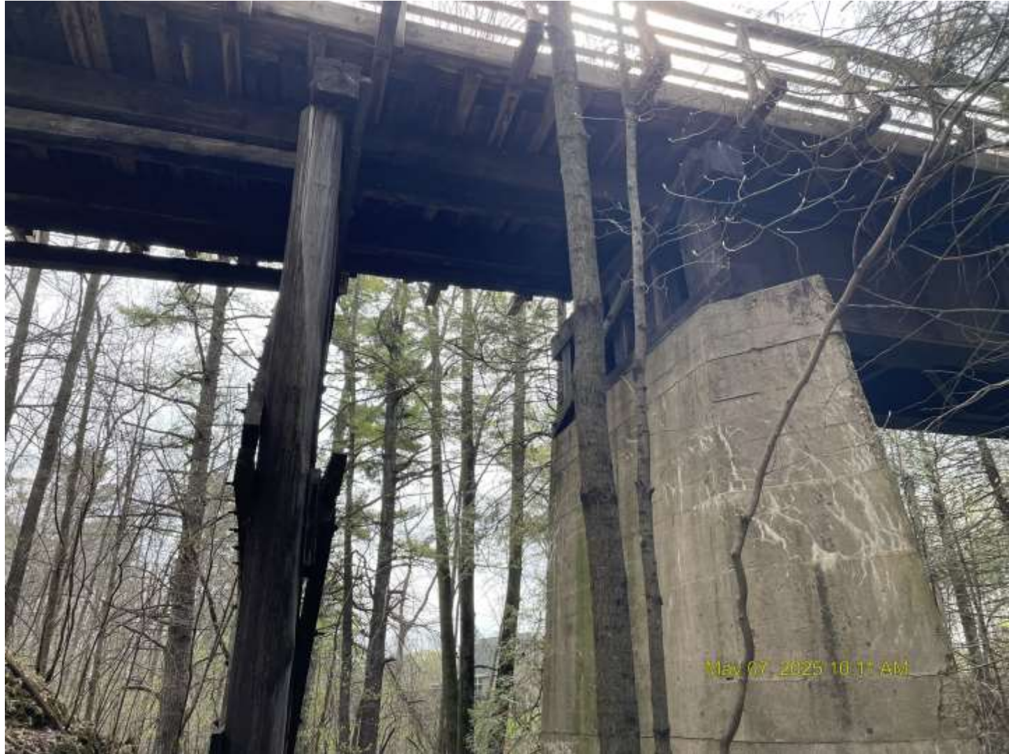
Looking east between Pier 5 and Pier 4
