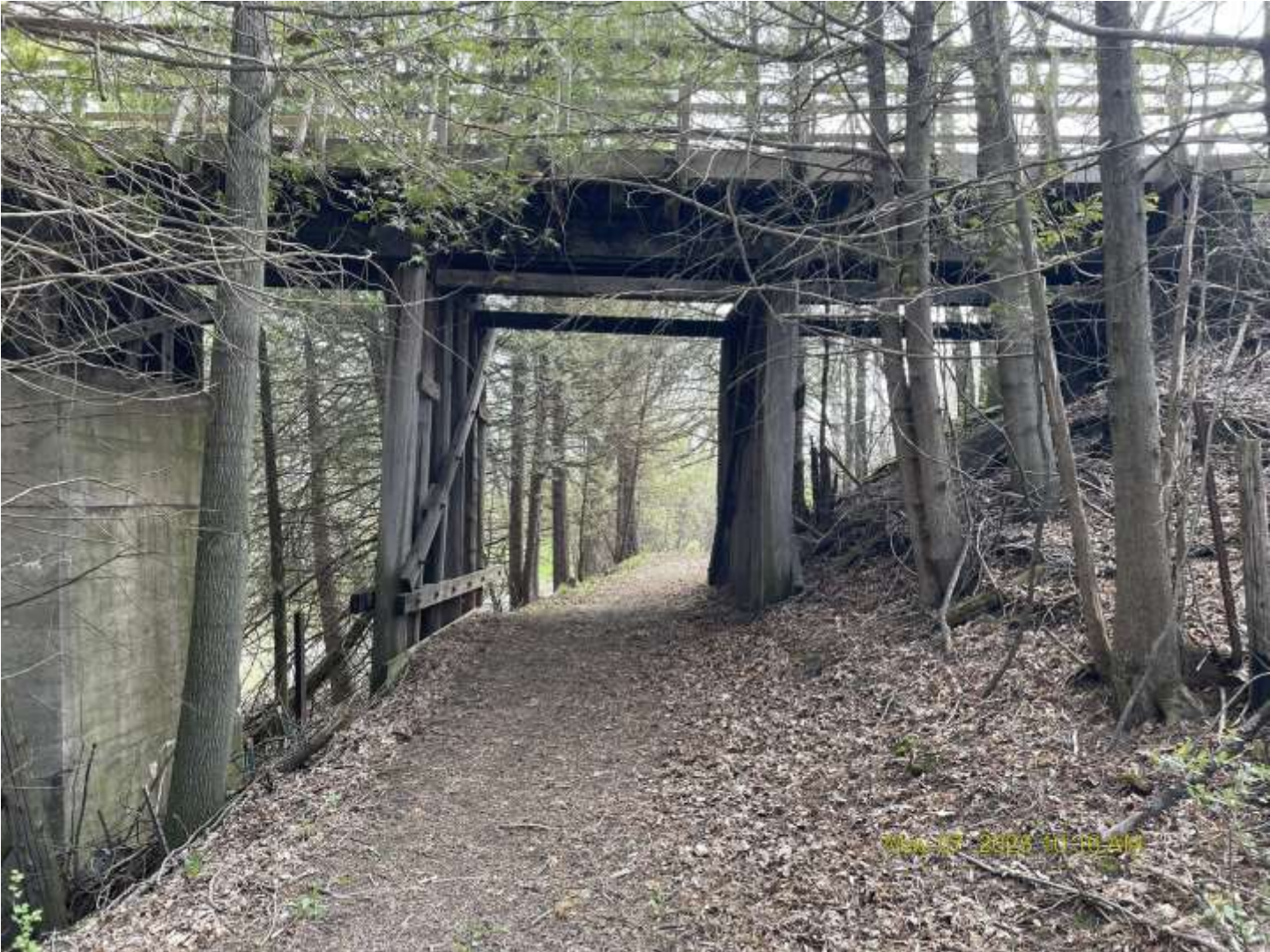
Looking east between S. Abut. & Pier 3
