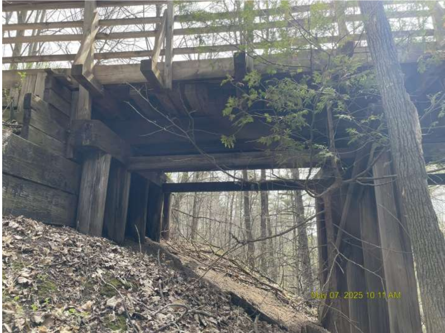
Looking east between N. Abut. & Pier 6
