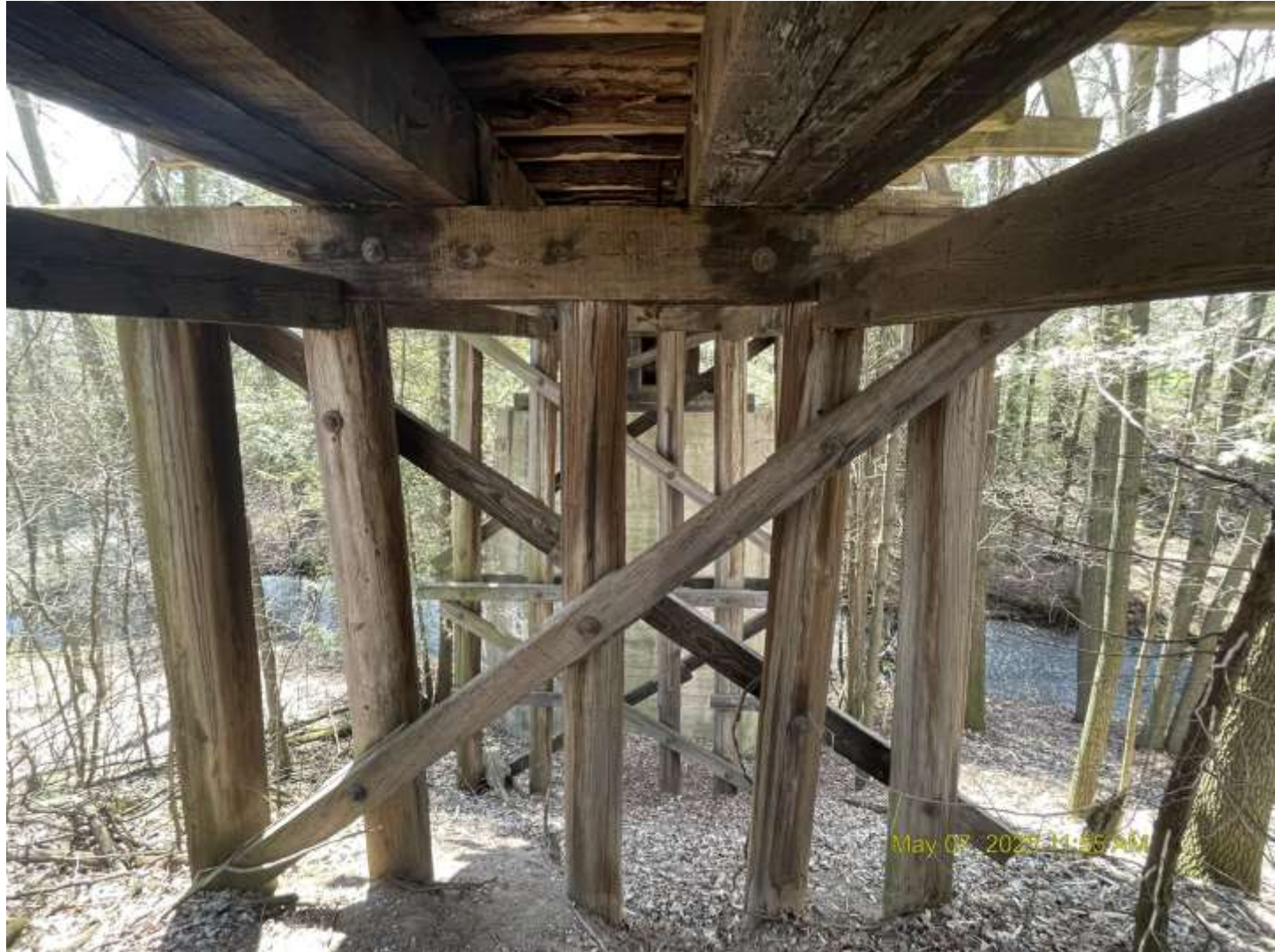
Looking south from N. Abut.
