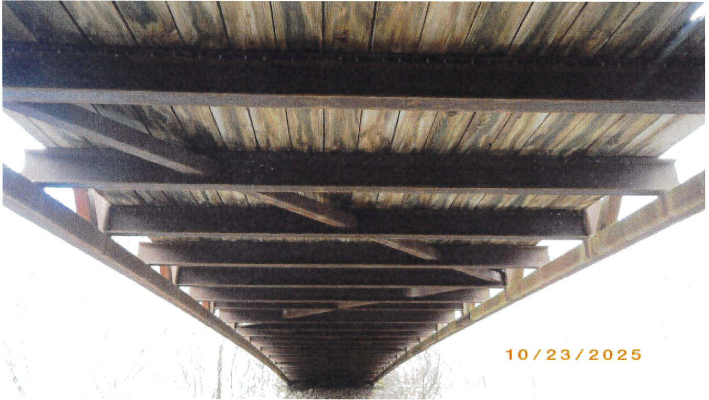
Typical deck / superstructure underside
