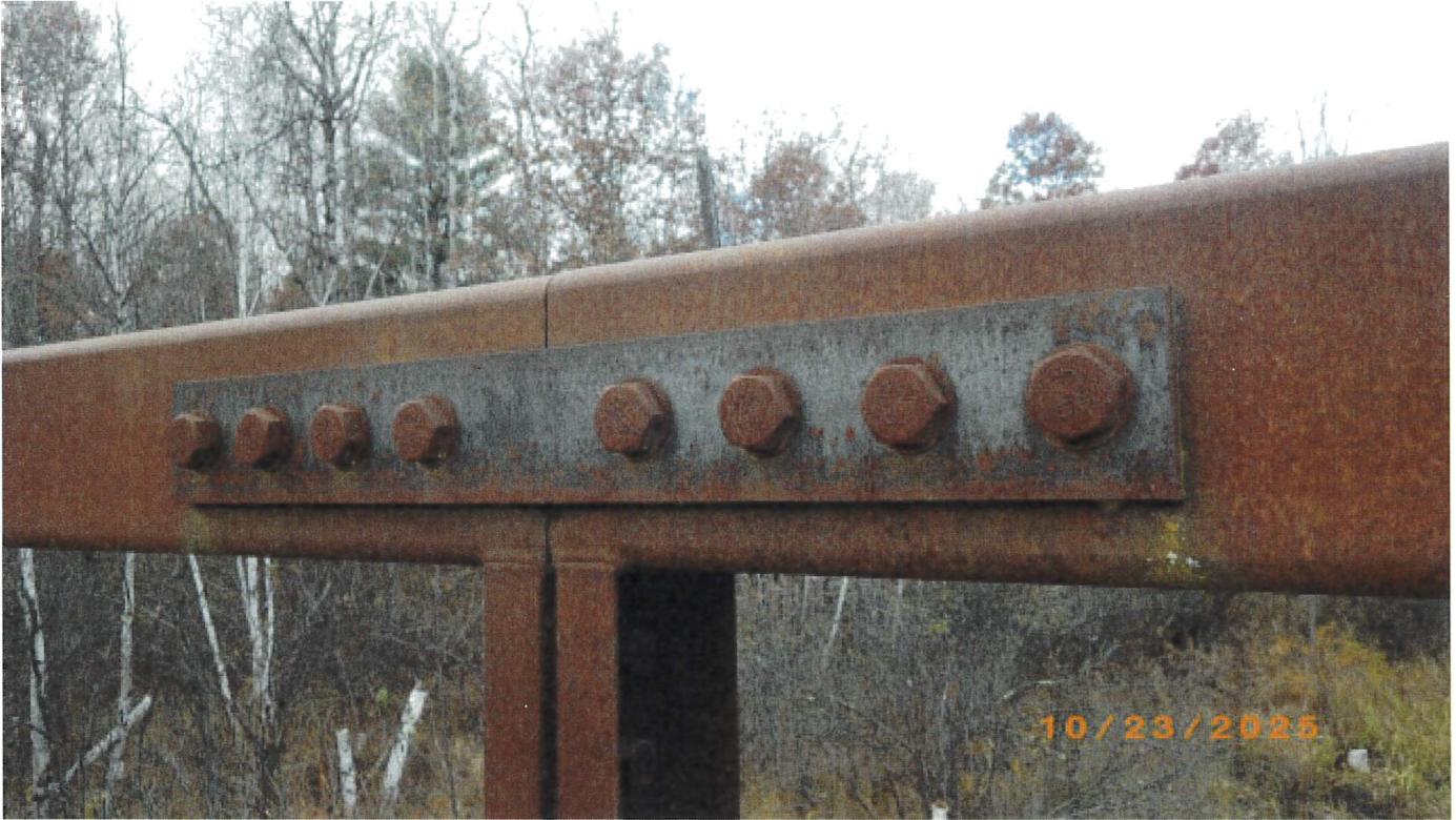
Downstream splice in good condition
