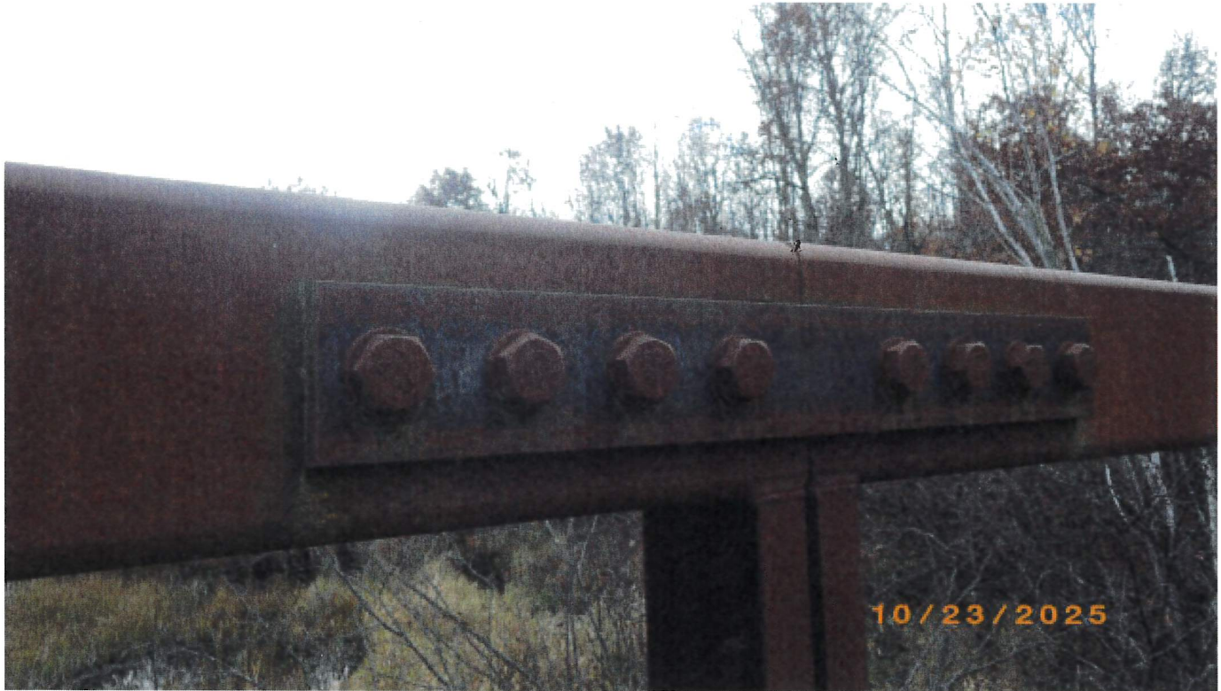
Upstream splice in good condition
