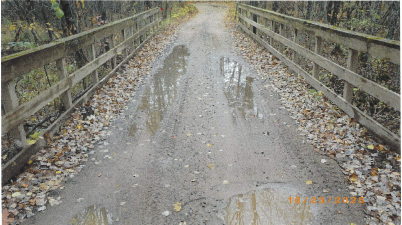
Top of deck
