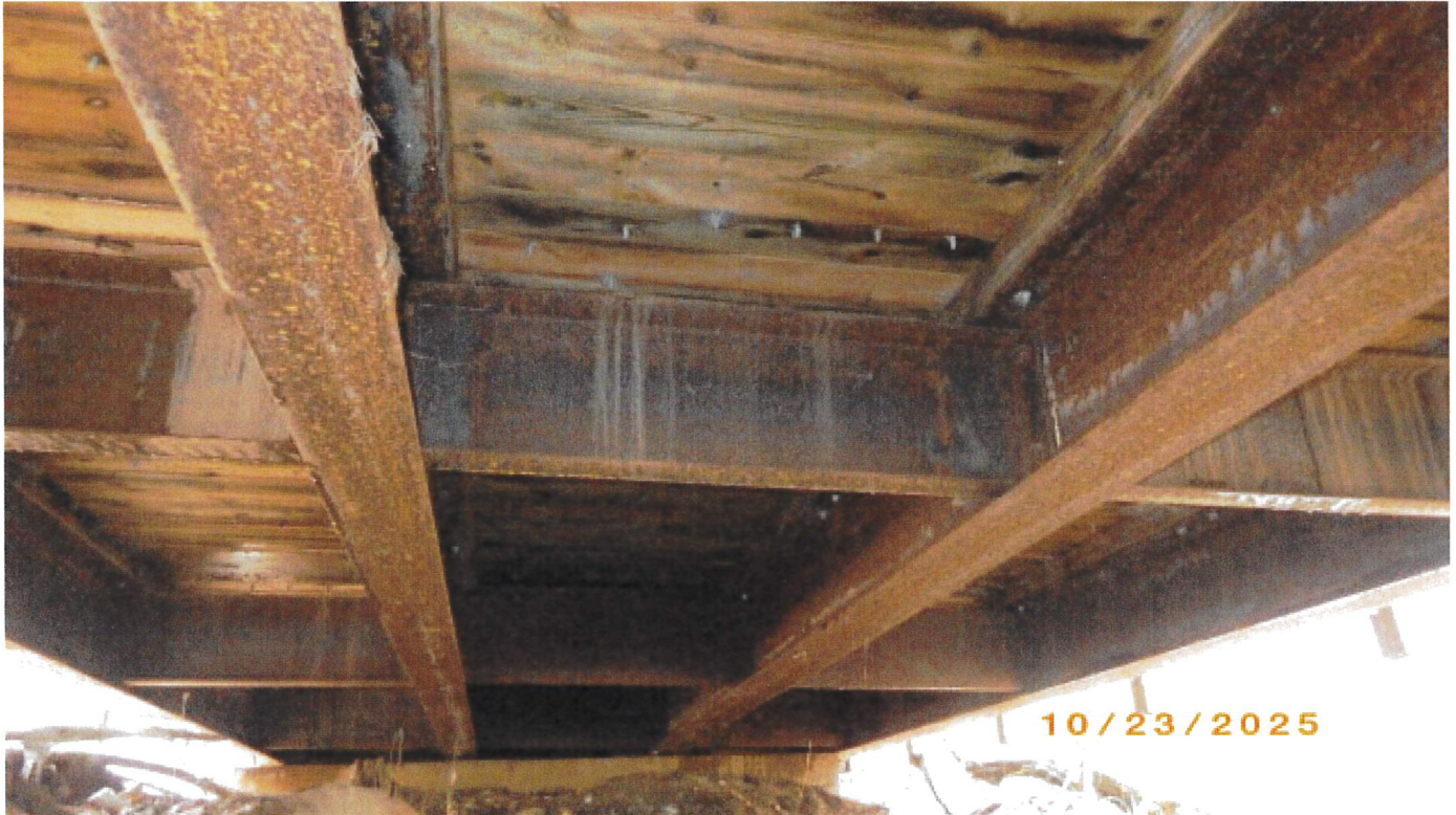
Typical deck / superstructure underside
