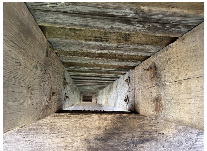
Photo 18 – Underside Near East Pier Looking West.
