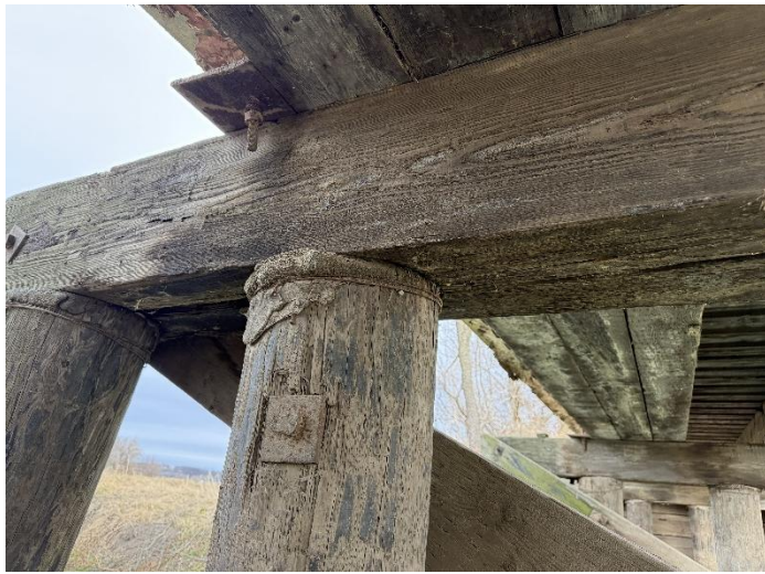
Photo 13 – West Pier Cap-Piles W5-W3.
