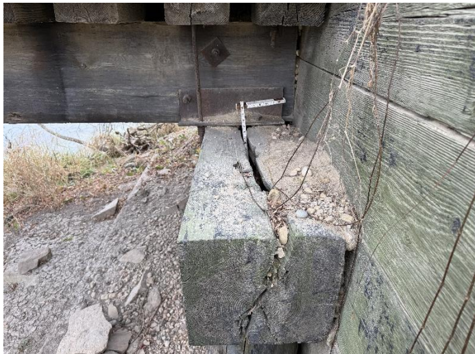
Photo 11 – West Abutment Cap-North End.
