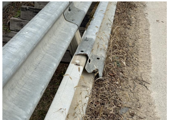
Photo 6 – North Rail Looking East.
