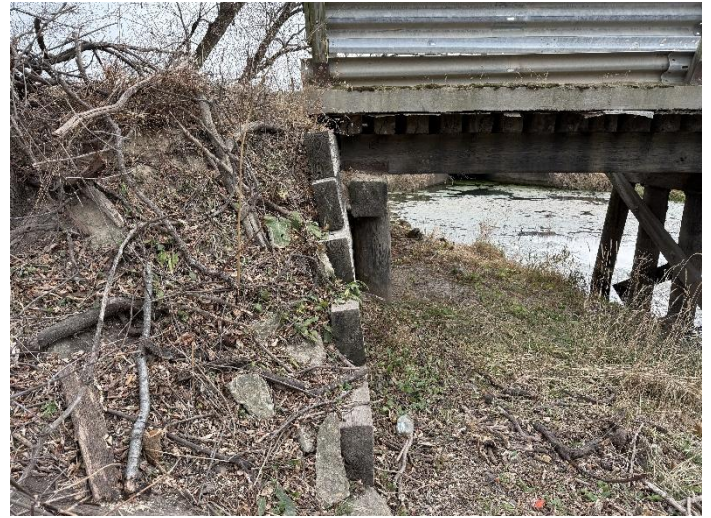
Photo 20 – East Abutment Looking South.
