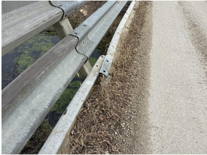
Photo 7 – North Rail Looking East.
