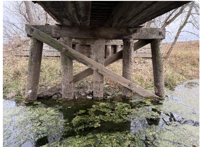
Photo 10 – East Pier Looking East.
