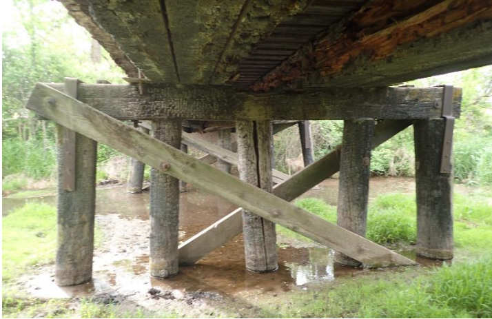
Photo 6 – Pier E2 Looking East
