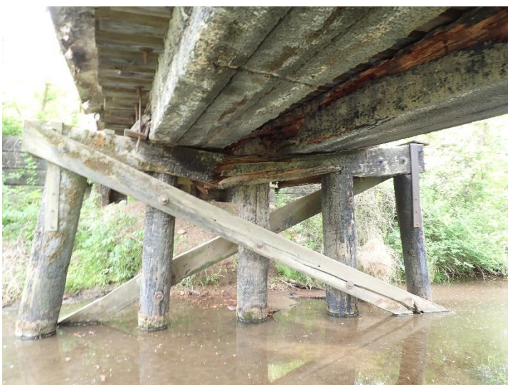
Photo 8 – Pier E1 Looking East
