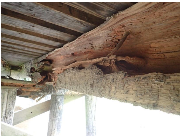
Photo 11 – Span E1 Looking Northwest
