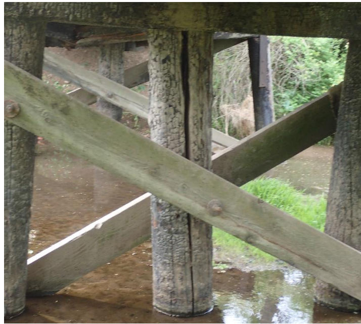
Photo 7 – Pier E2 Looking East
