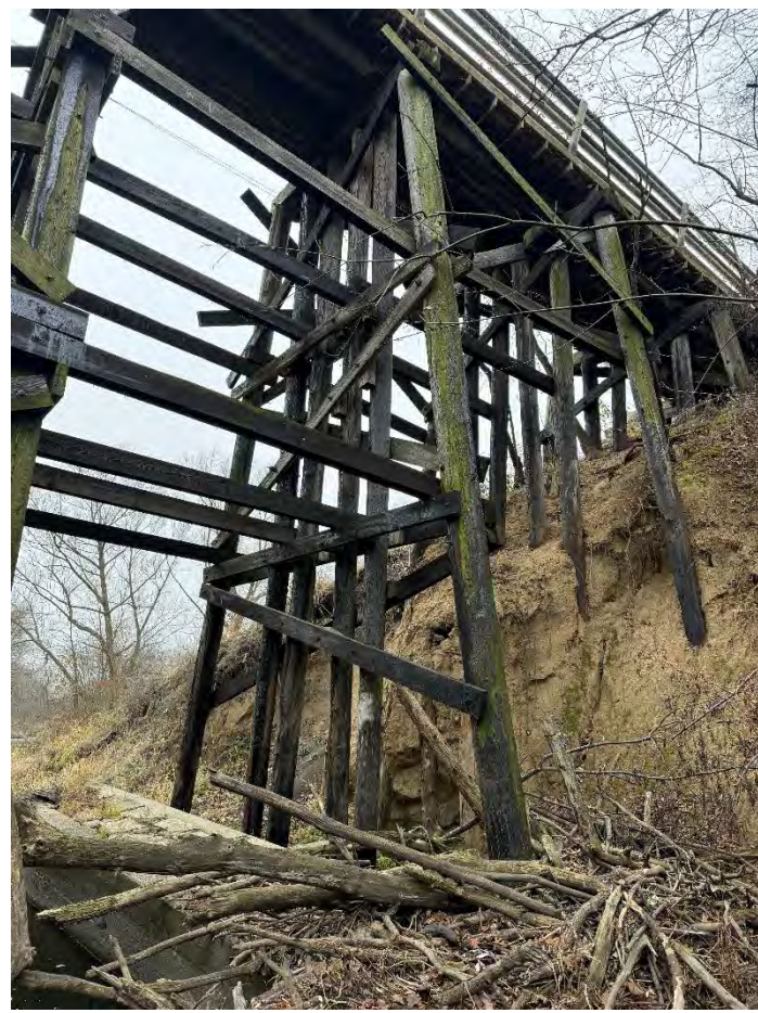
Photo 11 – West Embankment Looking Southwest .
