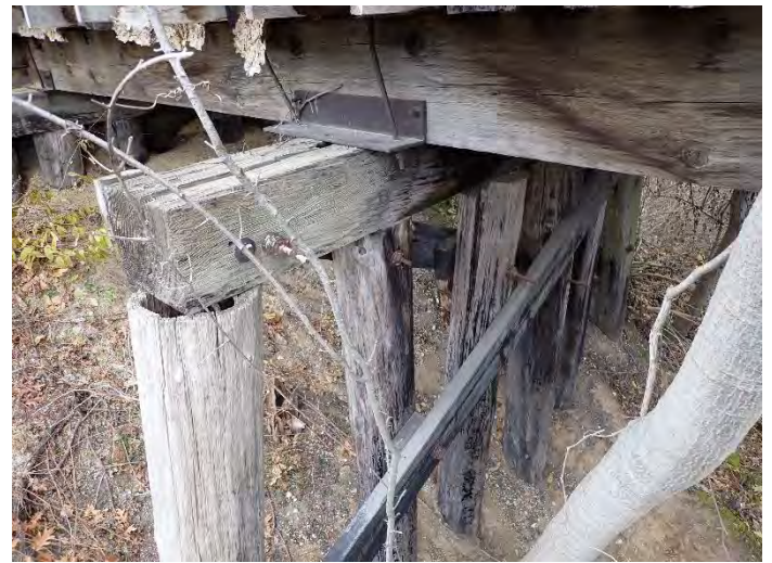
Photo 24 – Pier W1 Looking Northwest.
