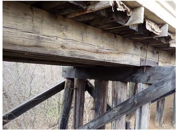
Photo 66 – Span W9 Beams Looking North.
