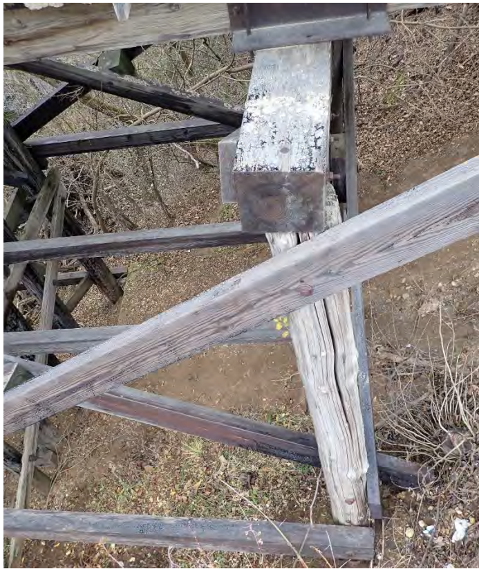
Photo 61 – Pier W9-Pile S1.
