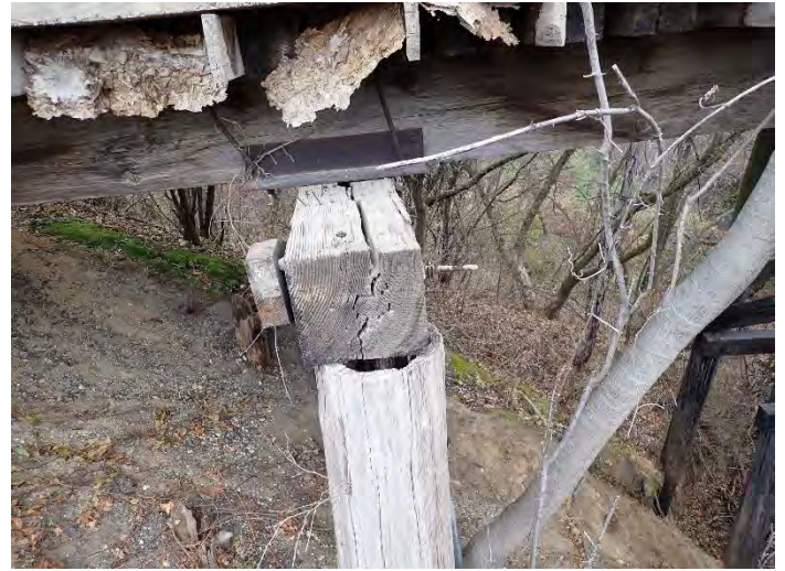
Photo 28 – Pier W1 Looking North.
