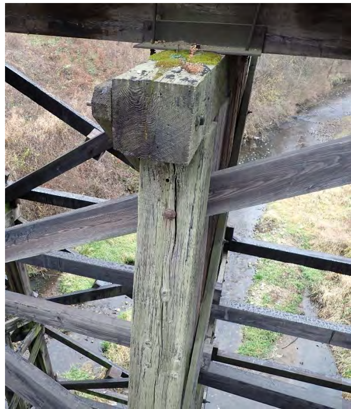
Photo 35 – Pier W4 Looking South.
