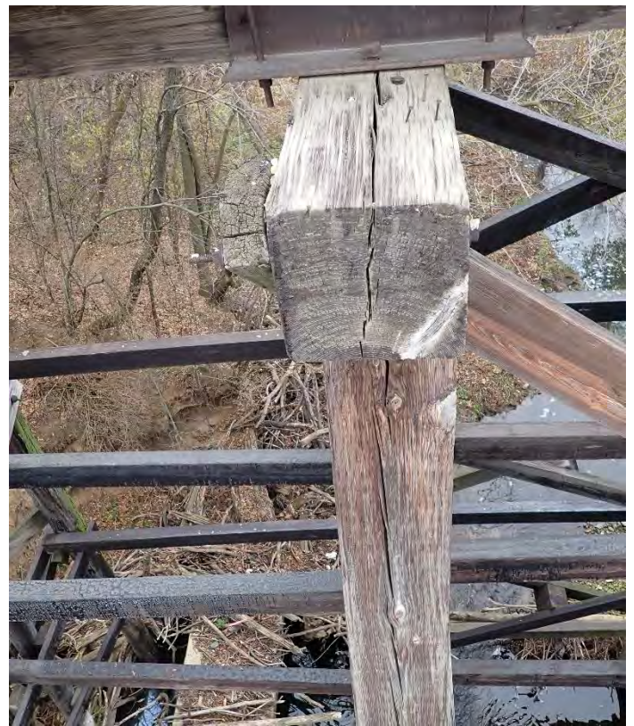
Photo 36 – Pier W4 Looking North.
