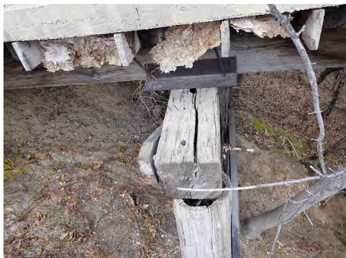
Photo 25 – Pier W1 Cap-South End.
