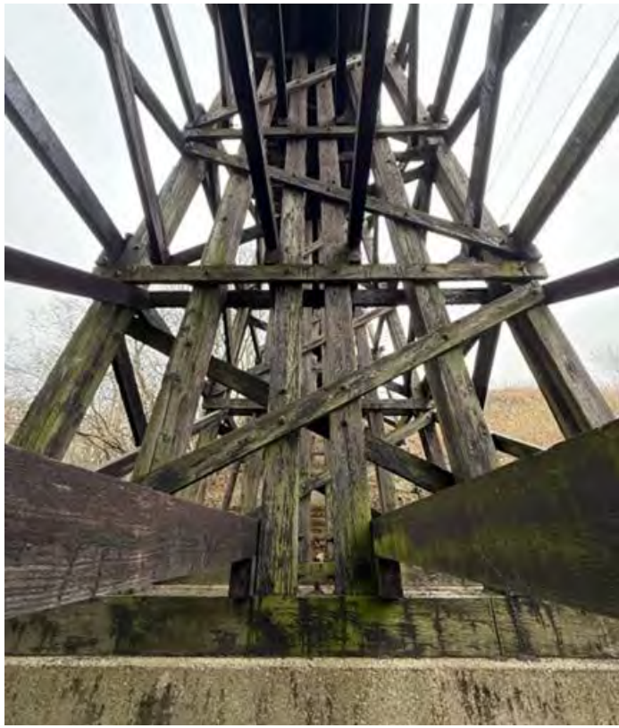
Photo 37 – Pier W5 Looking East.
