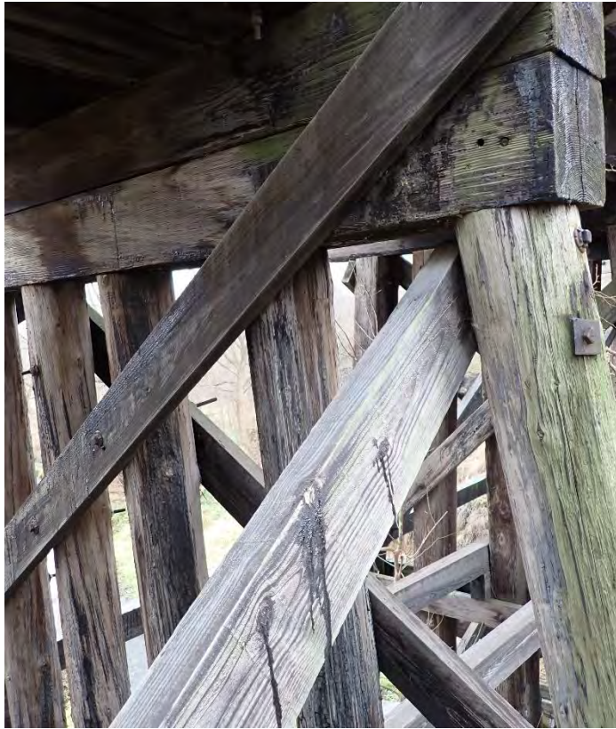
Photo 53 – Pier W7 Looking Southwest.
