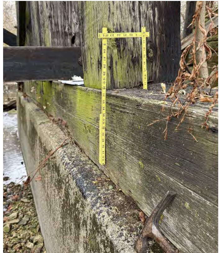
Photo 44 – Pier W6 Bottom Sill-Pile S2.
