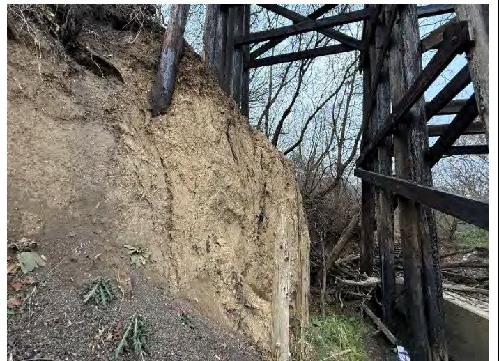
Photo 14 – West Embankment Looking North.
