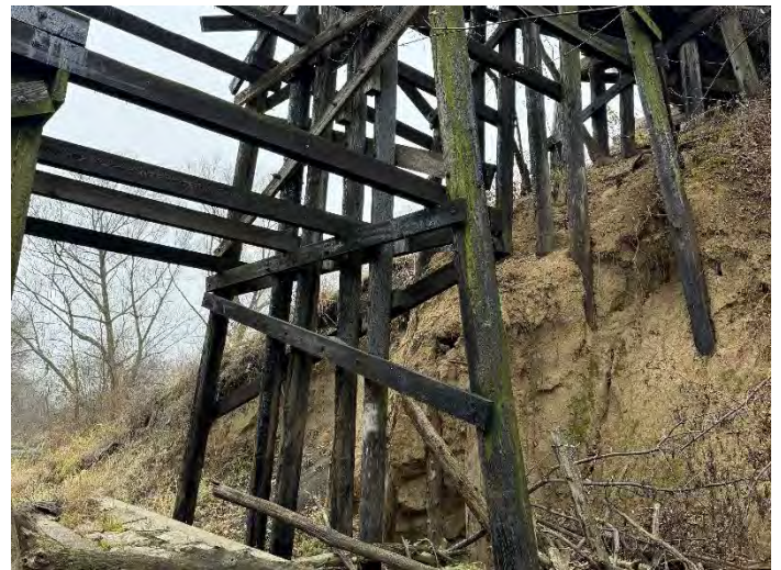
Photo 30 – Pier 2 W3-W2 Looking Southwest.
