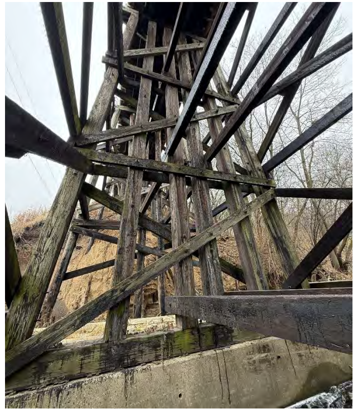
Photo 34 – Pier W4 Looking West.
