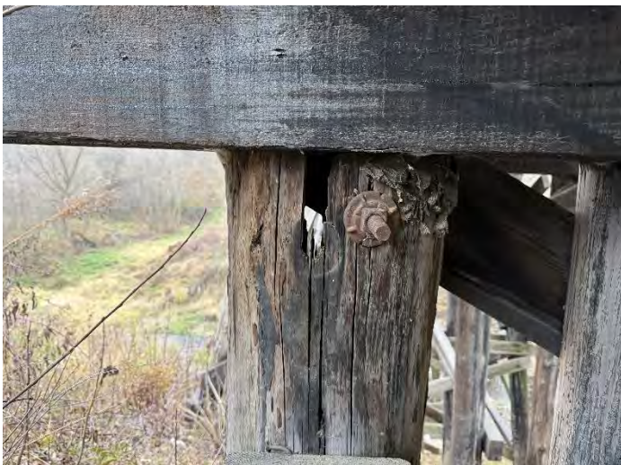
Photo 69 – Pier W10-Pile S2.
