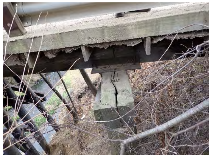
Photo 26 – Pier W1 Cap-North End.
