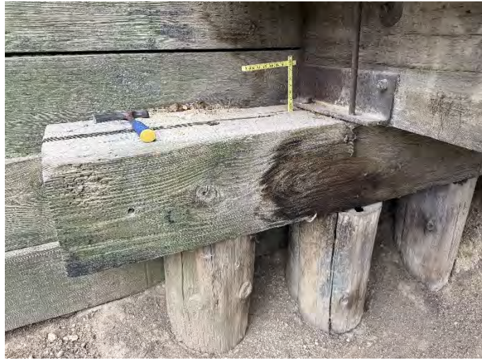
Photo 71 – East Abutment-South End.
