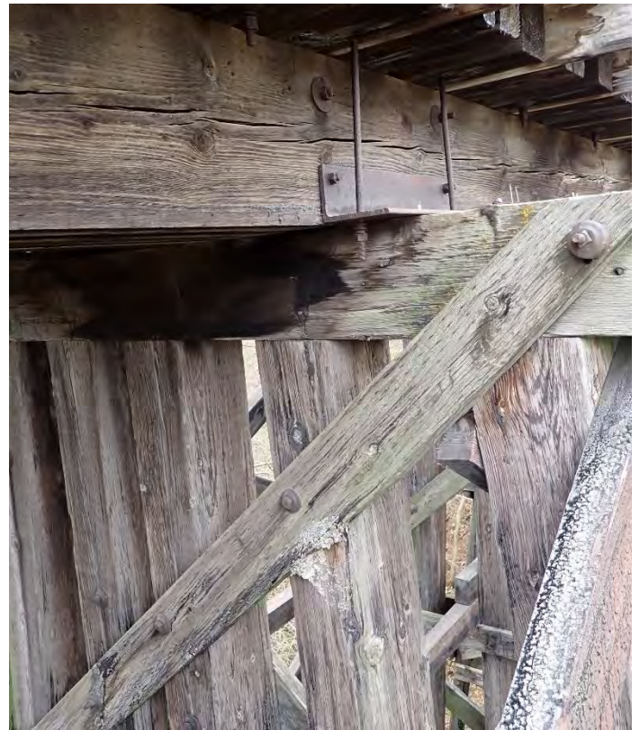
Photo 40 – Beams Over Pier W5 Looking East.
