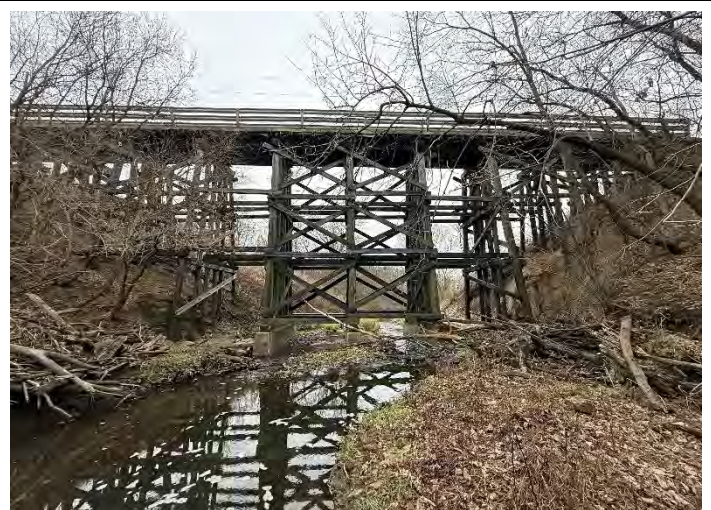
Photo 6 – Side View Looking South.
