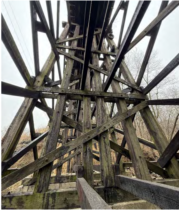
Photo 41 – Pier W5 Looking West.
