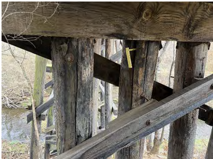
Photo 29 – Pier W1-Pile S5-S3.
