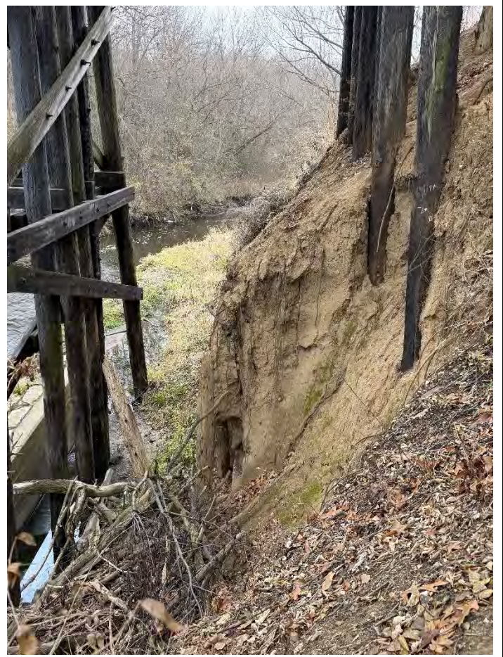
Photo 12 – East Embankment Looking South.
