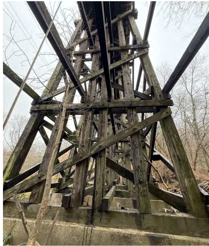
Photo 45 – Pier W6 Looking West.
