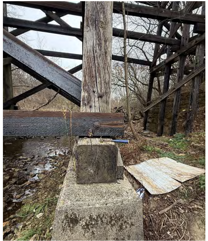
Photo 46 – Pier W6 Looking North.
