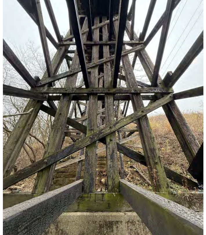
Photo 42 – Pier W6 Looking East.
