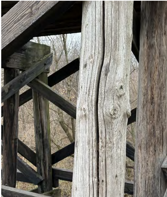
Photo 63 – Pier W9-Pile S1.
