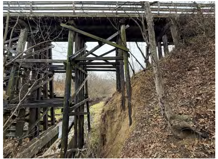
Photo 8 – West Embankment Looking South.
