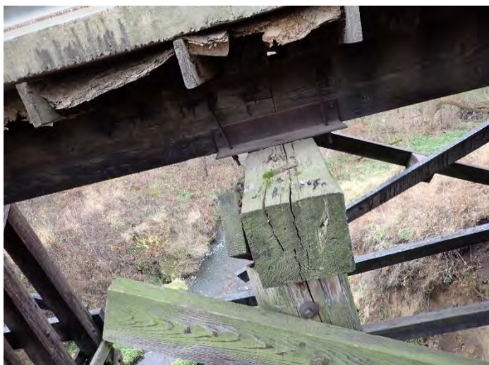
Photo 31 – Pier W3 Looking South.
