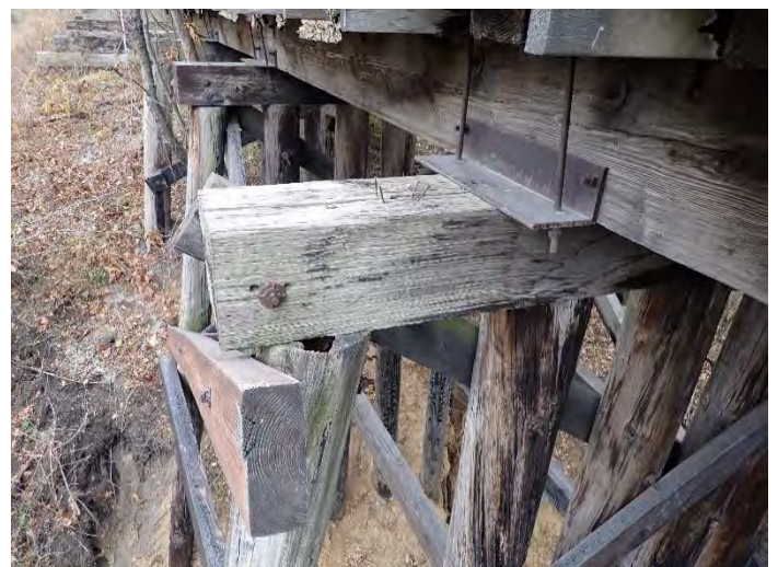
Photo 32 – Pier W3 Looking West.
