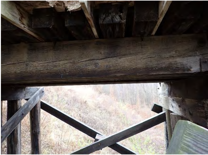
Photo 65 – Span W9 Beams Looking South.
