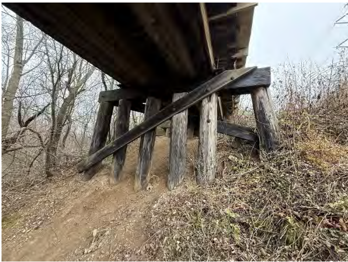
Photo 67 – Pier W10 Looking East.
