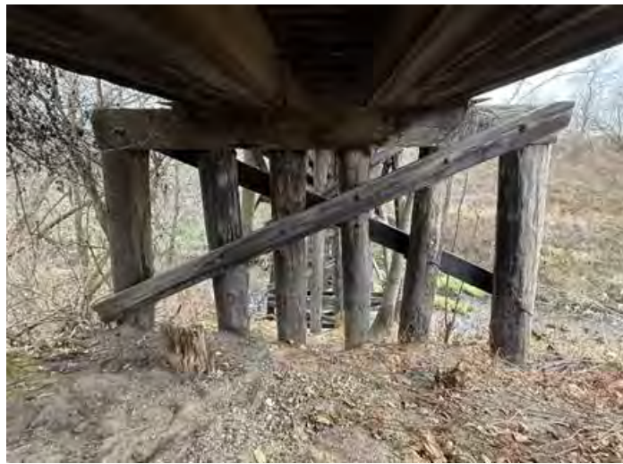
Photo 23 – Pier W1 Looking East.
