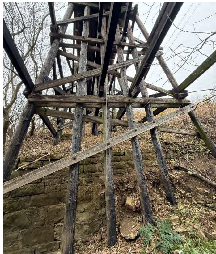
Photo 47 – Pier W7 Looking East.
