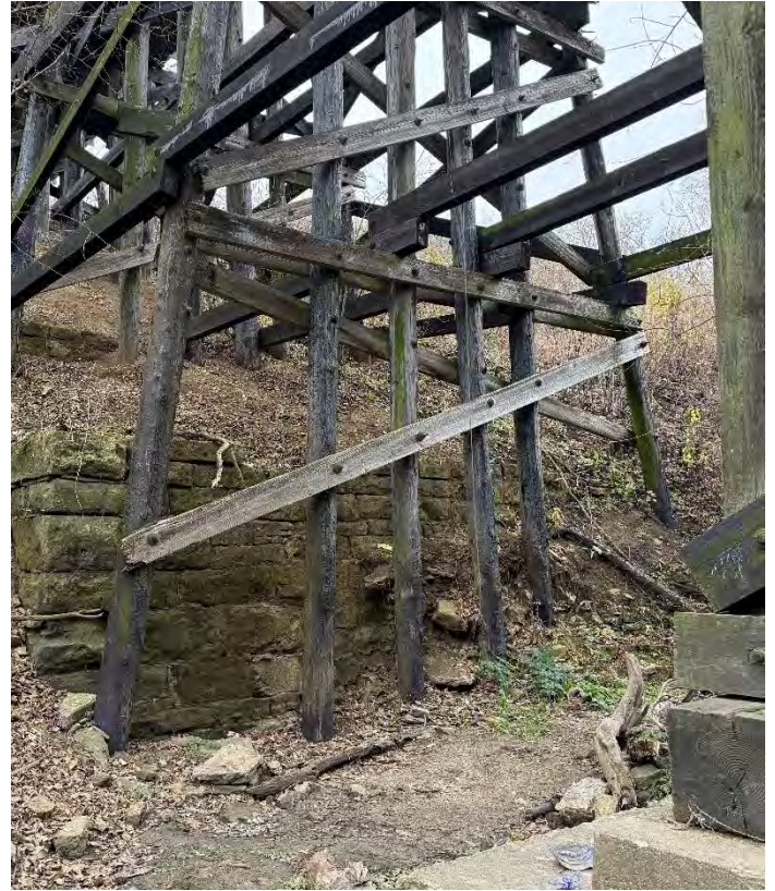
Photo 50 – Pier W7 Looking East.
