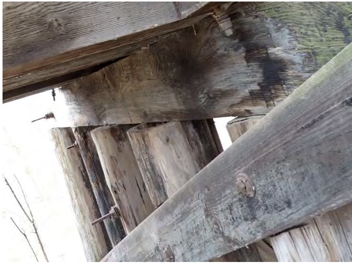
Photo 27 – Pier W1 Looking Southwest.
