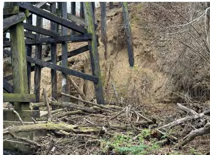
Photo 13 – Northwest Embankment Looking East.
