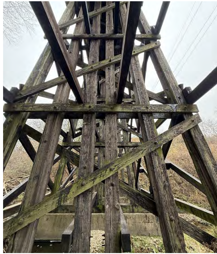
Photo 33 – Pier W4 Looking East.
