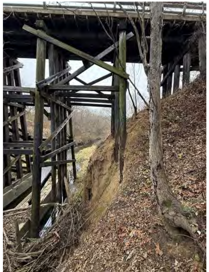
Photo 10 – West Embankment Looking South.
