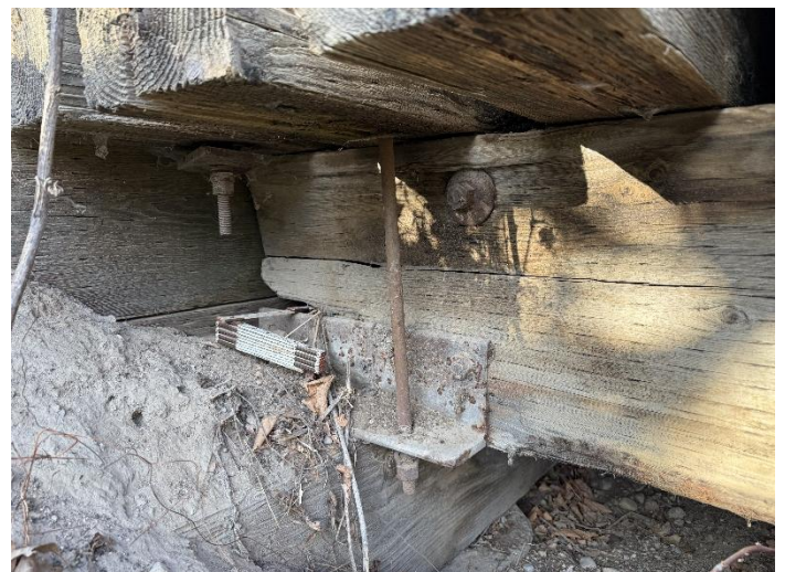
Photo 18 – S. Beam -S. Face. Over West Abutment .
