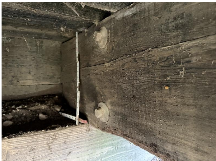
Photo 17 – N. Beam-S. Face Over West Abutment.
