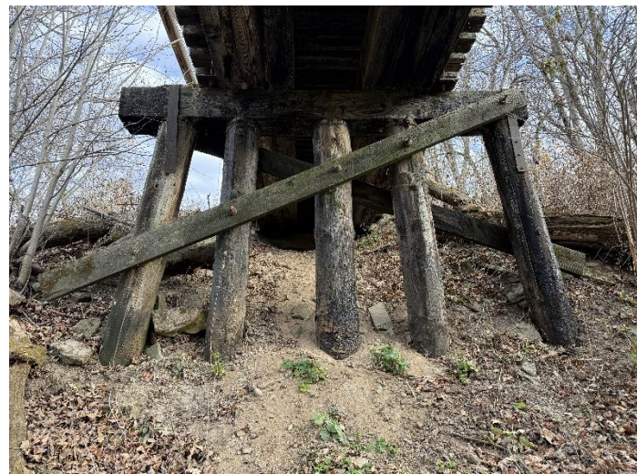
Photo 11 – Pier W4 Looking East.
