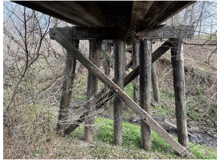
Photo 7 – Pier W2 Looking East.
