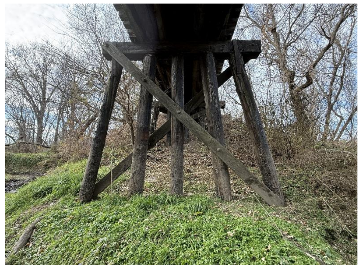
Photo 10 – Pier W2 Looking West.
