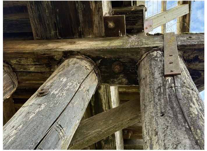
Photo 14 – Pier W3-Piles S3-S5.
