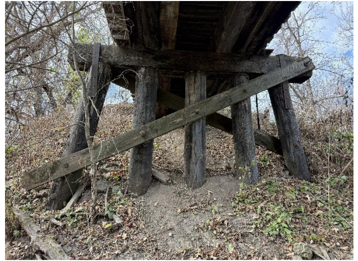
Photo 8 – Pier W1 Looking West.
