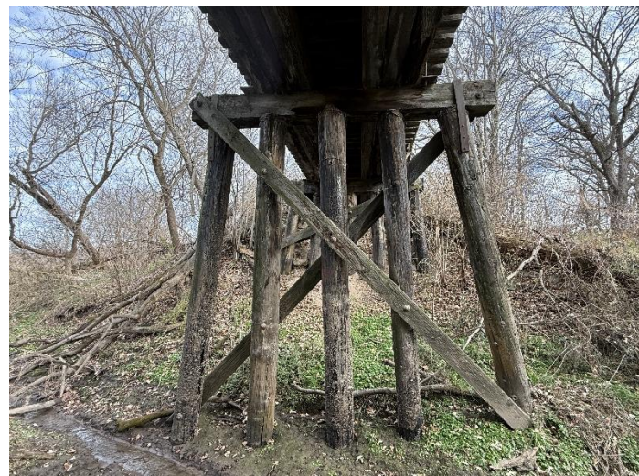
Photo 9 – Pier W3 Looking East.
