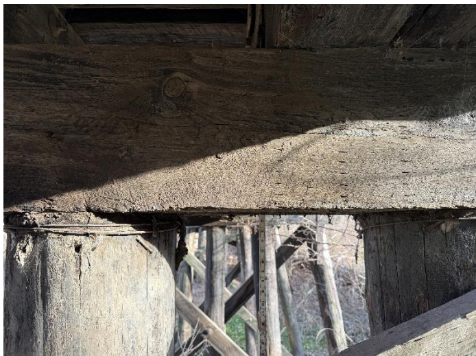
Photo 15 – Pier W1 Cap at Piles S2-S3.
