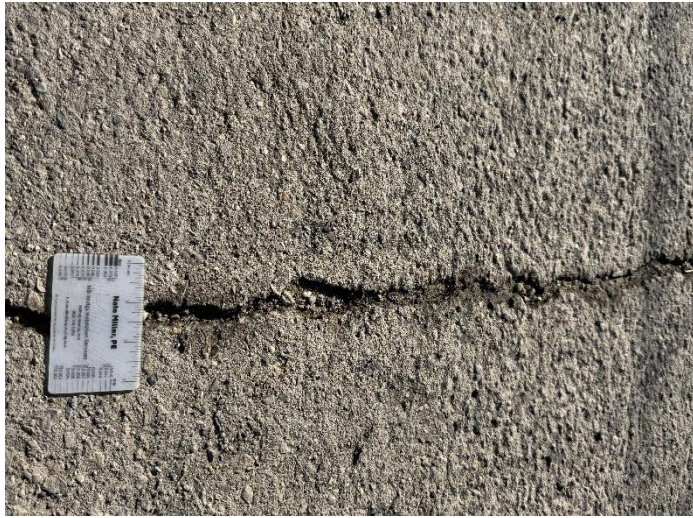
Photo 7 – Deck Near Pier.
