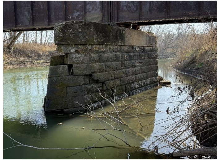
Photo 14 – Pier Looking South.
