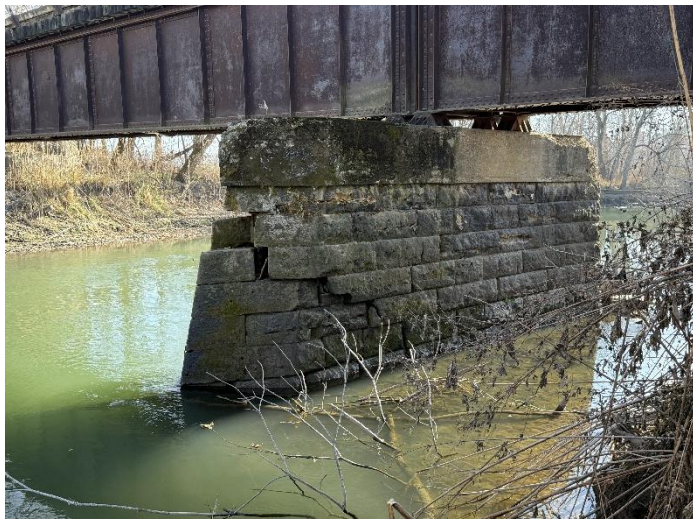
Photo 15 – Pier Looking South.
