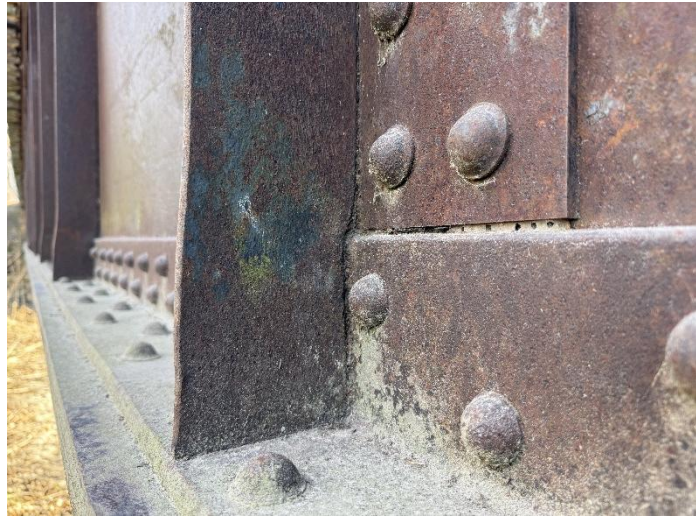
Photo 19 – West Span-North Beam.
