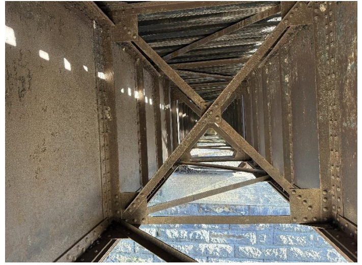
Photo 20 – West Span Looking East.
