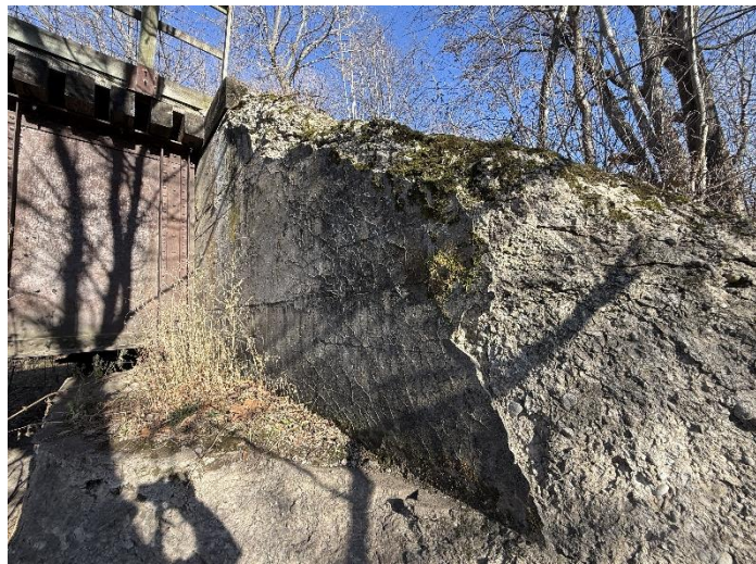
Photo 21 – Southeast Wing Wall Parapet.
