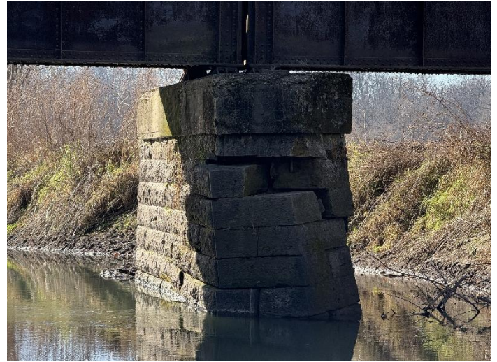
Photo 8 – Pier Looking South.
