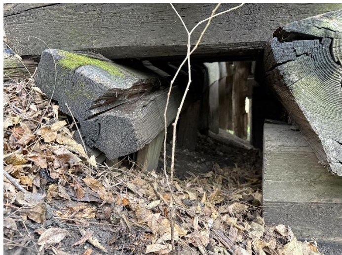
Photo 17 – Pier W4 Looking South.
