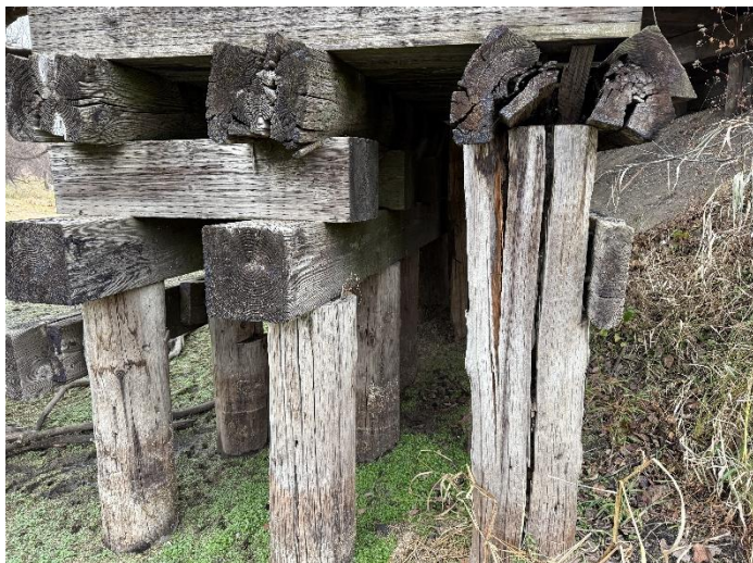
Photo 11 – Pier W4 Looking North.
