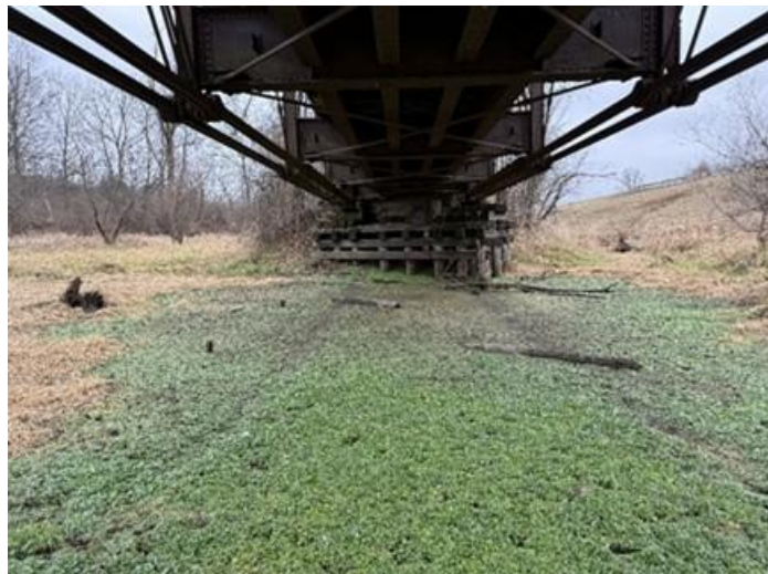
Photo 33 – Pier W4 Looking East.
