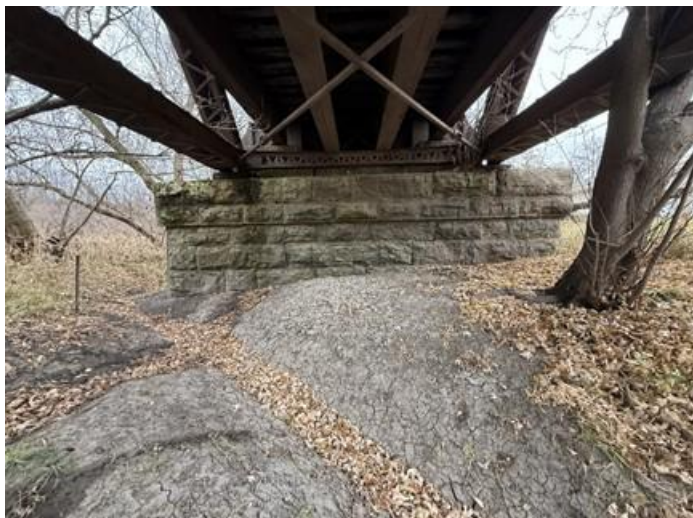
Photo 23 – Pier W2 Looking East.
