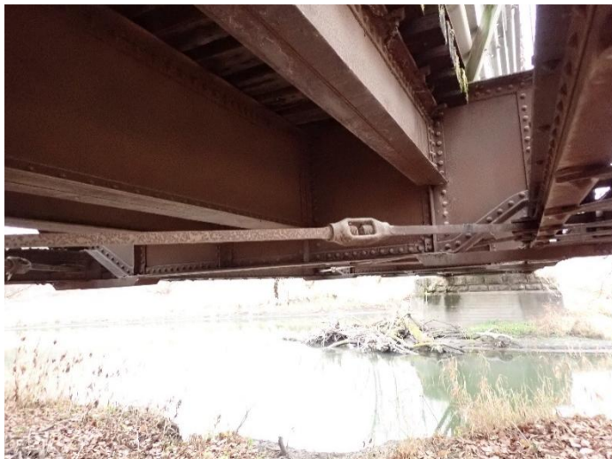
Photo 45 – Span W1-Floor Beam 1 Looking East.
