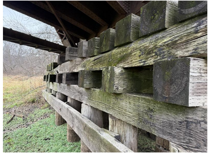
Photo 14 – Pier W4 Looking North-Front Face.
