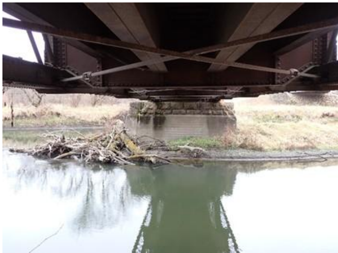
Photo 21 – Pier W1 Looking East.
