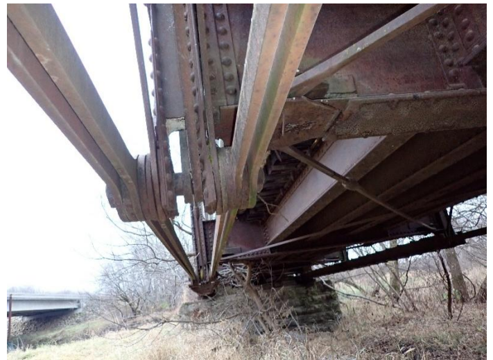
Photo 46 – Span W3-South Truss L3.
