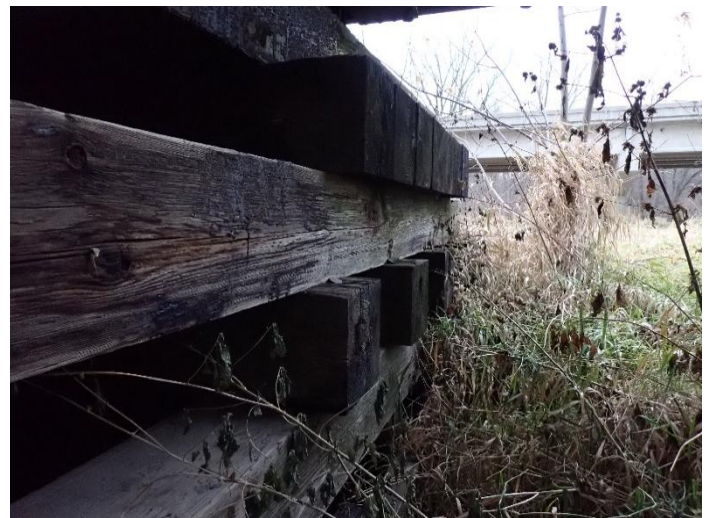
Photo 30 – Pier W3 Looking South.
