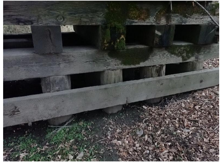
Photo 32 – Pier W3 Looking West.
