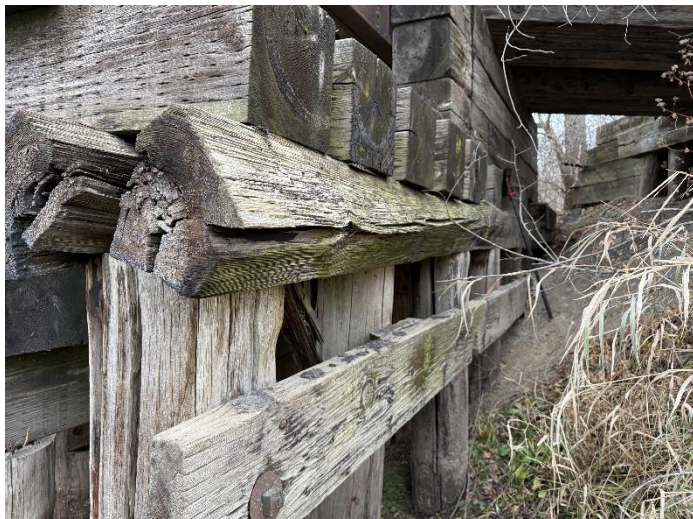
Photo 9 – Pier W4 Looking North.
