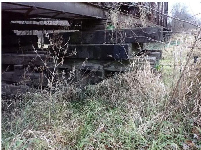
Photo 29 – Pier W3 Looking East.
