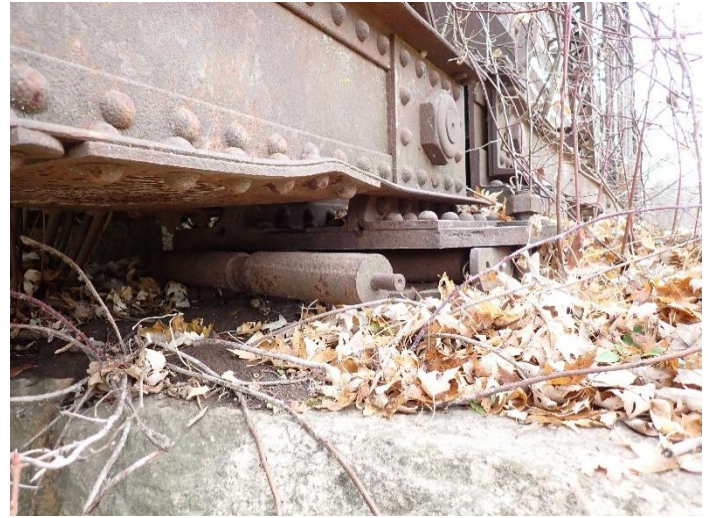
Photo 38 – Span W2-SE. Bearing Over Pier W2.
