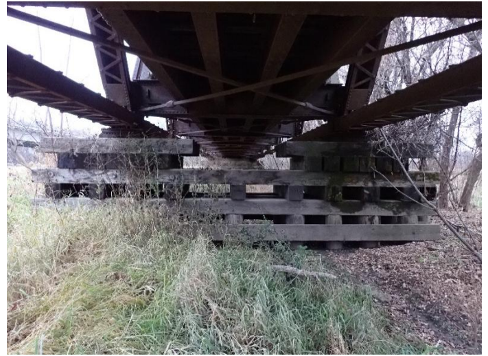
Photo 26 – Pier W3 Looking West.
