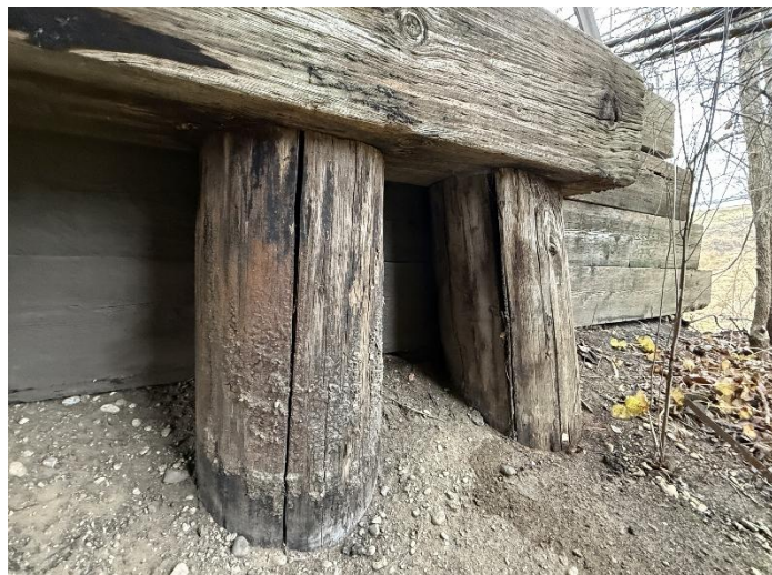
Photo 35 – East Abutment-Piles S2-S1.
