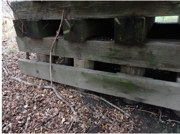
Photo 31 – Pier W3 Looking East.
