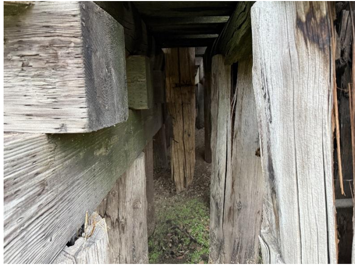
Photo 13 – Pier W4 Looking North-Piles.
