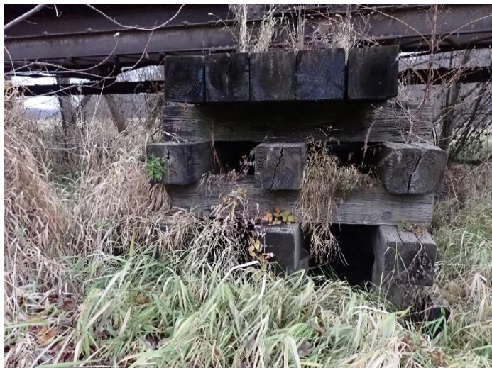
Photo 27 – Pier W3 Looking North.
