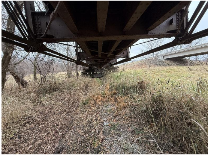
Photo 25 – Pier W3 Looking East.
