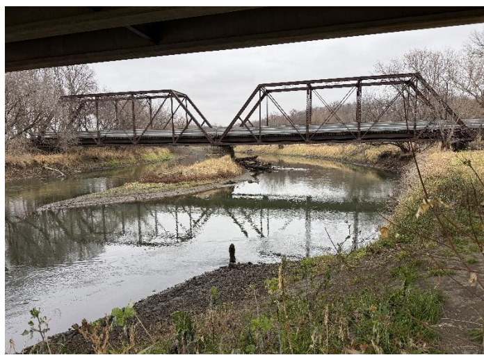
Photo 5 – Side View Looking North-West Spans.
