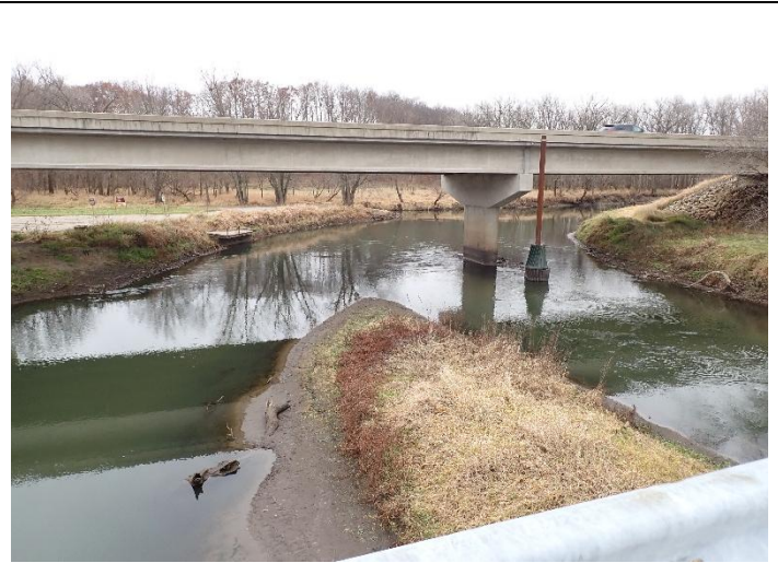
Photo 4 – Downstream Looking South.
