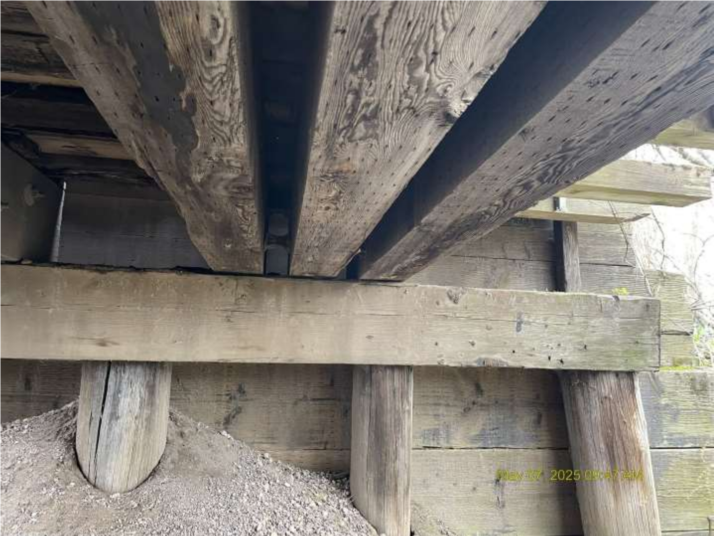
Looking east – south girders
