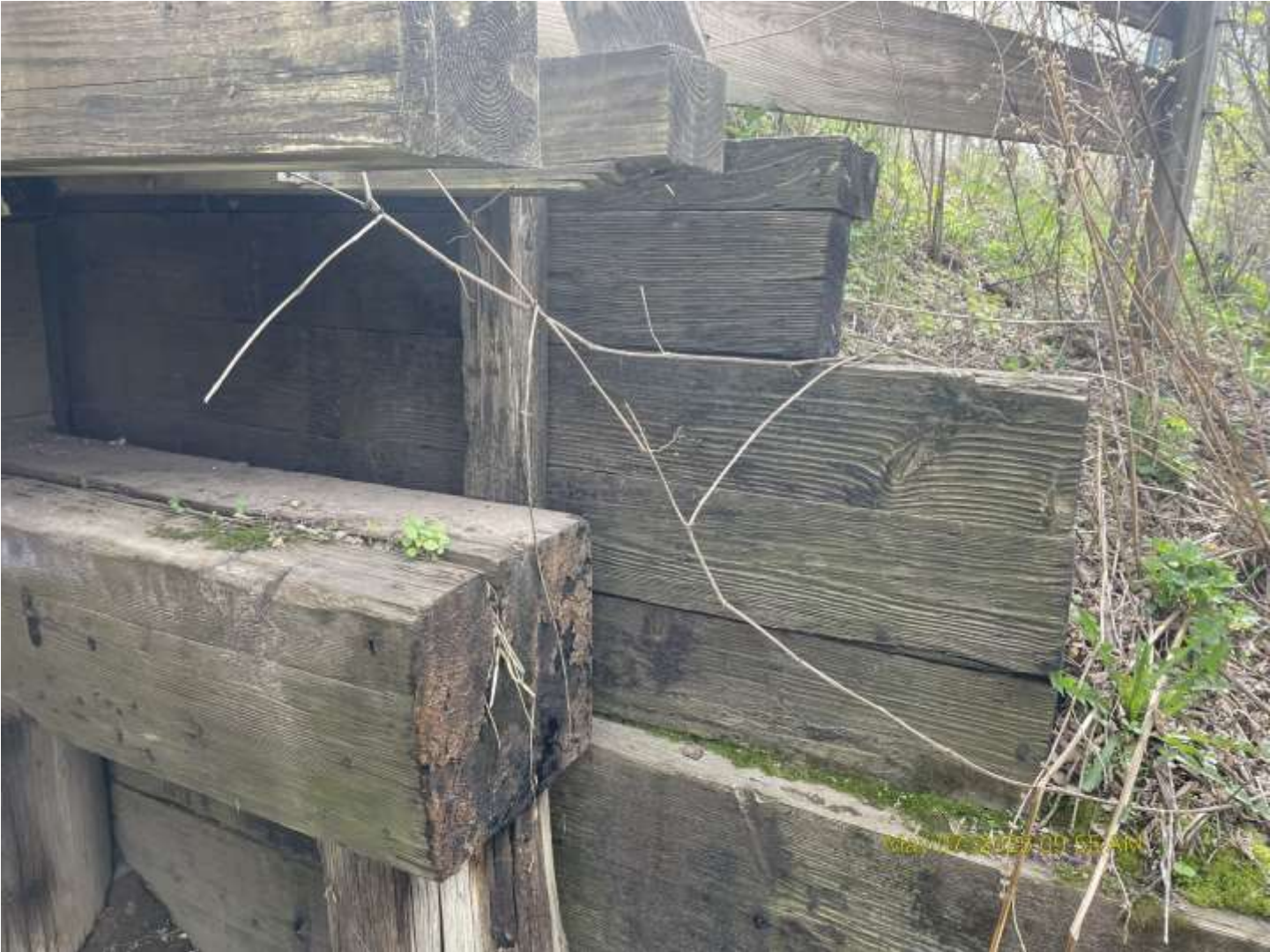
East pier cap south side
