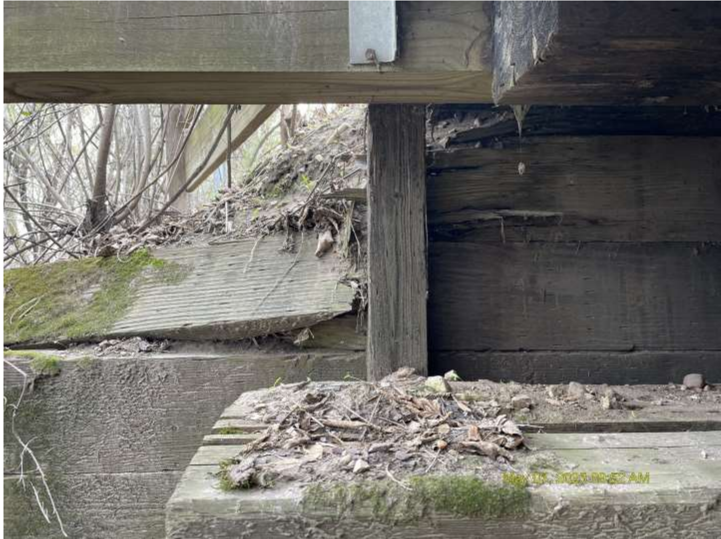
NE corner abutment wall
