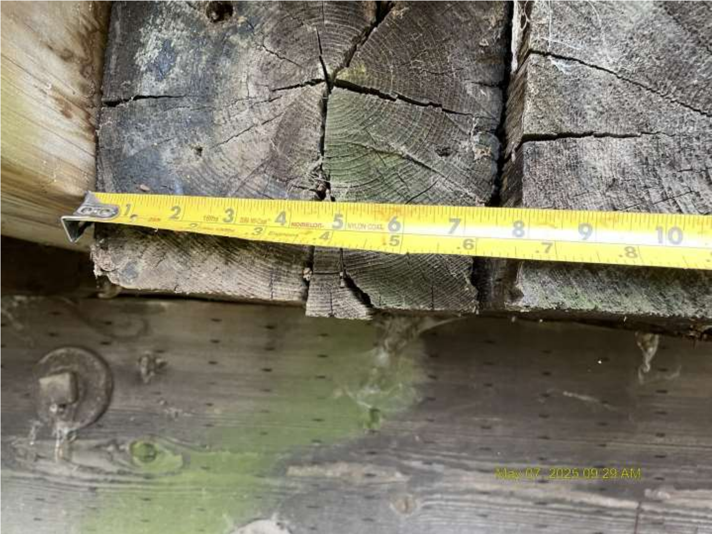
RR ties measurement
