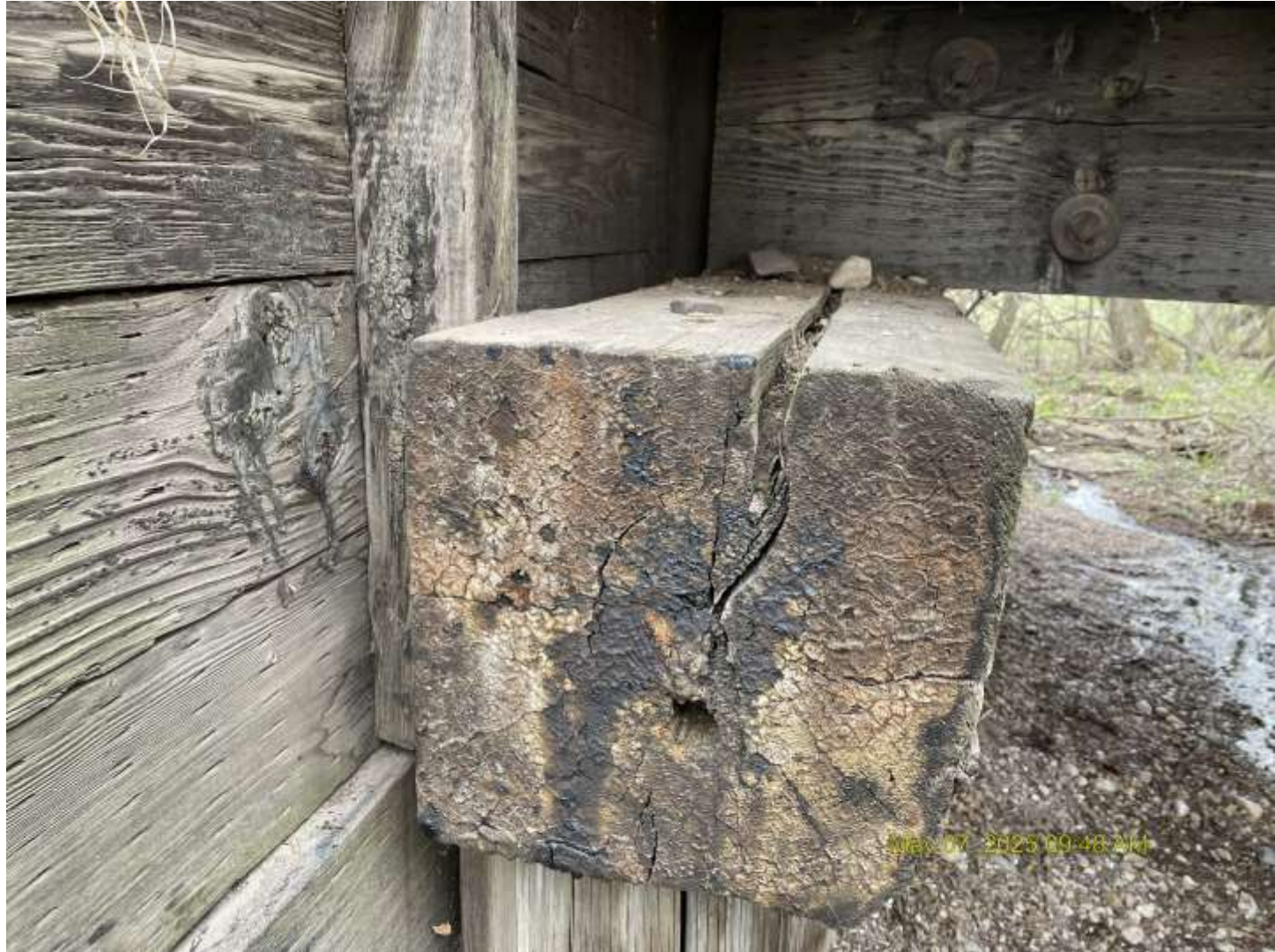
West pier cap
