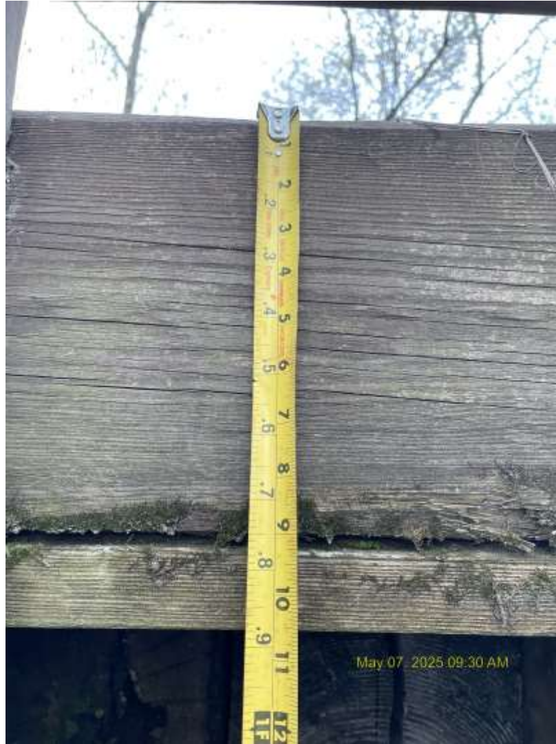
Deck and railing floorboard measurement
