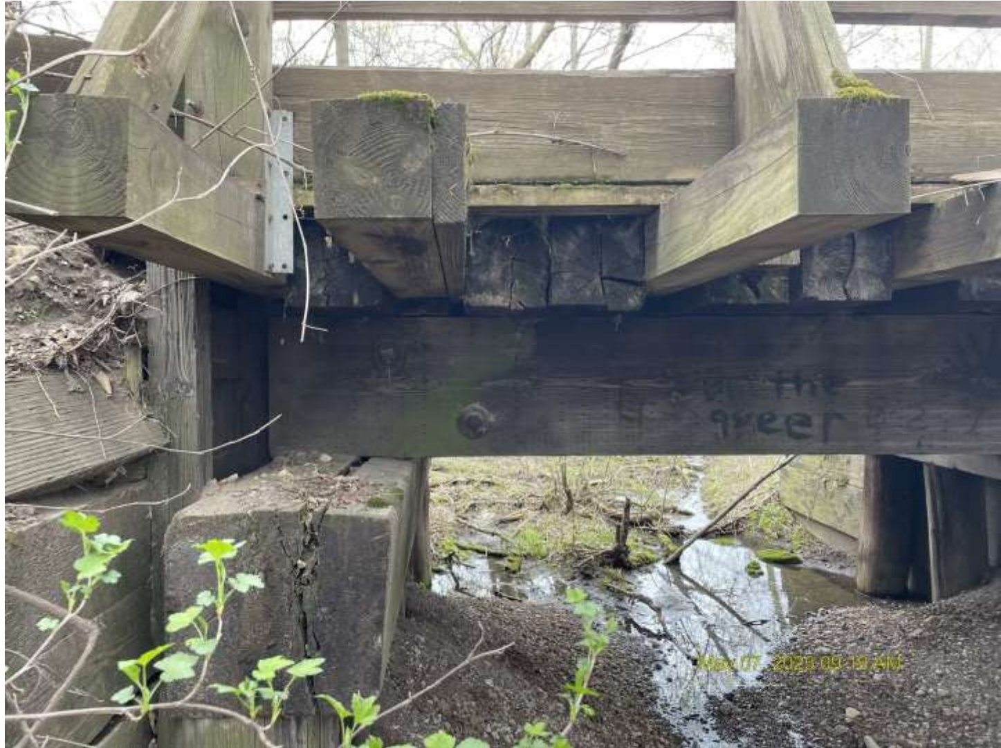
East pier cap
